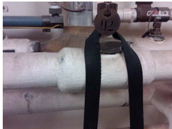
Photo 1.22 – H2O Valve insulation-sampled, no asbestos detected.
