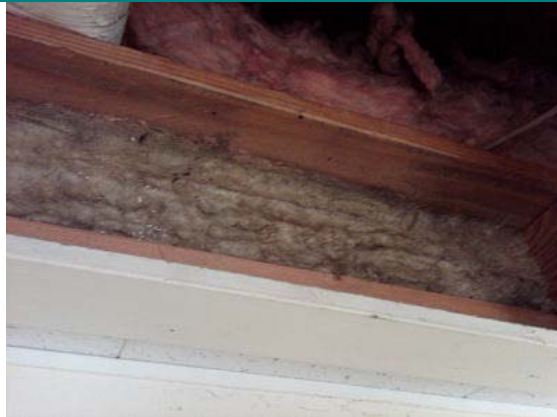
Photo 1.6 Building attic mineral fibre insulation bottom layer
