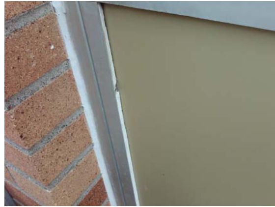
Photo 1.14 – Exterior board cement (no asbestos detected)
