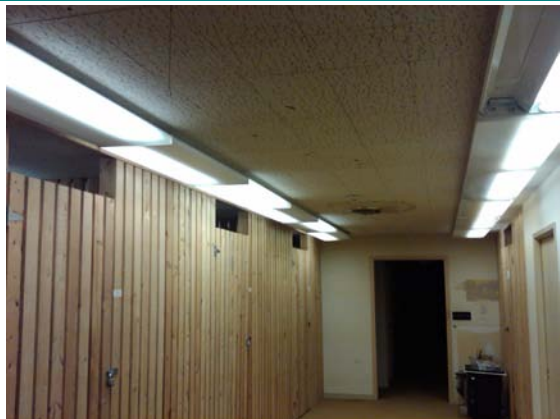
Photo 1.9 - Annex Storage Rooms
