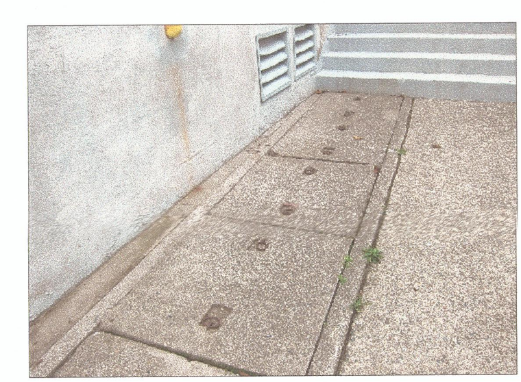
TYPICAL CONCRETE PANELS COVERING ABANDONED STEAM TUNNELS SCALE NTS
