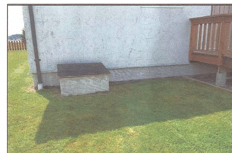
PHOTO OF PFVU-2 BUILDING CRAWLSPACE ACCESS PHOTO #2 SCALE NTS
