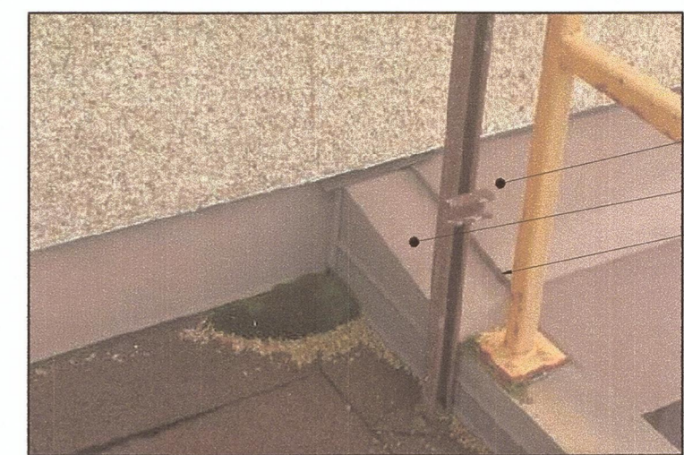
4a EXISTING FLAT TO SLOPED ROOF PHOTO SCALE: N.T.S.
