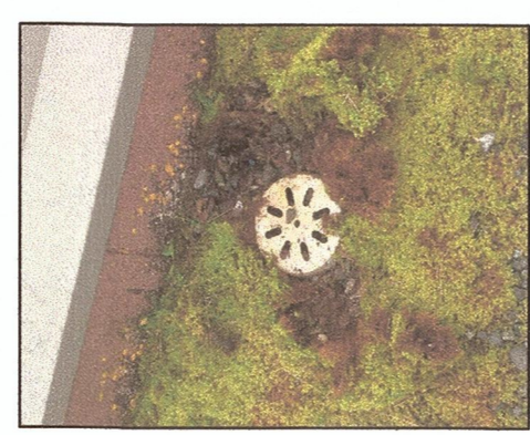
PHOTO 3 TYPICAL ROOF DRAIN
