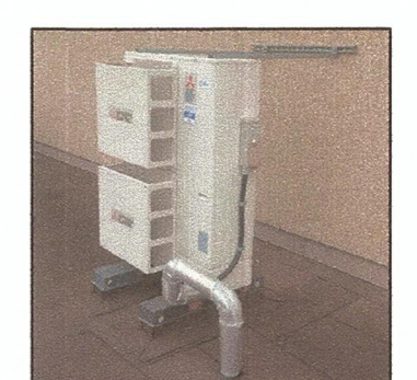
PHOTO_7 MECHANICAL CONDENSING UNIT M2
