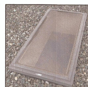
PHOTO 2 TYPICAL FLAT SKYLIGHT
