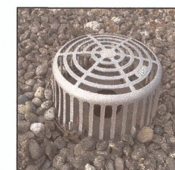
PHOTO 6 TYPICAL ROOF DRAIN
