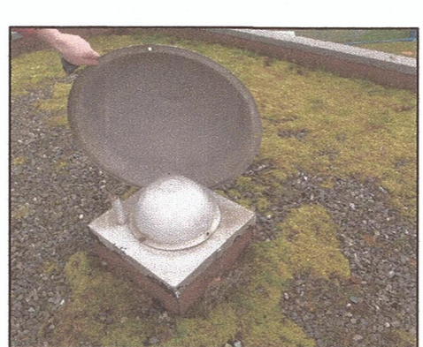
PHOTO 2 DECOMMISSIONED ROOF VENT
