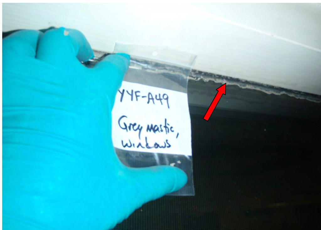
Photograph 44: Asbestos-containing grey window putty on upper window in Room 106A above Room 143. ( Sample 49 ).
