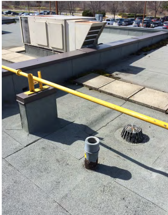
Photograph 27: Typical potential lead-containing roof vent pipe.
