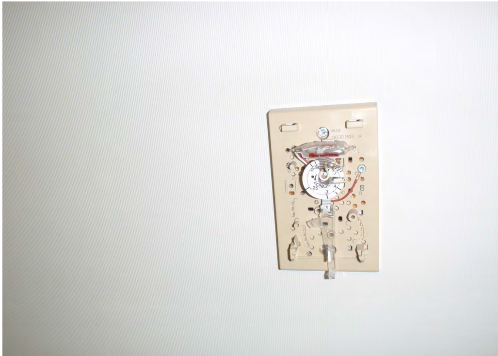
Photograph 25: Typical mercury-containing thermostat (Room 142).
