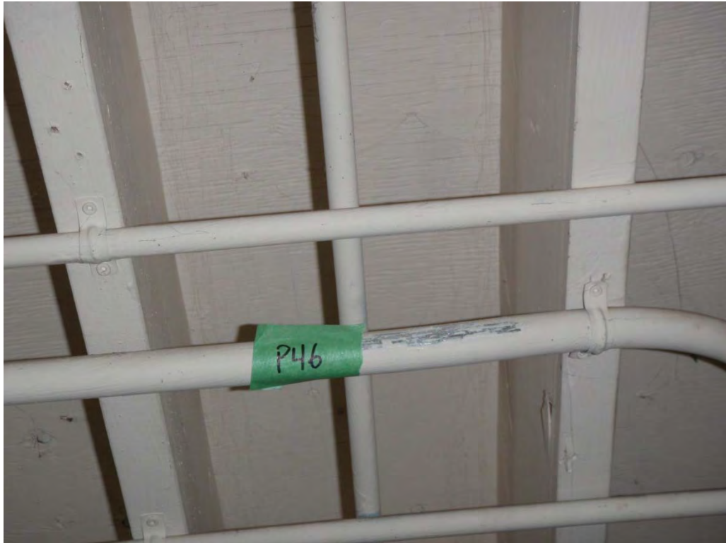
Photograph 87: Lead-based beige paint on steel pipe near ceiling of Room 107 ( Sample P46 ).
