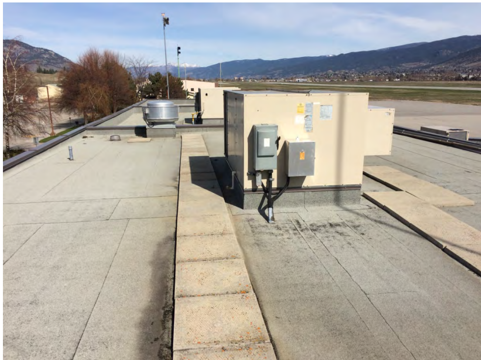
Photograph 26: Typical rooftop air conditioning unit.
