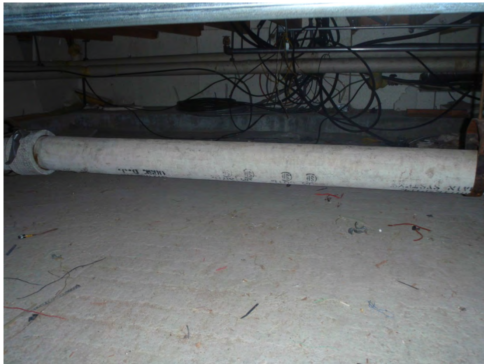
Photograph 17: Room 127 crawlspace with asbestos-containing concrete pipe.
