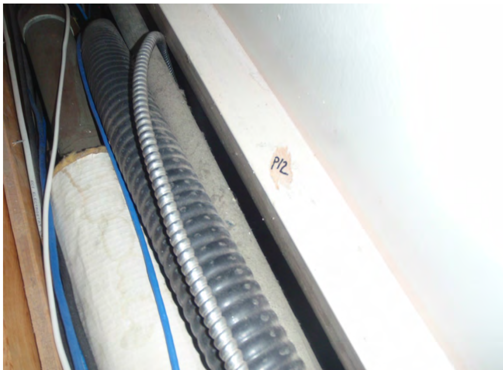
Photograph 66: Lead-based off-white trim paint in Room 106A above Room 143 ( Sample P12 ).
