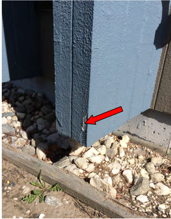
Photograph 47: Asbestos-containing exterior wall texture on west side of building ( Sample A114 and Sample A116 ).
