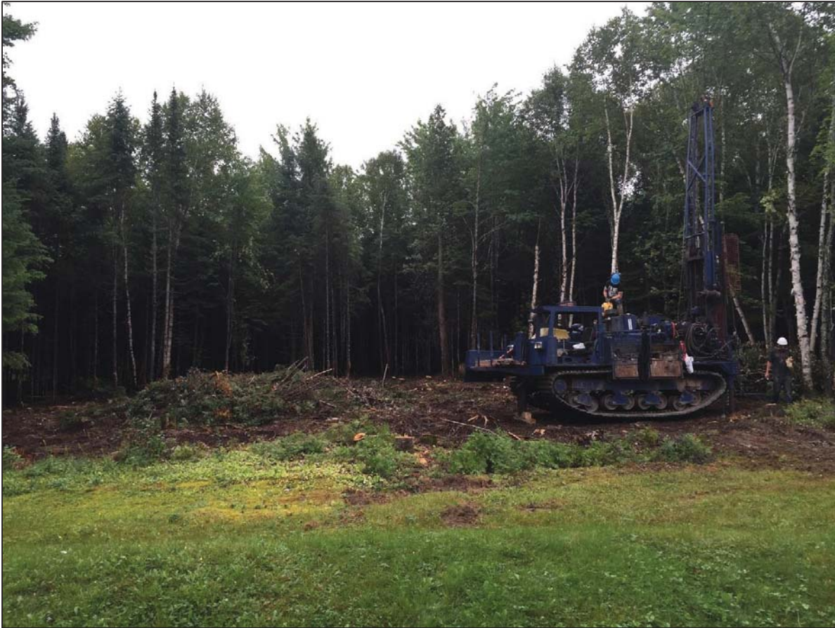
Figure 1 Borehole advancement in clearing on site
