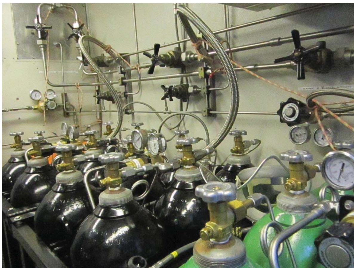
Figure 1: CDS RCC – Air banks
