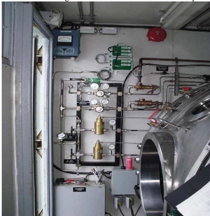
Figure 5: Interior view of bulkhead between the compressor and recompression chamber sections of the Existing CDS – RCC. View from the recompression chamber section side.
