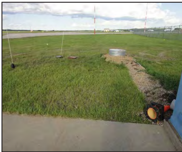
Photo 05 - UST manhole and fuel line trench leading to the fuel dispensing stand.
