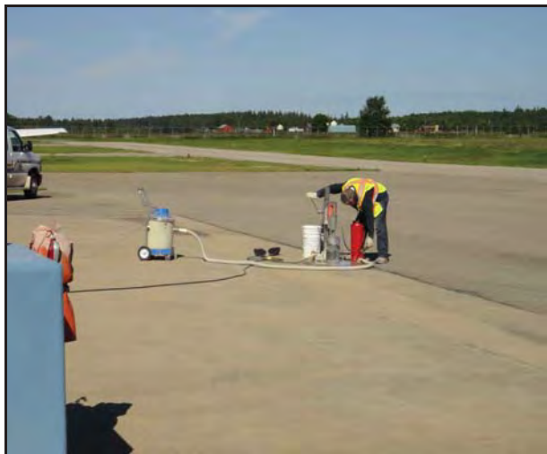
Photo 17 - Concrete coring at test hole PA-09 located north of the RCMP Hangar.
