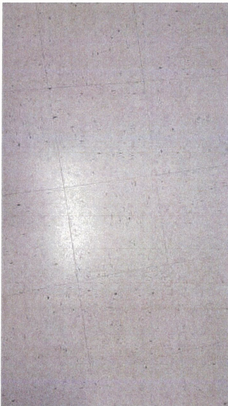
Floor tiles in Rooms 240 and 245 – Samples B14A and B14B.
