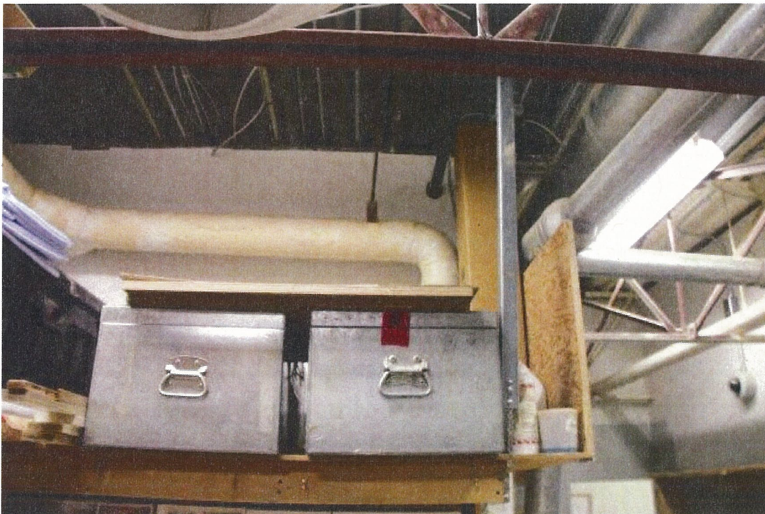
Northeast corner (Room 248) – pipe insulation – elbow.
