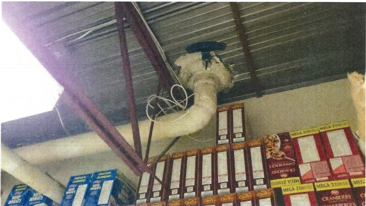
Fibreglass insulation around roof drain.
