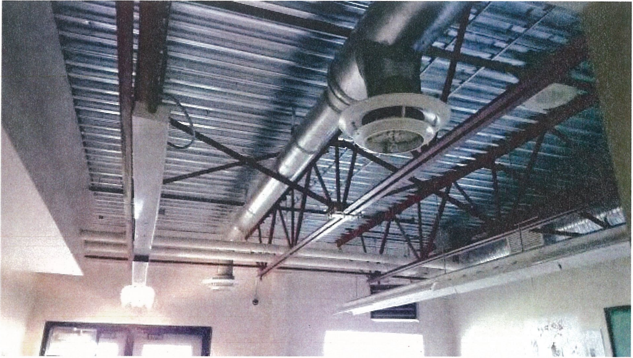
Grey duct mastic in ceiling ducts (Room 237).
