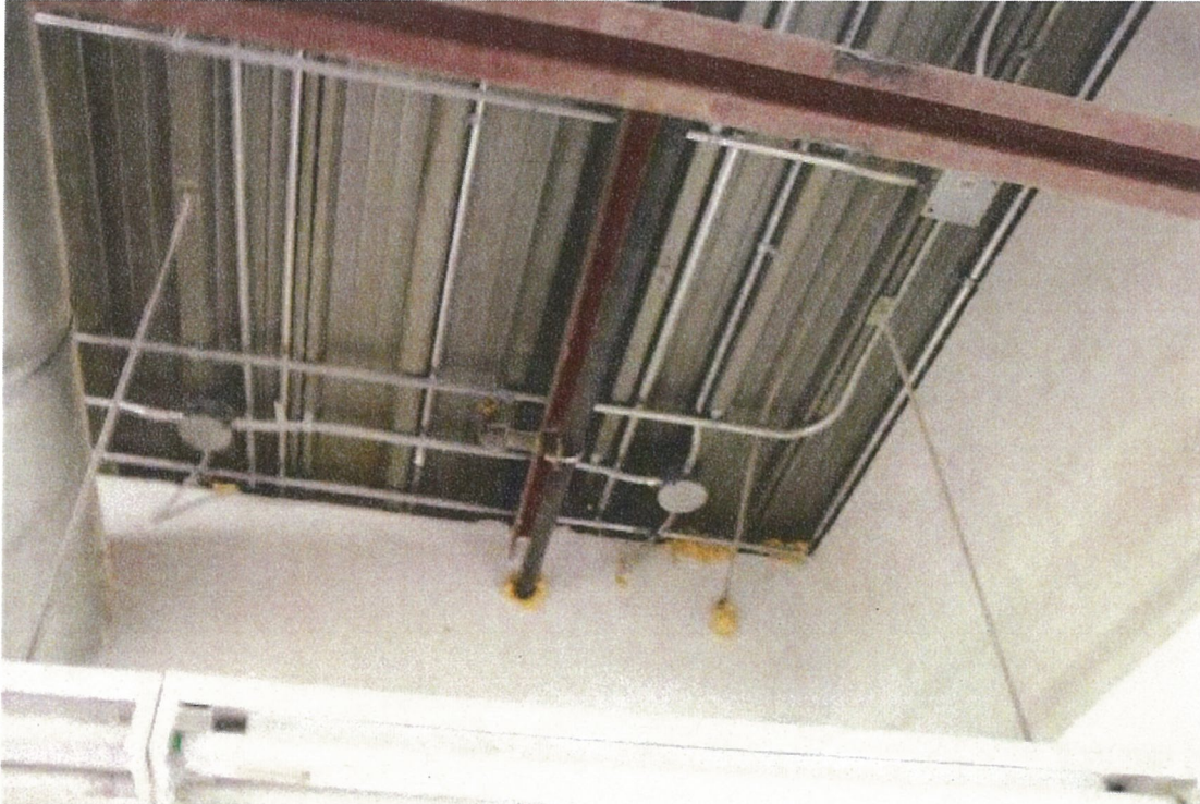
Southwest corner (Room 248) - Foam firestop.
