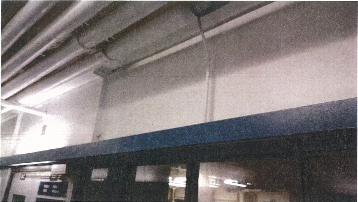
Metal structure above doors and windows (Hallway 216).
