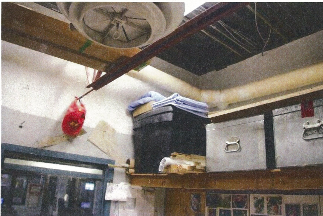
Northeast corner (Room 248) – pipe insulation – elbow.
