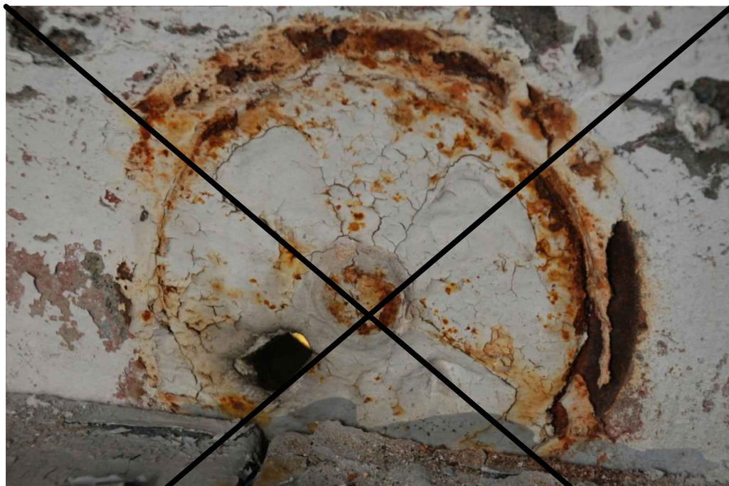
PHOTO 14 - DETAIL OF EXISTING LANTERN VENT, INTERIOR. REMOVE CAP AND REMOVE PAINT AND CORROSION. PROVIDE GASKET FOR SEAL AND REINSTATE CAP IN "CLOSED" POSITION. MAKE-GOOD ANY DAMAGE TO CONCRETE SUSTAINED DURING REMOVAL OF CAP.
