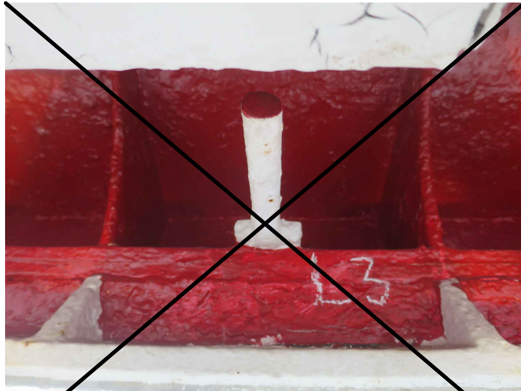
PHOTO 12 - DETAIL VIEW OF INTERIOR LANTERN TIE BAR TO BE REPLACED TO MATCH ORIGINAL. REFER TO STRUCTURAL.
