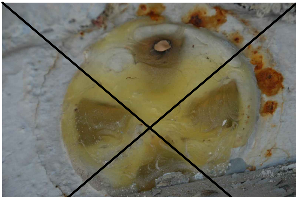
PHOTO 13 - DETAIL OF EXISTING LANTERN VENT WITH FAILED RUBBER SEAL, INTERIOR. REMOVE SEAL, PAINT AND CORROSION. PROVIDE REPLACEMENT CAP WITH GASKET AND INSTALL IN "CLOSED" POSITION. MAKE-GOOD ANY DAMAGE TO CONCRETE SUSTAINED DURING REMOVAL.
