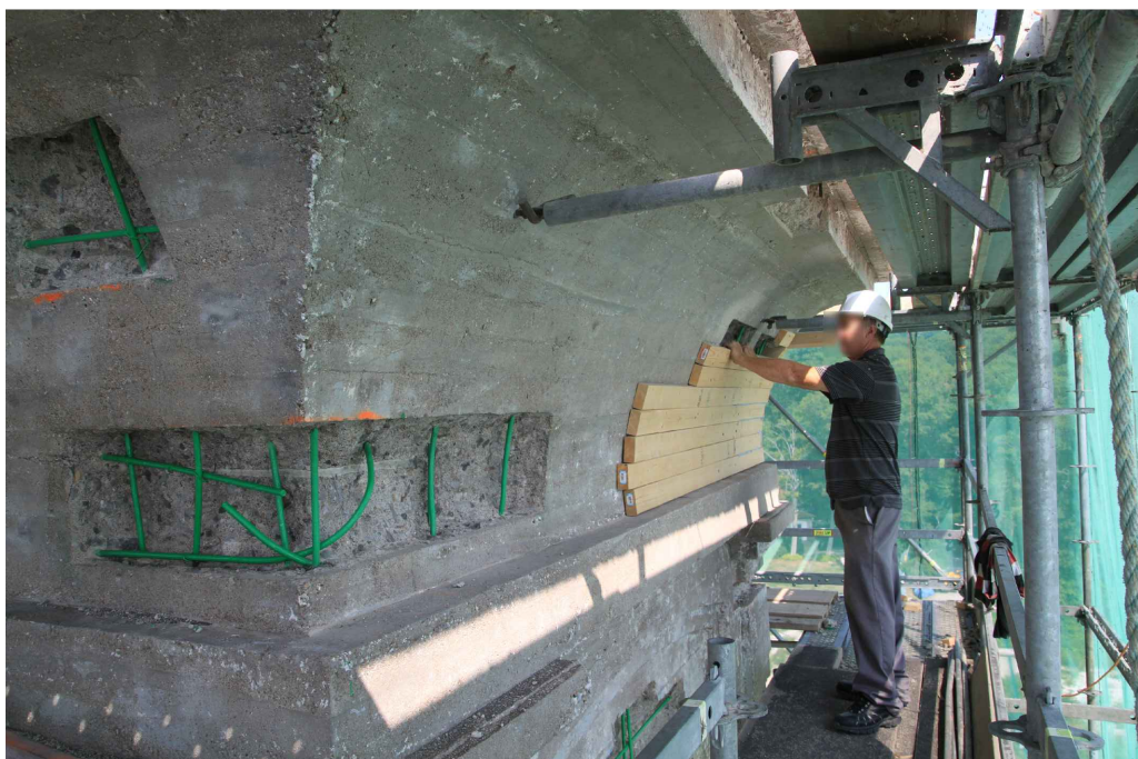
PHOTO 17 - EXAMPLE OF BOARD-FORMED CONCRETE FINISH TECHNIQUE BEING APPLIED AT POINT ABINO LIGHTHOUSE, ONTARIO. ALL CONCRETE REPAIRS TO HAVE BOARD FORMED FINISH.
