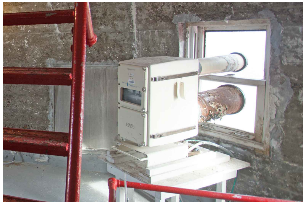
PHOTO 04 -INTERIOR VIEW SHOWING FOG DETECTOR TO BE REMOVED BY OTHERS. FOG DETECTOR WINDOW TO BE REMOVED WITH INSIDE FACE OF OPENING ROUGHENED AND FILLED WITH CONCRETE. REFER TO STRUCTURAL.
