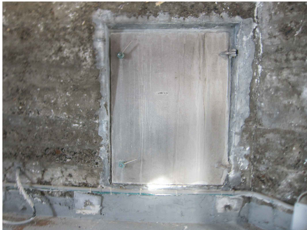
PHOTO 15 - INTERIOR OF SECOND FLOOR PLATFORM ACCESS DOOR. REMOVE DOOR, ROUGHEN EDGES AND FILL WITH CONCRETE. REFER TO STRUCTURAL.
