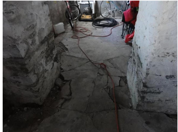
Photo 26: Differential cracks in heaved basement floor
