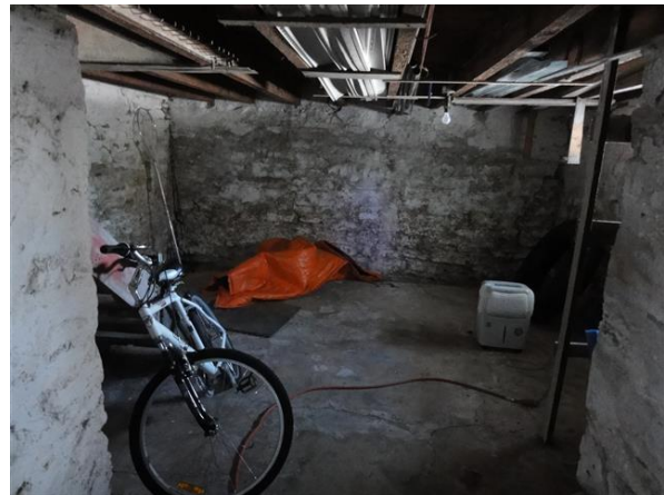
Photo 22: Stone foundation walls below tower
