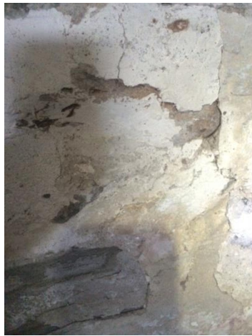
Photo 49: White parging on stone found. Samples 7A-C.
