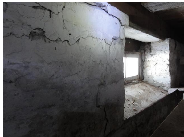
Photo 24: Cracked cement parging on stone and mortar
