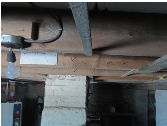
Photo 35: Deflected floor joist framing around fireplace chimney base
