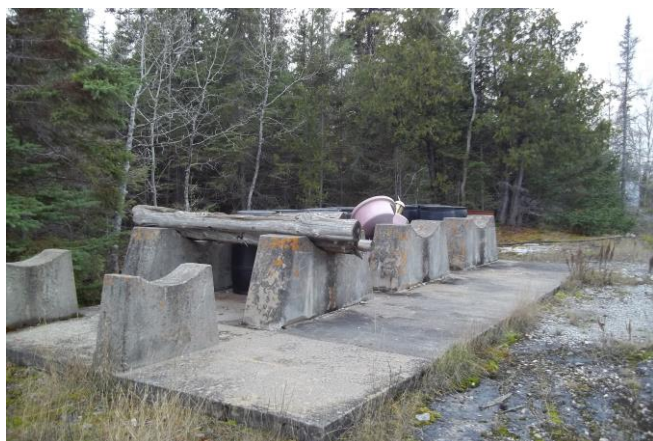
Photograph 11: [Exterior] Former tank nest area indicates that fuel storage tanks have previously been removed from the subject property.
