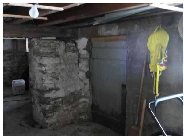
Photo 30: Support beams on top of stone foundation
