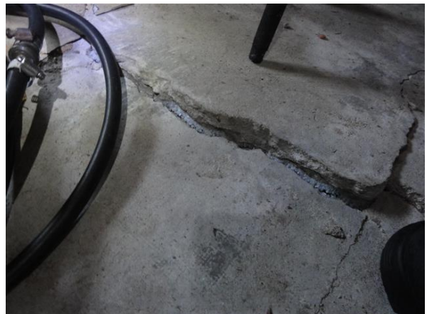
Photo 34: Differential cracks in heaved basement floor
