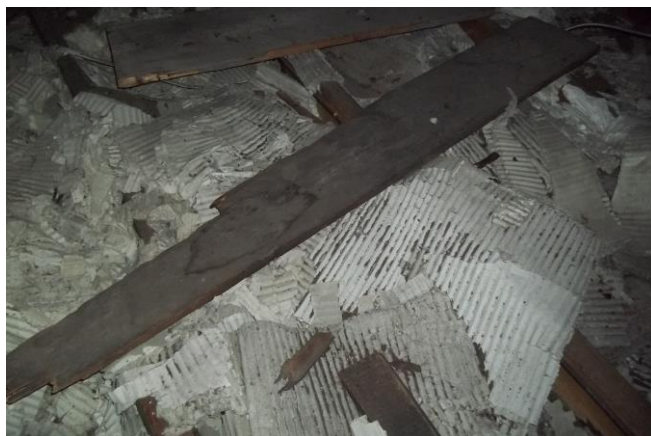
Photograph 6: [Fog Alarm Building] Asbestos-containing Air Cell pipe insulation debris observed in the attic.
