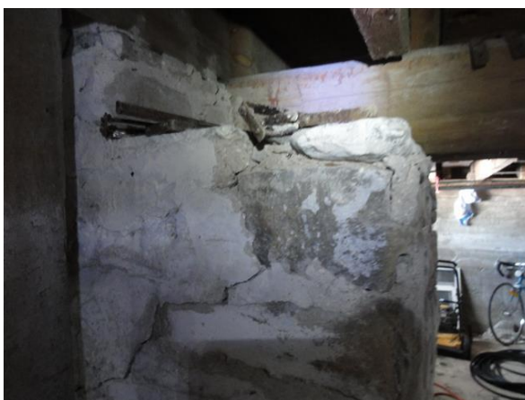
Photo 29: Support beams on top of stone foundation
