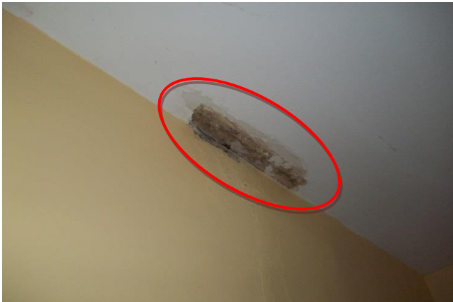
Photograph 15: [Assistant Lighthouse Keeper's Dwelling] Mould growth observed on the kitchen ceiling.
