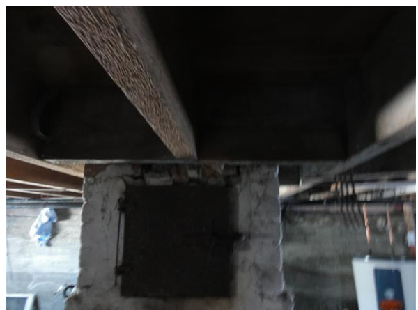
Photo 36: Deflected floor joist framing around fireplace chimney base
