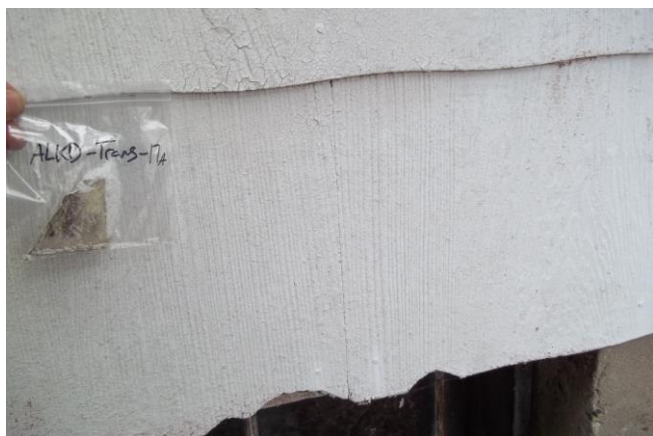
Photograph 7: [Assistant Lighthouse Keeper's Dwelling] Asbestos-containing transite siding panels observed on outside of building (Sample set ALKD-TRANS-17).
