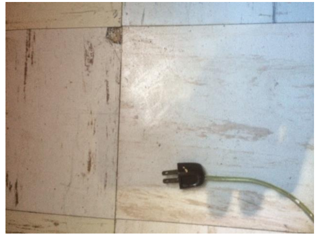
Photo 44: Vinyl floor tile and mastic. Samples 2A-C
