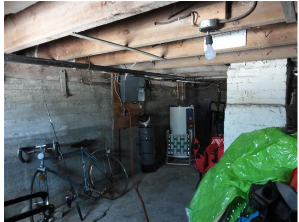
Photo 32: Poured-in-place concrete foundation walls and wood floor joists supporting light station residence
