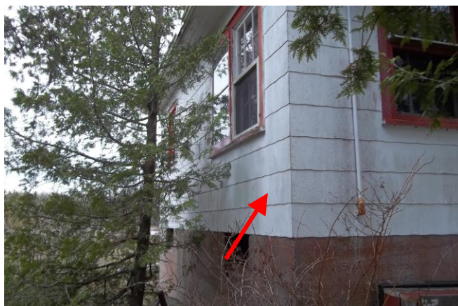
Photograph 8: [Assistant Lighthouse Keeper's Dwelling] Asbestos-containing transite siding panels observed on outside of building (Sample set ALKD-TRANS-17).
