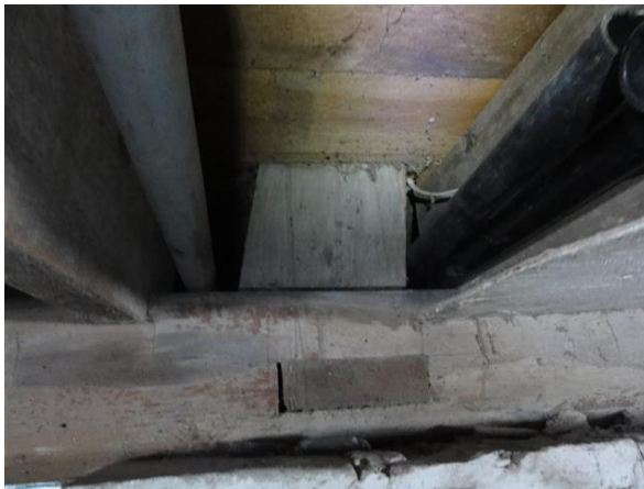
Photo 27: Tower's wood corner post and support beams on top of stone foundation wall
