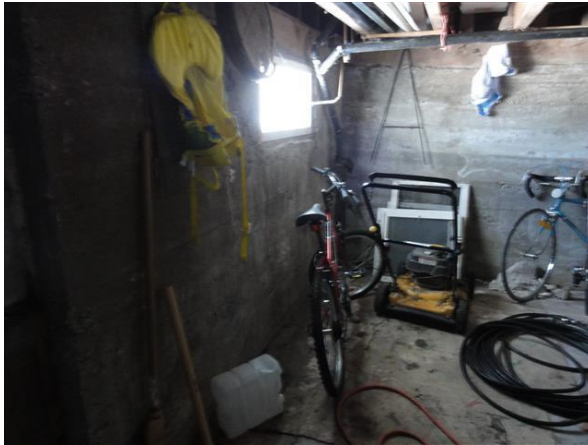
Photo 31: Poured-in-place concrete foundation walls below light station residence
