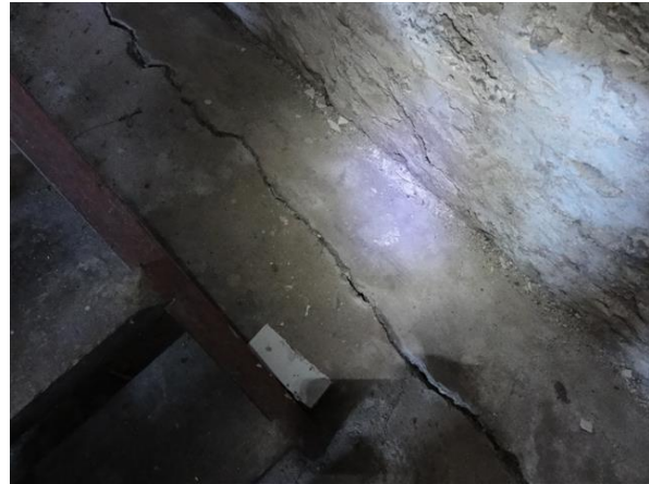
Photo 38: Differential cracks in heaved basement floor
