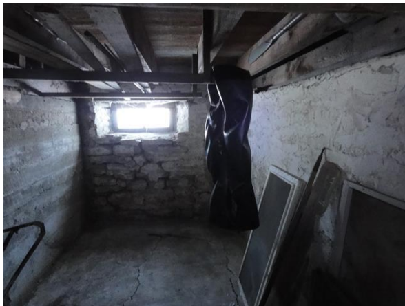
Photo 39: Poured-in-place concrete and stone foundation walls under south section
