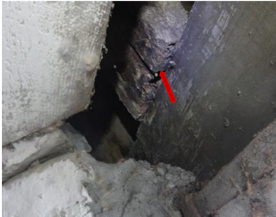
Photo 25: Dry rot in base of tower's wall stringers
