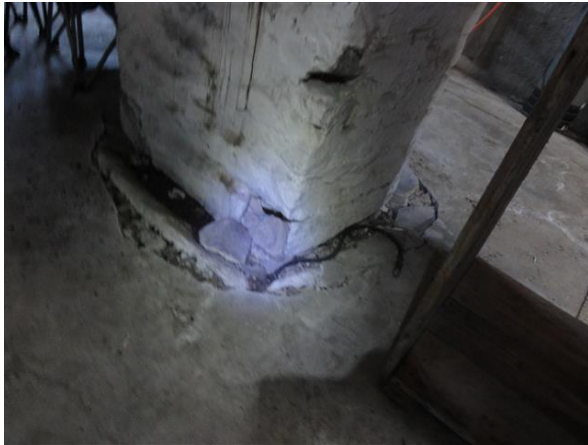
Photo 37: Differential cracks in heaved basement floor
