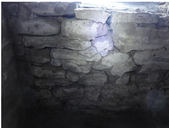
Photo 23: Deteriorated mortar in tower's stone foundation
