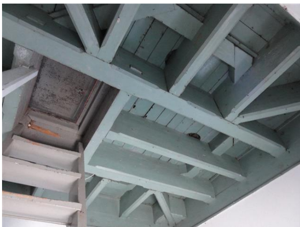
Photo 41: Beacon house platform framing, access ladder and floor hatch
