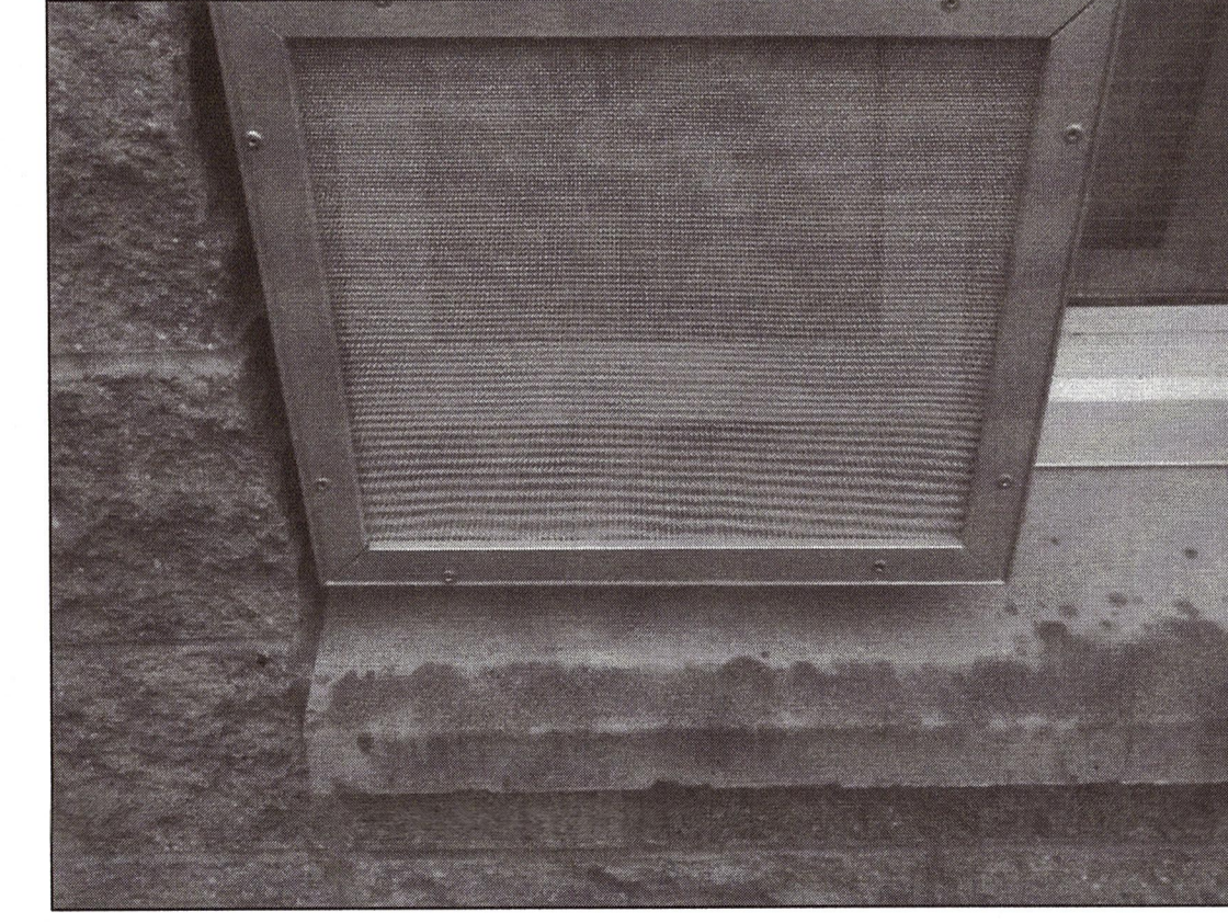
EXISTING SECURITY AWNING WINDOW ENCLOSURE - BUILDING C
