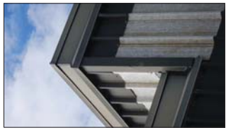
ENCLOSURE CORRUGATED GLAZED PANEL CORNER TRANSITION
