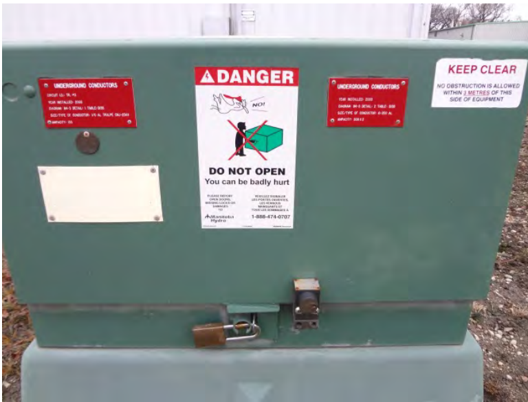
Photo – 8 Transformer TR#2 – 300Kva 12470-347/600V
