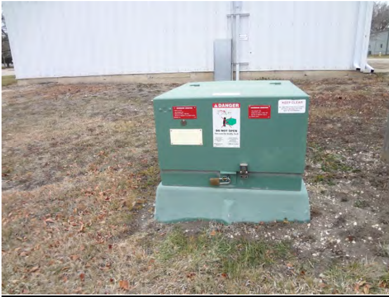
Photo – 9 Transformer TR#4 – 50Kva 7200-347/600V (Identical to transformer TR#3)
