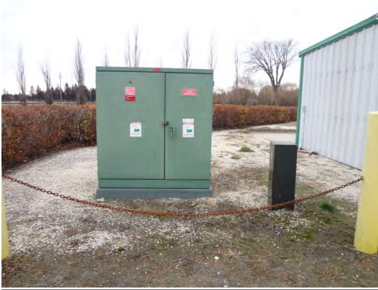
Photo – 7 Transformer TR#1 – 750Kva 12470-347/600V
