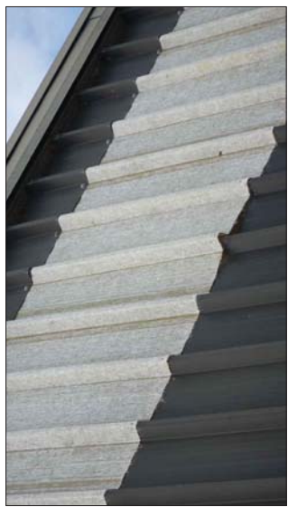
FIGURE 1. EXISTING CORRUGATED GLAZED PANEL TRANSITIONS
