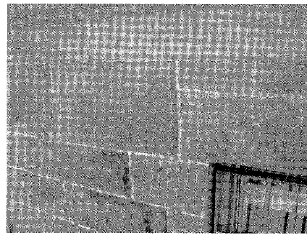
3 SURFACE CRACKS AND CRACK IN CORNER OF LINTEL
