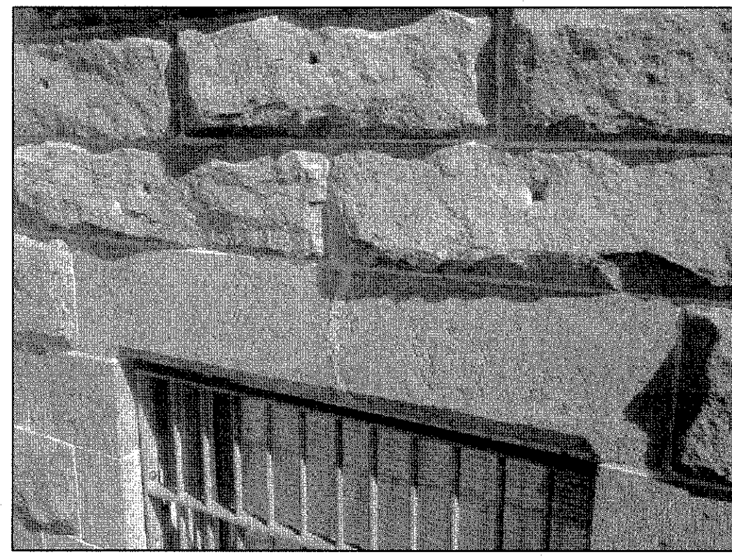
1 CRACK IN STONE LINTEL
