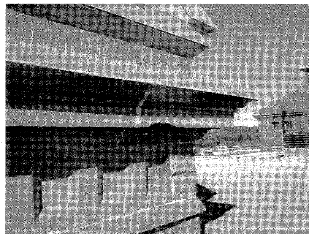
7 DAMAGED STONE, AND STONE EROSION AT SE CORNER OF TOWER
