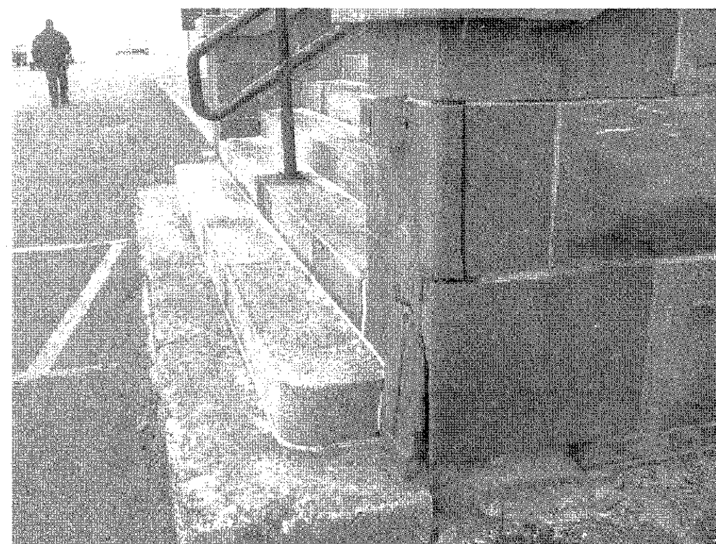
6 DAMAGED STONES AT SW CORNER OF ENTRANCE STAIRS - METAL HANDRAIL BEYOND
