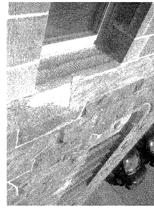
11 CRACKED STONE SILL - NOTE ANTI-PIGEON SPIKES (TYP. LVL. 4 WINDOWS)
