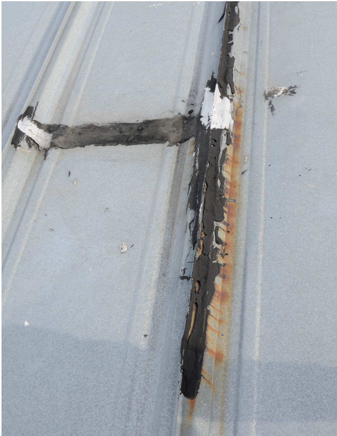
Photo 11: Typical metallic paint and asphalt mastic applied at the standing seam and head / end laps in the metal roof system. All asphalt, metallic paint material and surface corrosion to be removed prior to installation of new microsealant tape material
