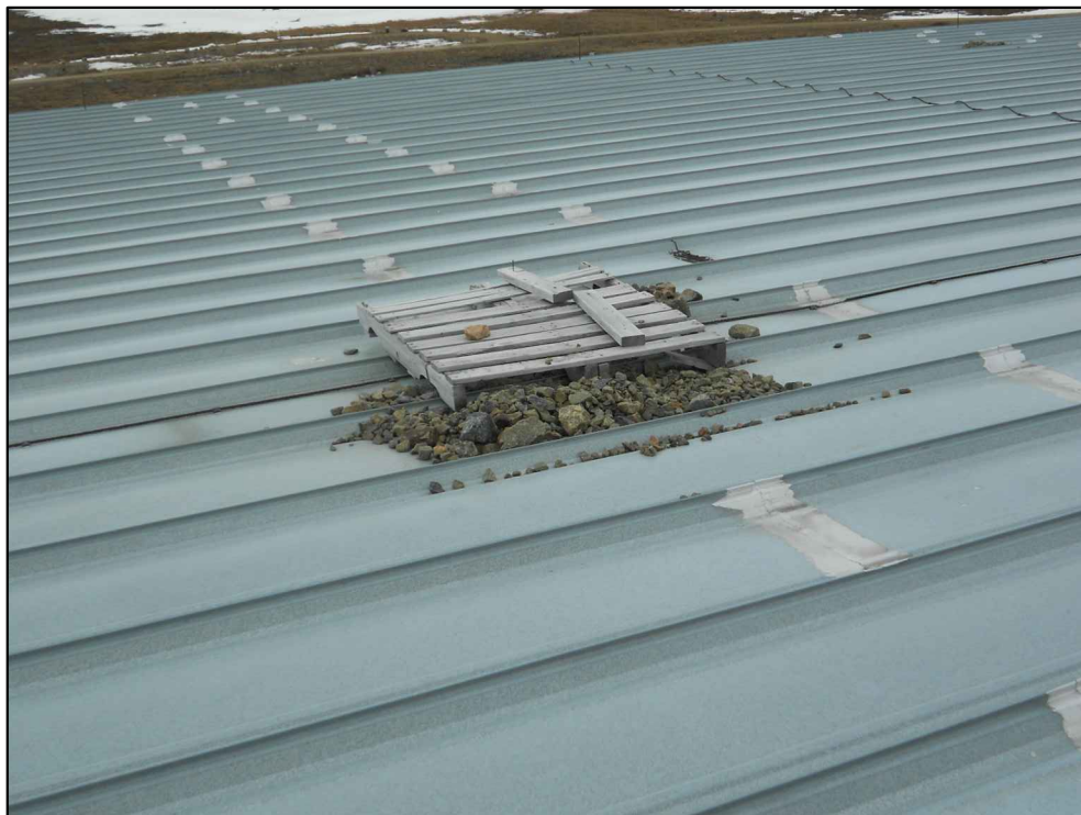
PHOTO_9: TYPICAL STONE PILE ON ROOF DECK (4 LOCATIONS)
