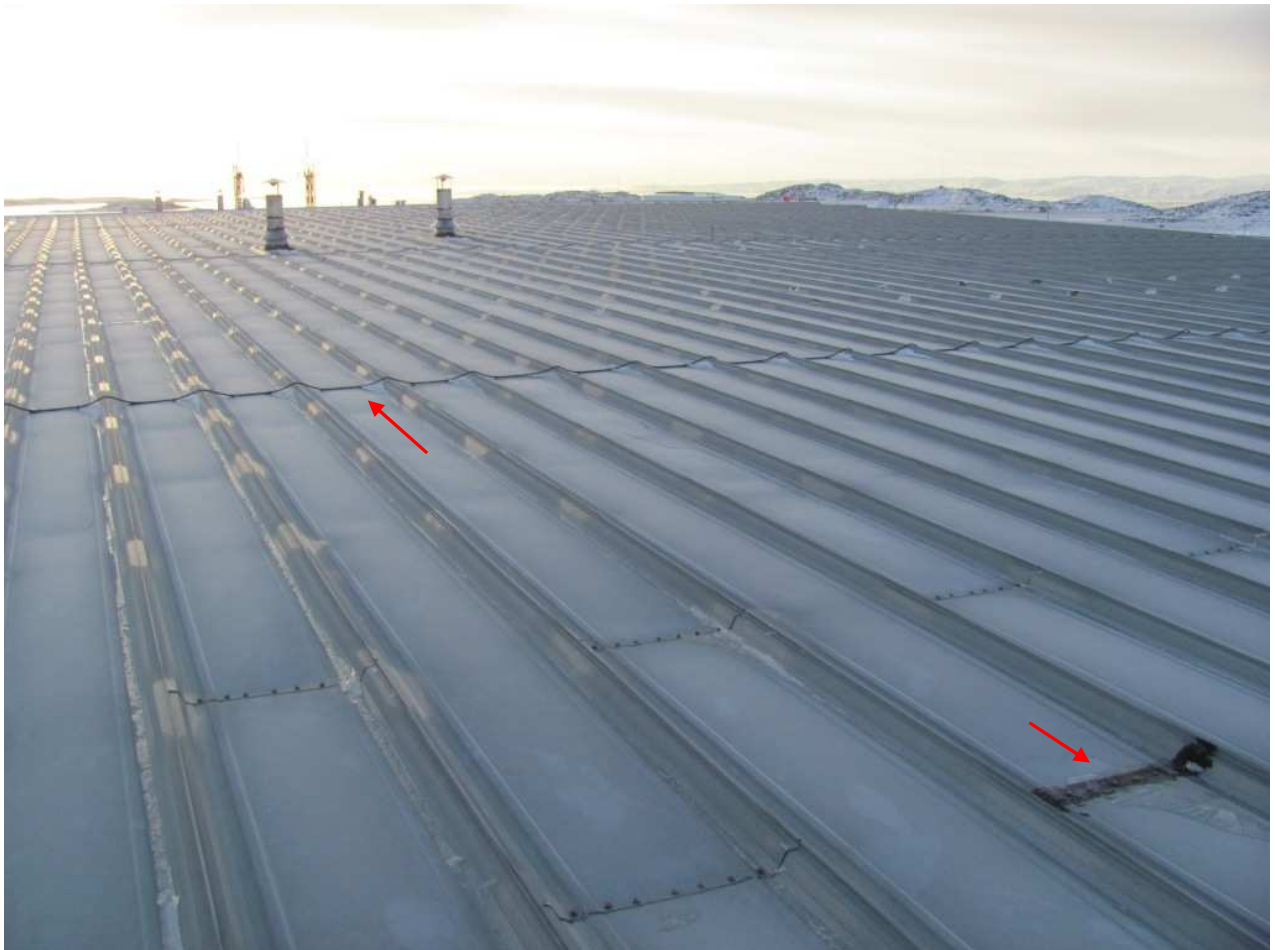
Photo 2: Typical view of the main roof deck, photograph taken from the mid-section of the roof deck with a view of the south half of the hanger roof assembly. Note the lighting arrest system that spans the length and width of the roof deck and the bitumen mastic.
