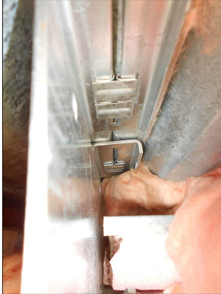
PHOTO_14: VIEW OF EXISTING PANEL CLIP FROM THE UNDERSIDE OF THE ROOF SYSTEM
