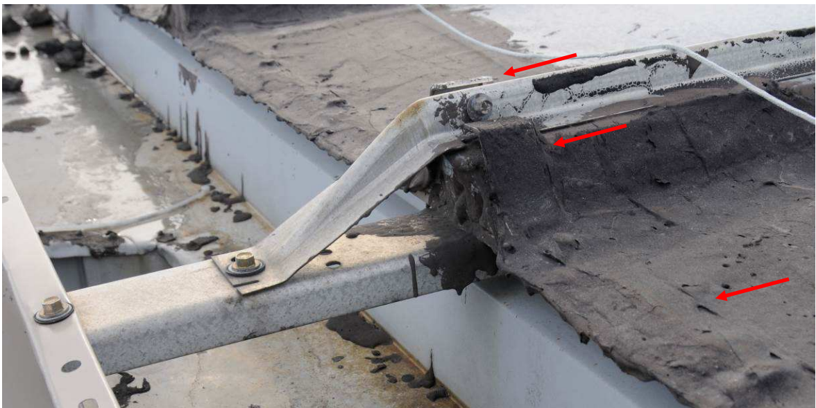
Photo 17: Typical Installation of asphalt mastic at the north and south ends of the roof deck. Note the installation of the rain gutter support bracket and end lap securement strap.
