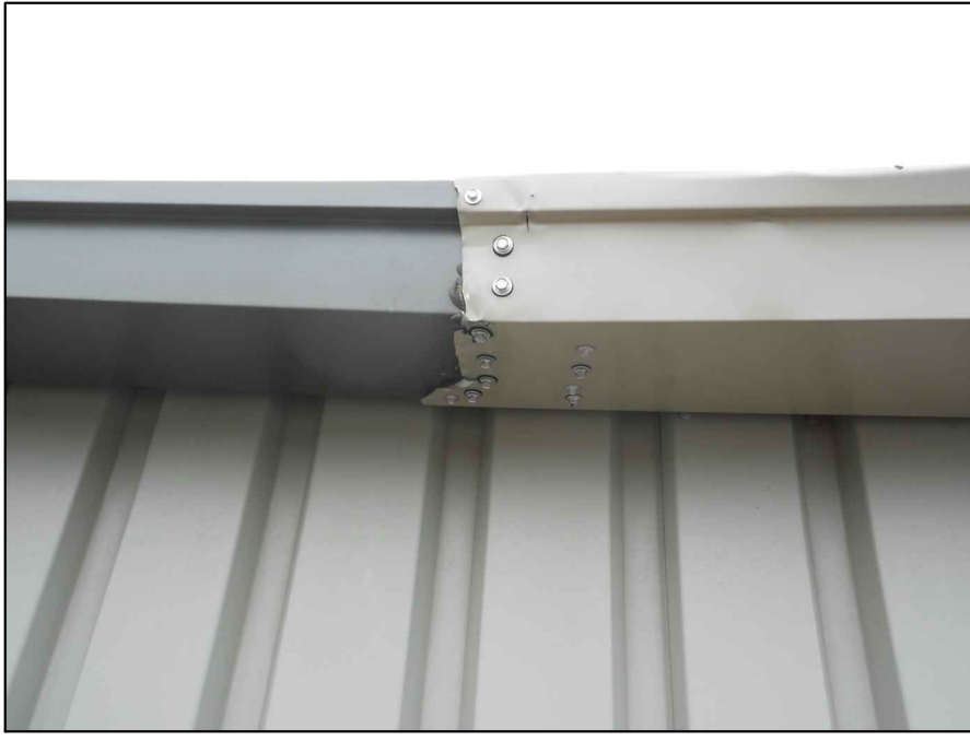
PHOTO_15: VIEW OF DAMAGED GUTTER TEMPORARY REPAIR
