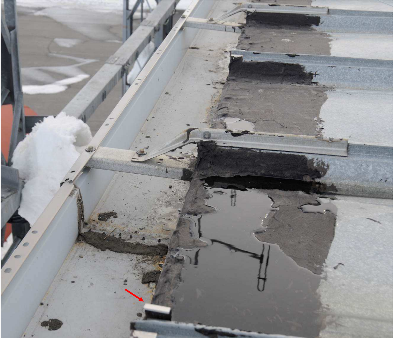
Photo 8: Typical end lap at the north / south elevations of the roof system. Note the installation of the rain gutter at these locations. All asphalt, metallic paint material and surface corrosion to be removed prior to installation of new material. Contractor to re-install existing rain gutter support brackets and end lap clamp where existing brackets and clamps are loose or dislodged.
