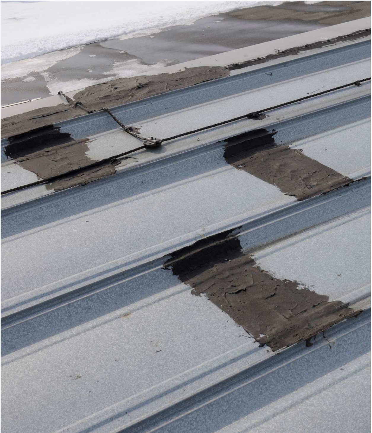
Photo 12: Typical asphalt mastic application at the head / end laps between metal roof panels. All asphalt material to be removed prior to installation of new microsealant tape material
