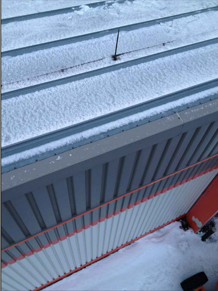
PHOTO_16: TYPICAL ROOF INSTALLATION AT (SIDE) PERIMETER OF ROOF DECK. SEE 2/R1.
