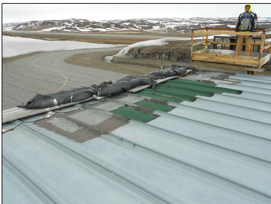
PHOTO_10: AREA OF DAMAGED ROOF DECK, NORTH EAST CORNER OF ROOF DECK
