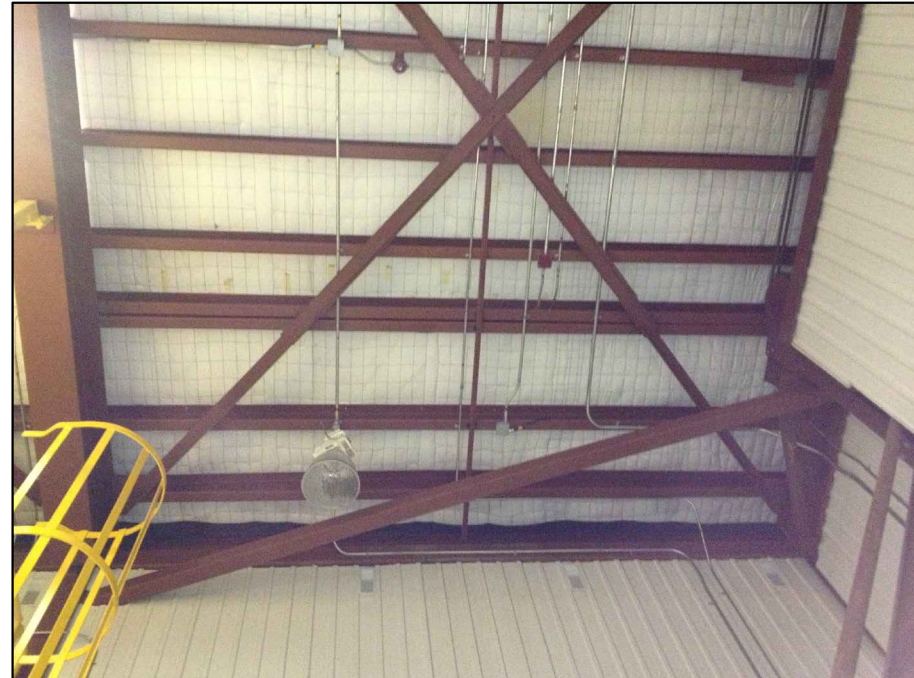
PHOTO_19: UNDERSIDE OF DAMAGED CORNER OF ROOF DECK AT NORTH/EAST CORNER OF ROOF SYSTEM
