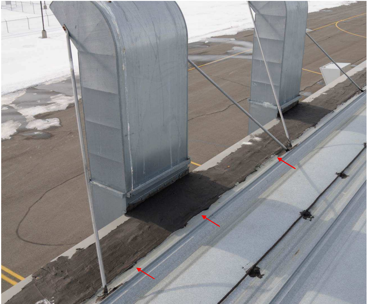
Photo 6: Typical asphalt mastic application at the interface between the sheet metal flashings along the eve of the roof system and metal roof panels on the east and west elevations. Photo taken along west elevation. All asphalt material to be removed prior to installation of new microsealant tape material along the joint between the metal pan and the sheet metal flashings along the east and west elevations.
