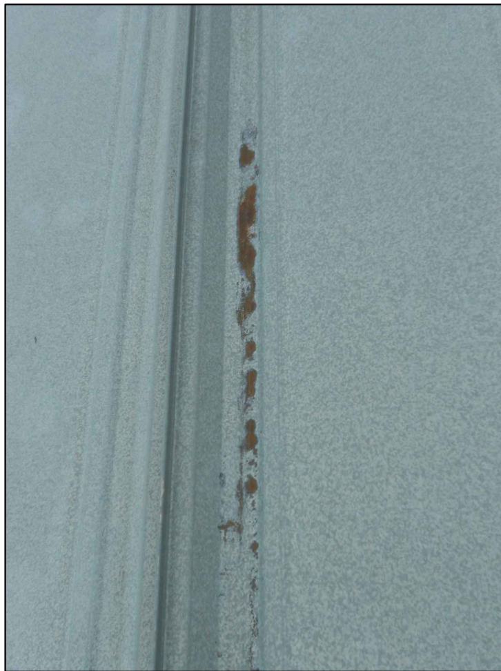
PHOTO_13: TYPICAL ROOF DECK CORROSION
