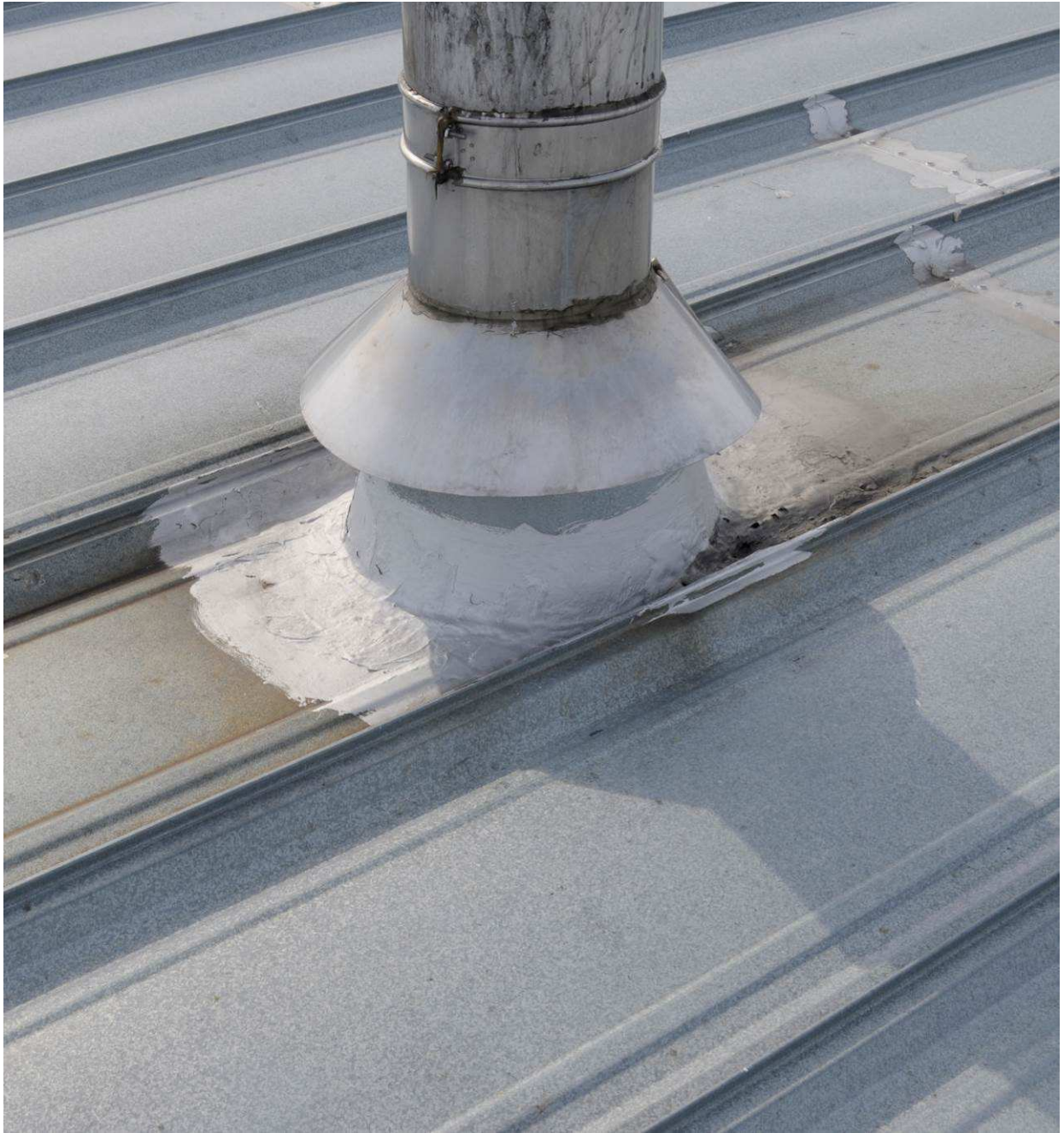
Photo 13: Typical metallic paint applied at the base of a exhaust stack. All metallic paint (and asphalt) material to be removed prior to installation of new bituminous membrane flashings.
