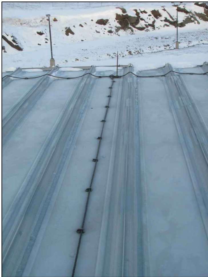
PHOTO_11: TYPICAL LIGHTNING ARREST SYSTEM
