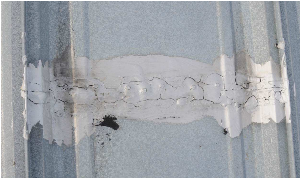
Photo 10: Typical metallic paint applied at the head / end laps between metal roof panels. All metallic paint (and asphalt) material to be removed prior to installation of new microsealant tape material
