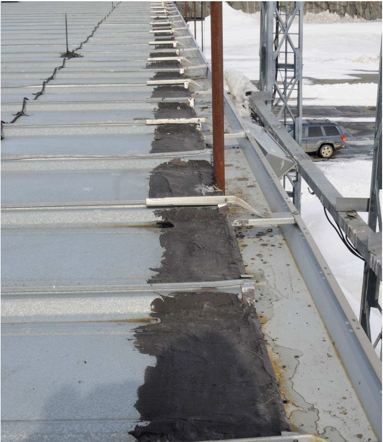
Photo 7: Typical asphalt mastic application at the interface between the sheet metal flashings along the eve of the roof system and metal roof panel on the north and south elevations. Photo taken at south elevation. All asphalt material to be removed prior to installation of new microsealant tape material.
