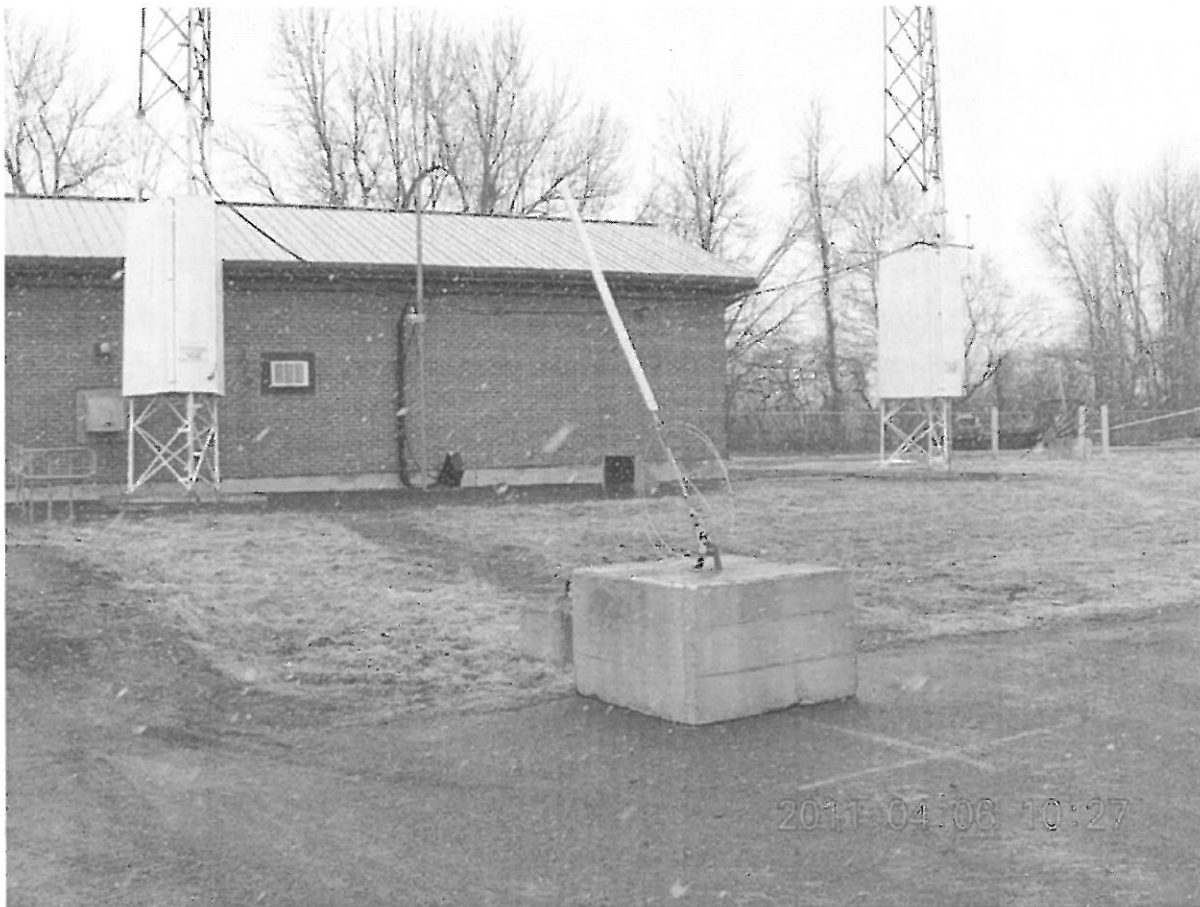
Figure 6: Current Temporary Guy Support
