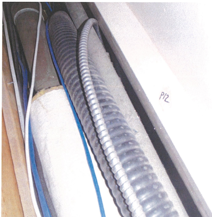
Photograph 66: Lead-based off-white trim paint in Room 106A above Room 143 ( Sample P12 ).
