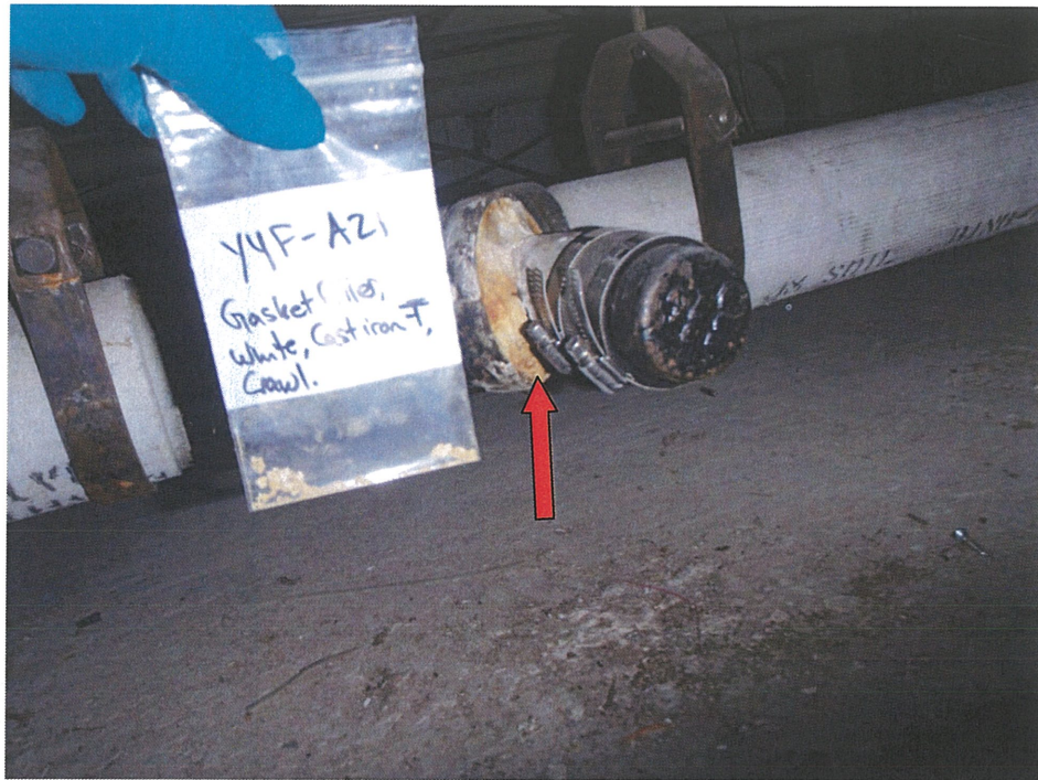
Photograph 33: Asbestos-containing bell and spigot joint filler ( Sample A21 ).
