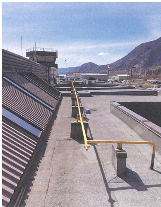
Photograph 8: Roof – Facing south (standing west of raised portion of roof).
