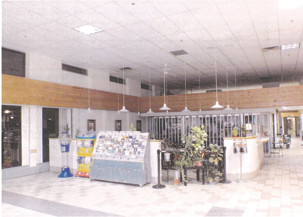
Photograph 15: Room 160 (restaurant) – Facing southeast.
