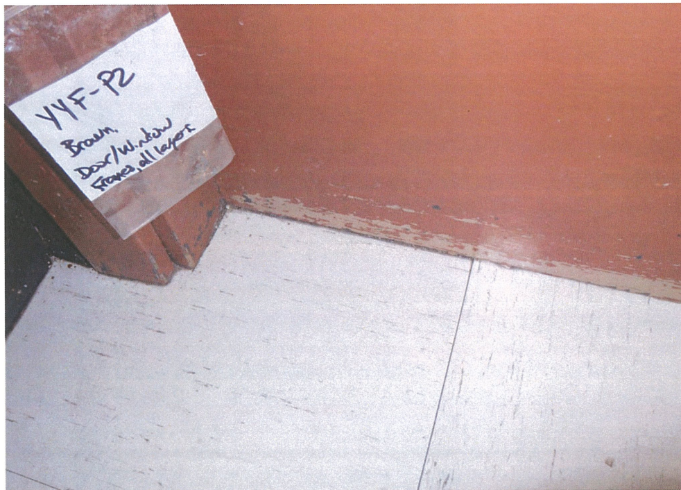
Photograph 60: Lead-based brown paint on door and window frames in Room 125 ( Sample P2 ).
