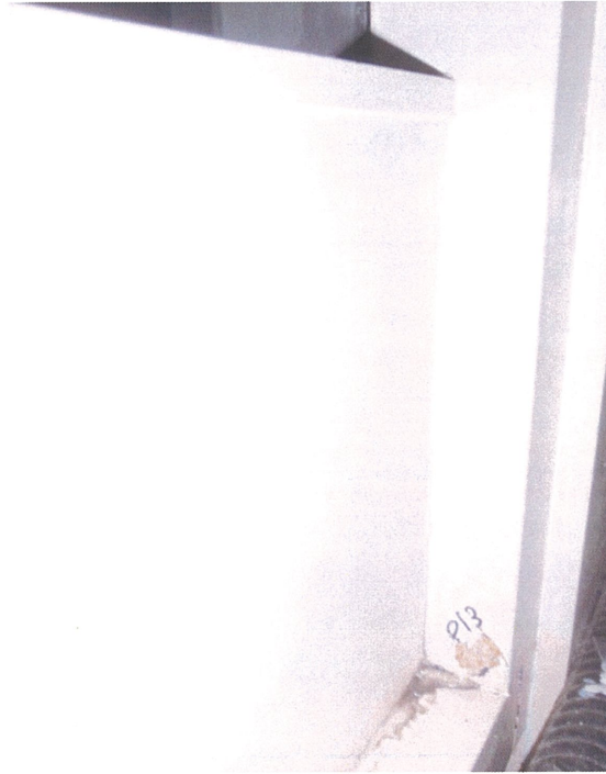
Photograph 67: Lead-based white paint in Room 106A above Room 143 ( Sample P13 ).
