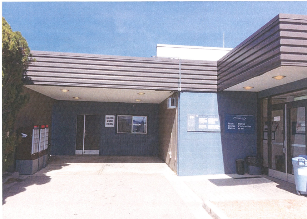
Photograph 4: South end of building – Facing north.
