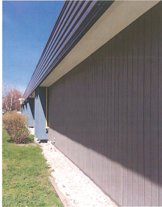
Photograph 3: Front (west) side of building – Facing north.
