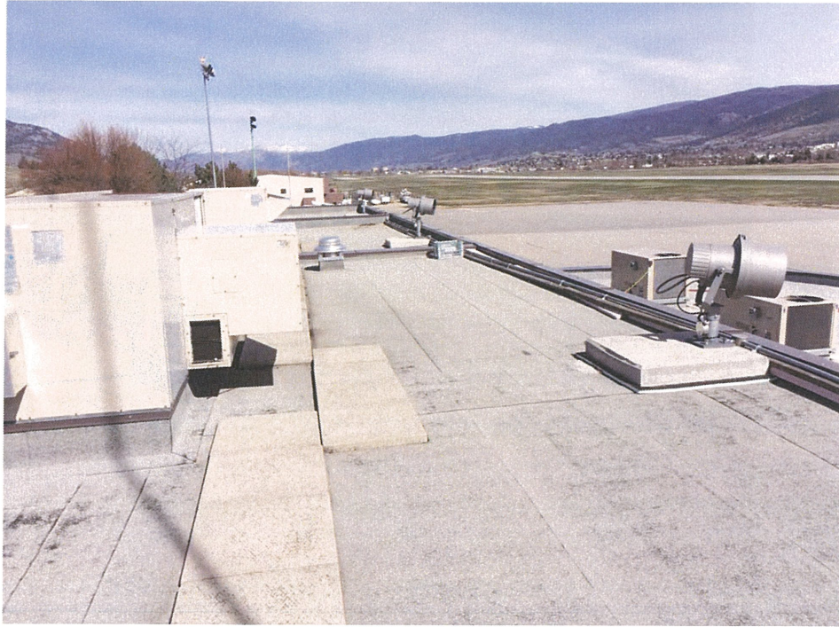
Photograph 9: Raised portion of roof – Facing north..
