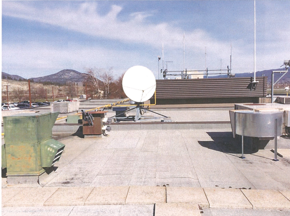
Photograph 7: Roof – Facing north towards raised portion of roof.
