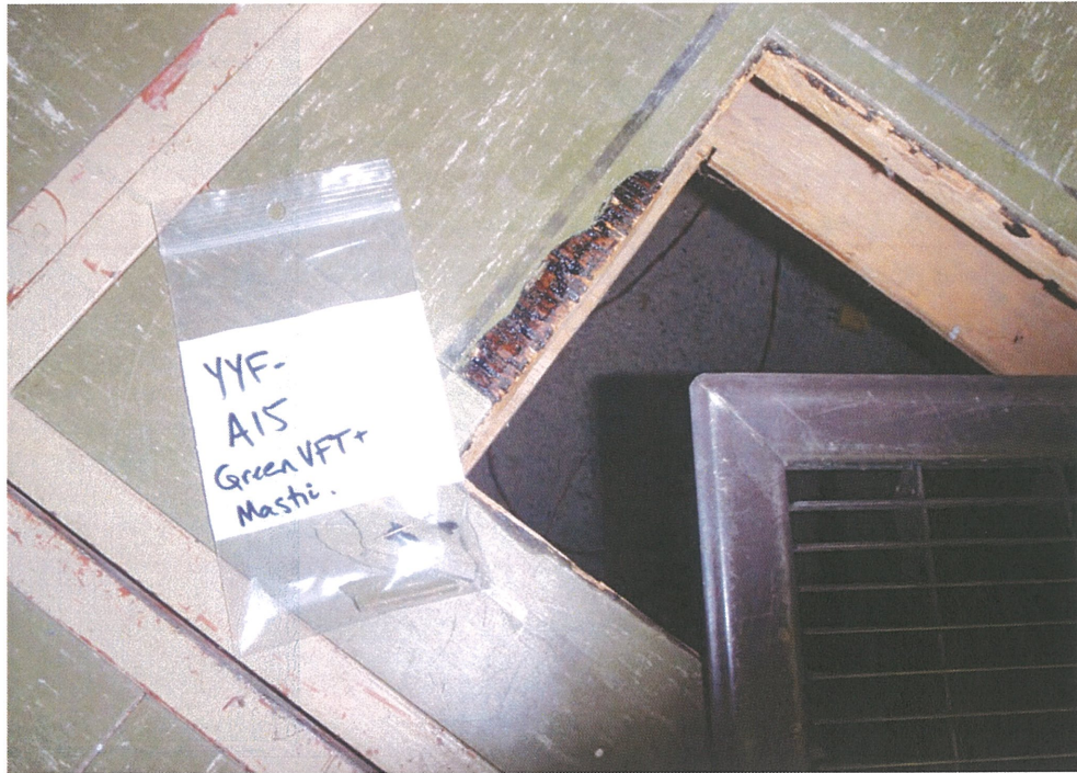
Photograph 31: Asbestos-containing green vinyl floor tiles ( Sample A15 ).
