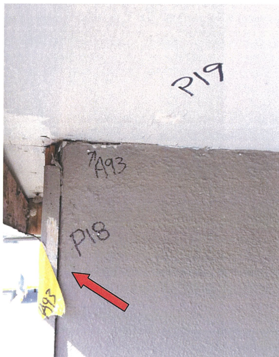
Photograph 70: Lead-based grey paint on wall of raised portion of roof ( Sample P18 ) and lead-based white paint on soffit of raised portion of roof ( Sample P19 ).
