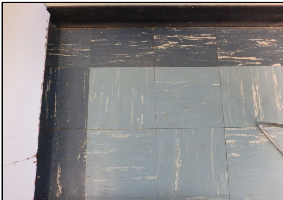
Photograph 1: Samples A-003 and A-011, Asbestos-Containing Blue Vinyl Floor Tiles with White Streaks, Lunchroom and Offices
