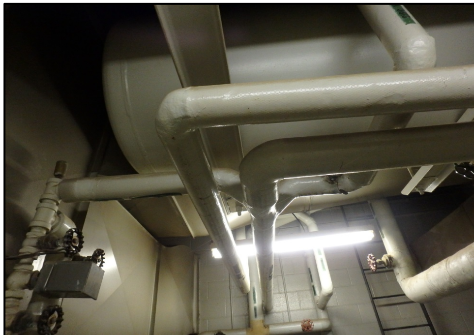
Photograph 7: Sample A-019, Asbestos-Containing Pipe Elbow Insulation, Boiler Room
