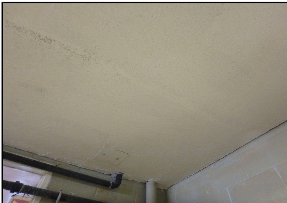
Photograph 5: Sample A-015, Asbestos-Containing Plaster Ceiling with Texture Finish, Cattle Area #2
