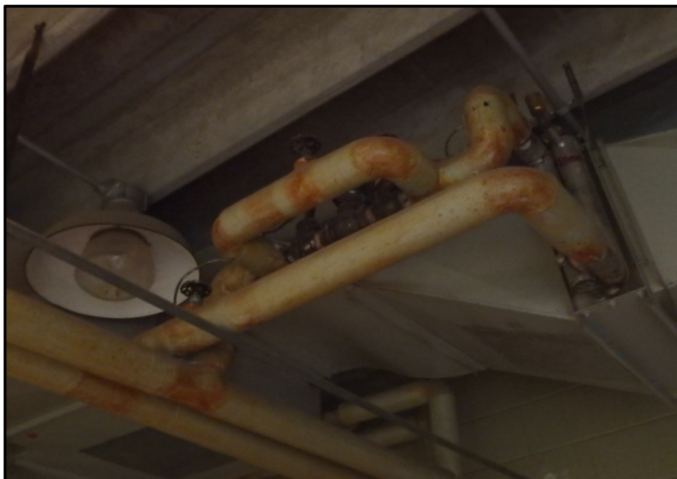
Photograph 6: Sample A-017, Asbestos-Containing Pipe Elbow Insulation, Storage #2
