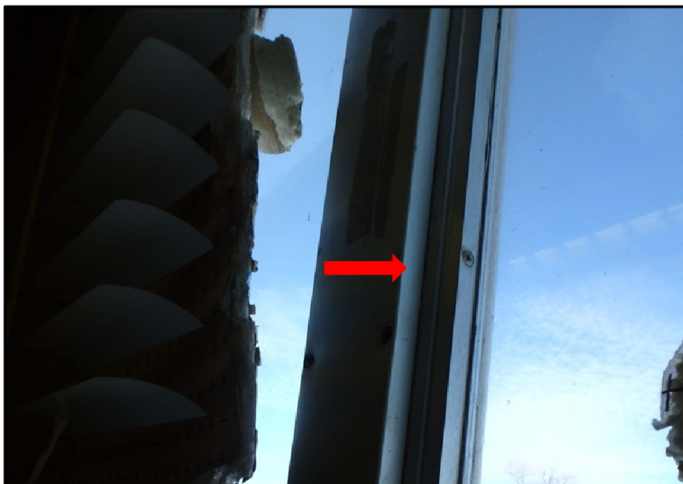
Photograph 4: Sample A-009, Asbestos-Containing Grey Window Putty, Lunchroom
