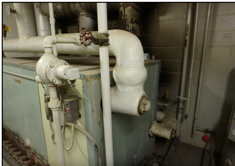
Photograph 8: Sample A-020, Asbestos-Containing Boiler Pipe Insulation, Boiler Room
