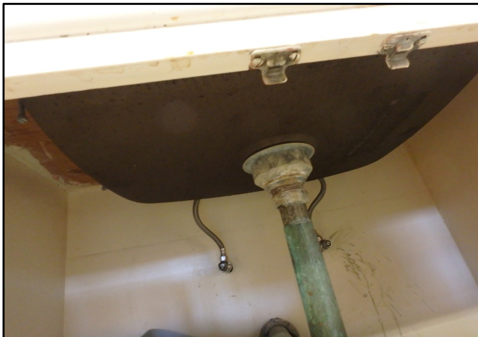
Photograph 3: Sample A-009, Asbestos-Containing Black Coating under Sink, Lunchroom
