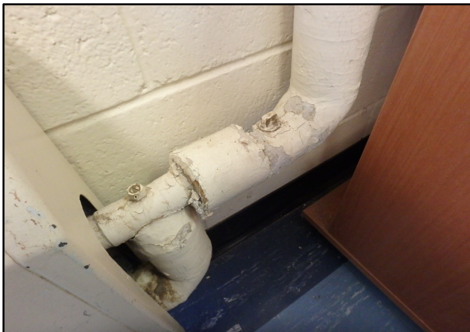
Photograph 2: Sample A-007, Asbestos-Containing Pipe Elbow Insulation, Women's Washroom
