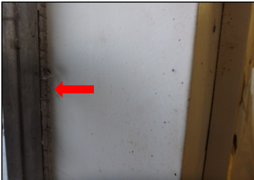
Photograph 9: Sample A-024, Asbestos-Containing Grey Window Caulking, Cleaning Room
