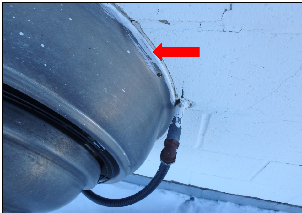
Photograph 11: Sample A-040, Asbestos-Containing White Caulking on Roof Wall Penetration, Exterior Wall
