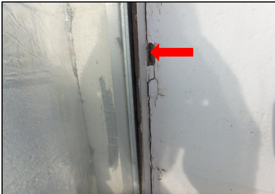
Photograph 10: Sample A-033, Asbestos-Containing White Window Caulking, Exterior
