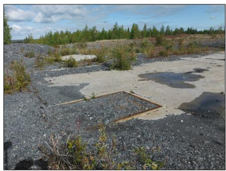
Photo B-13: Photo of the Mine Shaft Cap with the Mill Slab in the foreground (Stantec 2015 field program).
