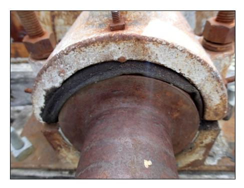
Photo 16: Asbestos containing break pad located in the Mill Building at Burnt Island
