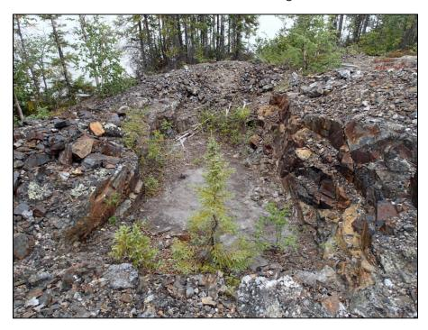
Photo G-2: West trench located in AEC 5 at the Treacy mine site. Note the presence of mill sediments at the base of the excavation.
