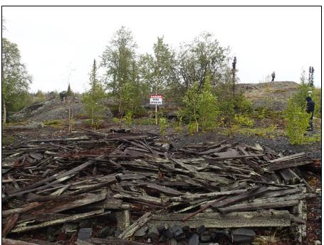
Photo B-18: Collapsed headframe at Zenith Island (Stantec 2015 field program).
