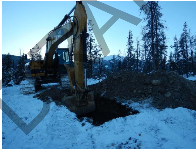
Excavation of TP14-05 on the west slope.
