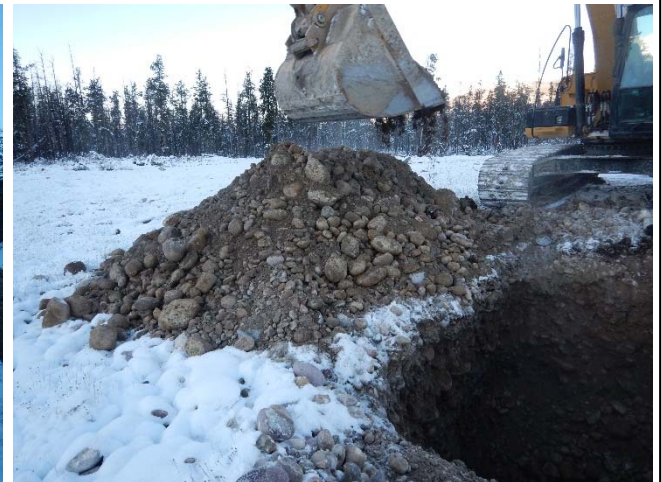
Gravel excavated from TP14-06
