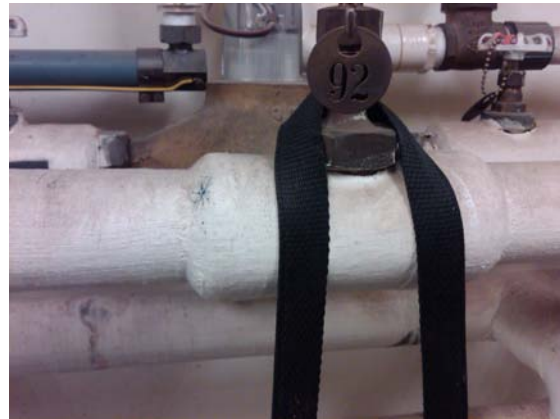
Photo 1.22 – H2O Valve insulation-sampled, no asbestos detected.
