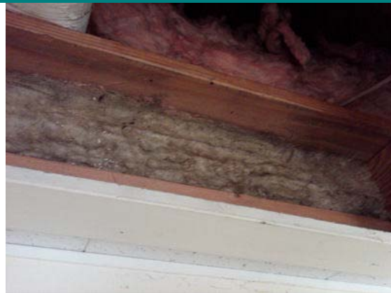
Photo 1.6 Building attic mineral fibre insulation bottom layer
