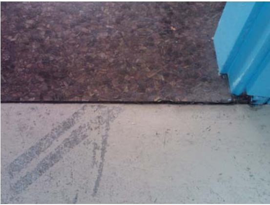
Photo 1.15 - Header House flooring
