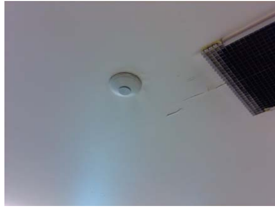
Photo 1.20 Smoke detector
