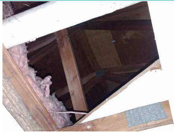
Photo 1.4 – Annex Building Room 42 attic - pink Fibreglass and Mineral Fibre Insulation.
