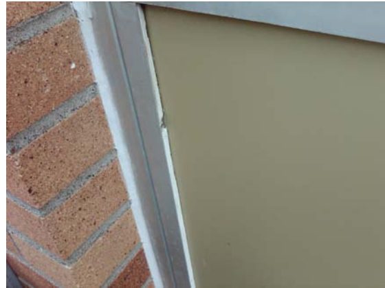
Photo 1.14 – Exterior board cement (no asbestos detected)
