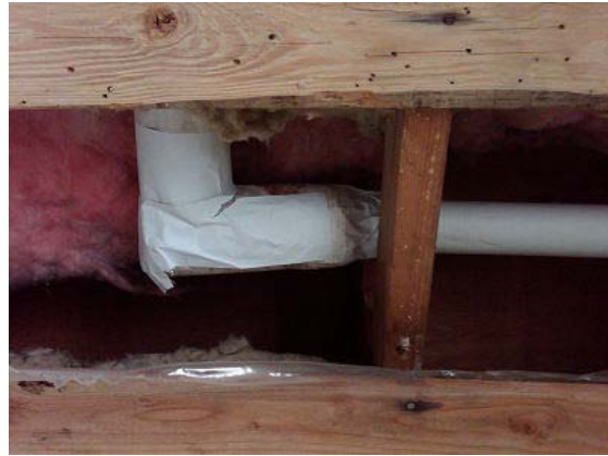
Photo 1.2 Annex Building Concealed Fibre Glass Insulation above Donna Conna Ceiling
