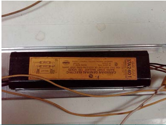
Photo 1.7 Annex Ballast-suspected to contain PCB's
