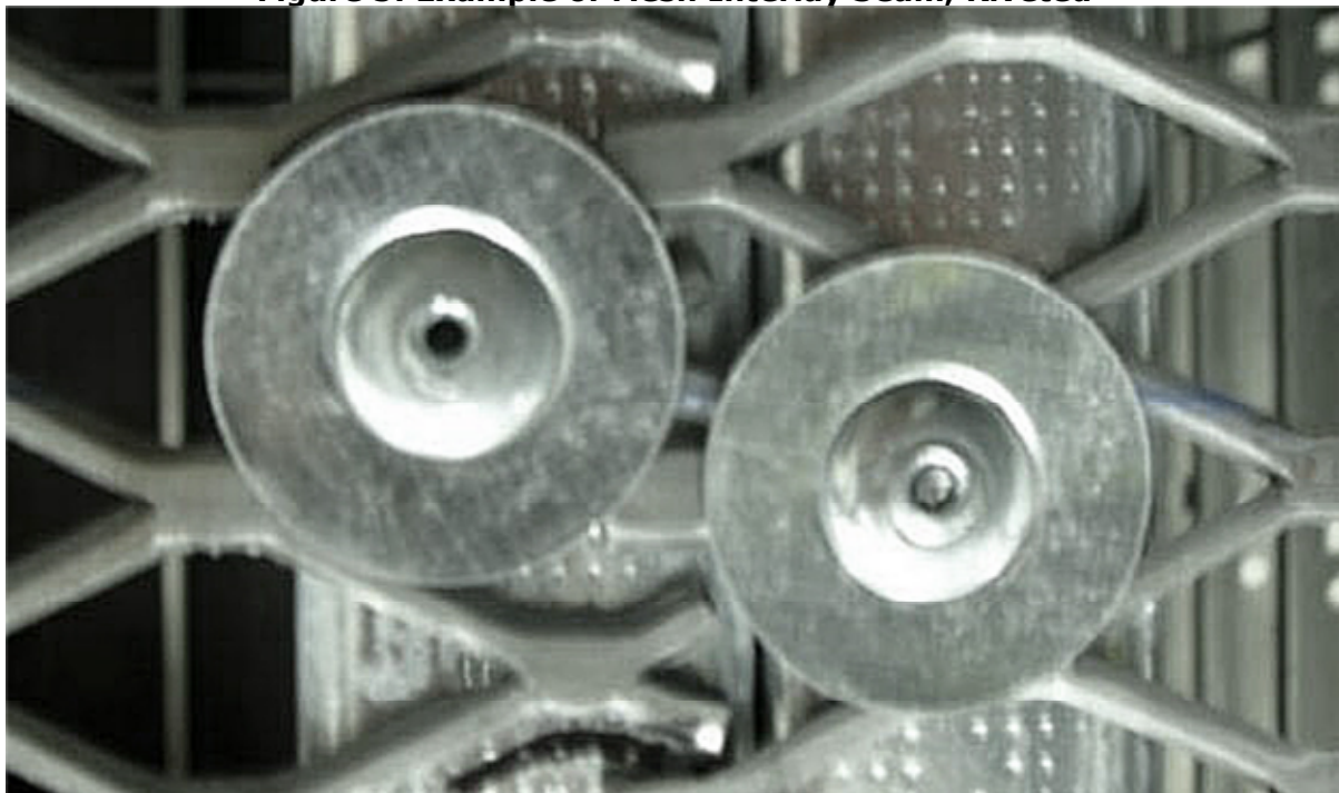
Figure 5: Example of Mesh Interlay Seam, Riveted
