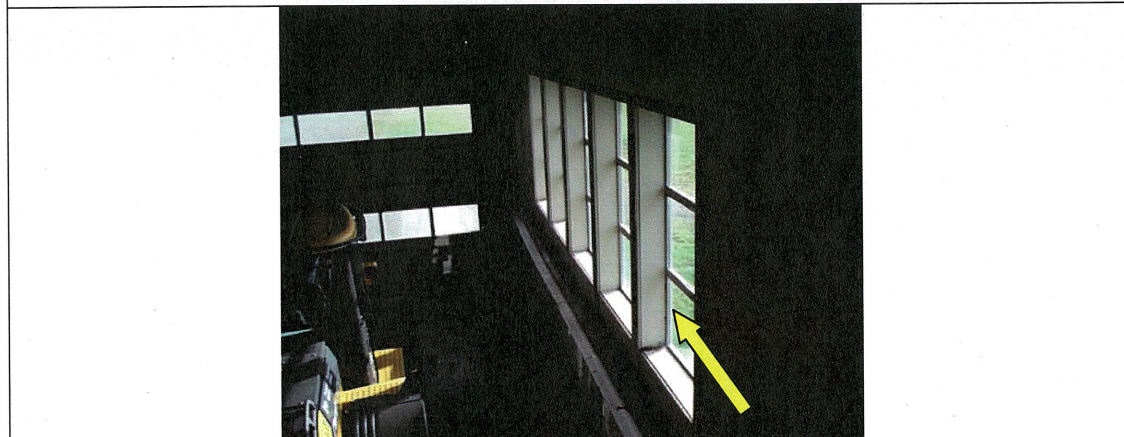
Typical asbestos-containing black window putty applied to the glazing of windows on the North and South facades
