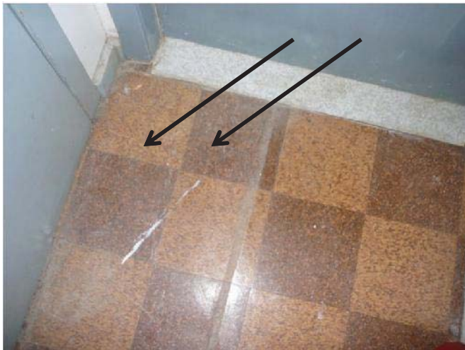
#14: Soils Research Building
