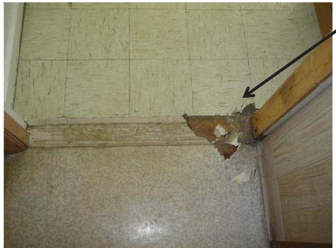
#14: Soils Research Building
