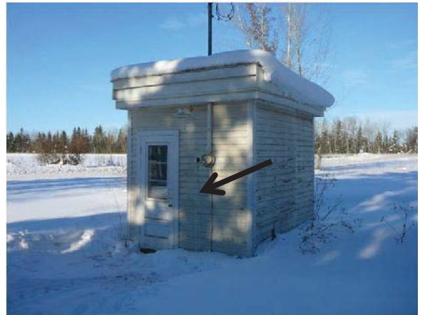
#57 Sewage Lift Pump House
