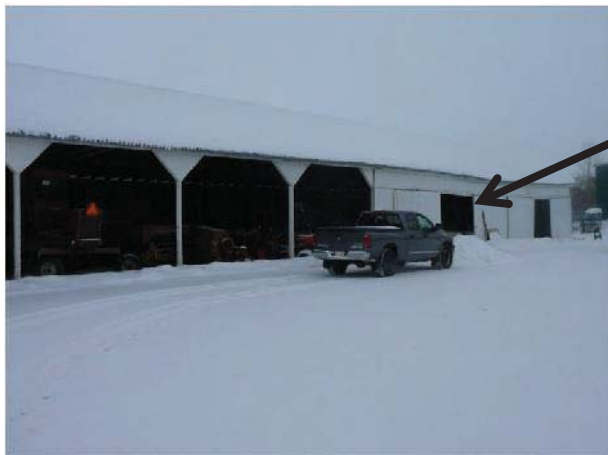
#10 Machine Pole Barn
