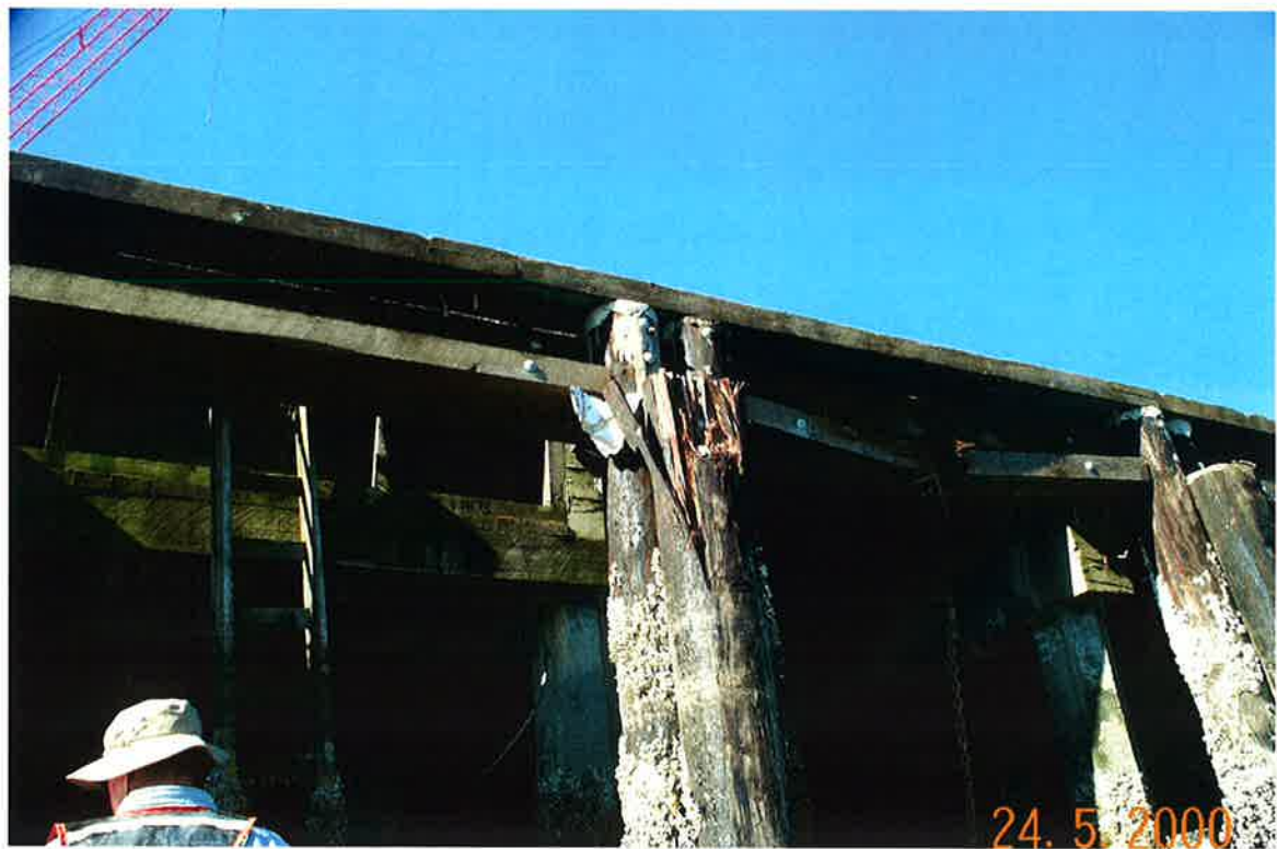
Photograph No. 10: Fungal decay in the top of the rub pile at Bent No. 33.
