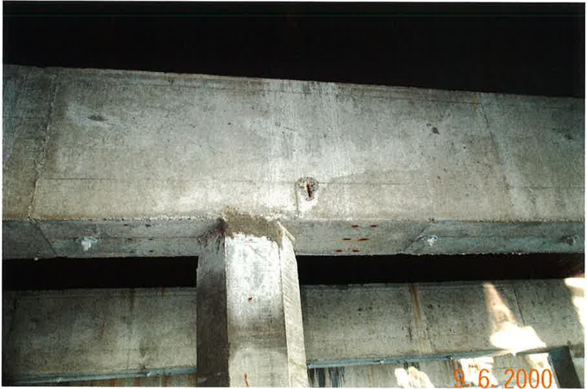
Photograph No. 7: Exposed, rusted reinforcement at Pile No. 36C.
