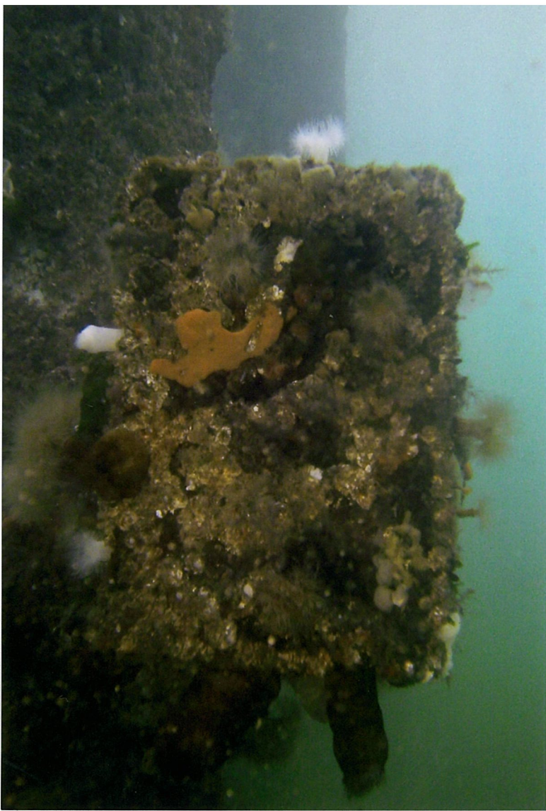
TIMBER CROSS BRACING DECAY AND ROT OBSERVED AT THE OLD FUEL FLOAT
