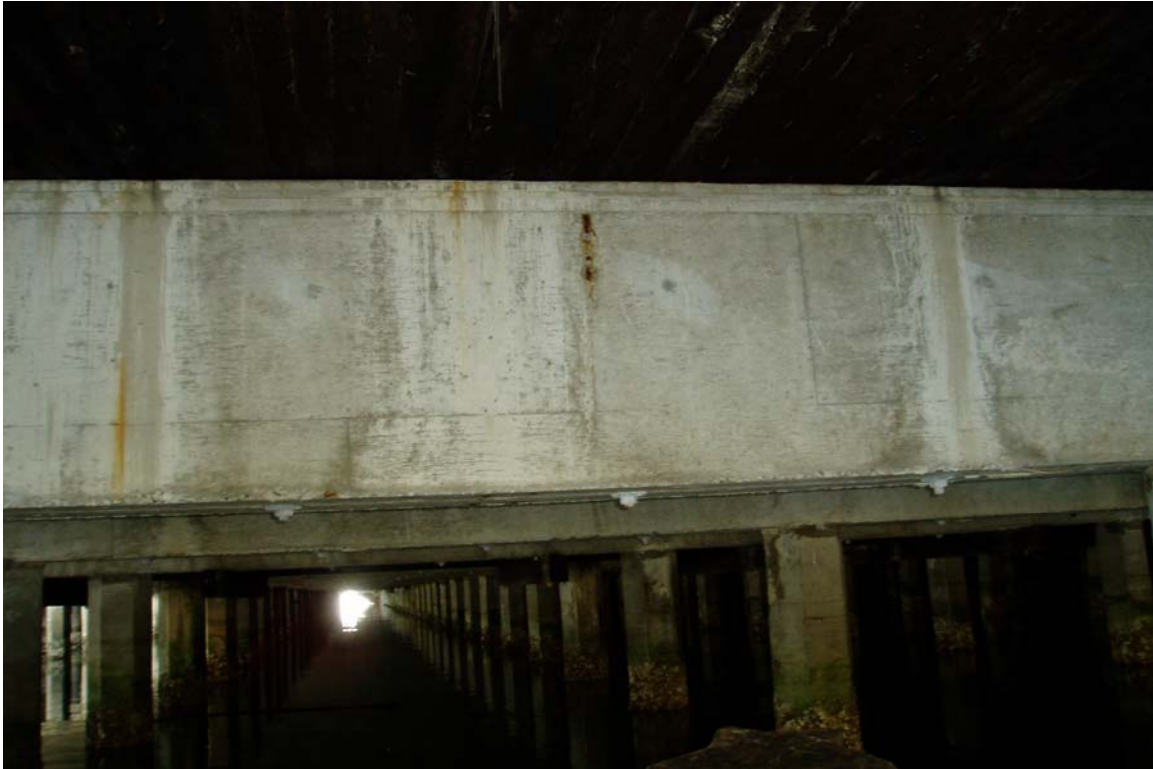
Photograph No. 8: Typical corrosion staining on pilecaps.
