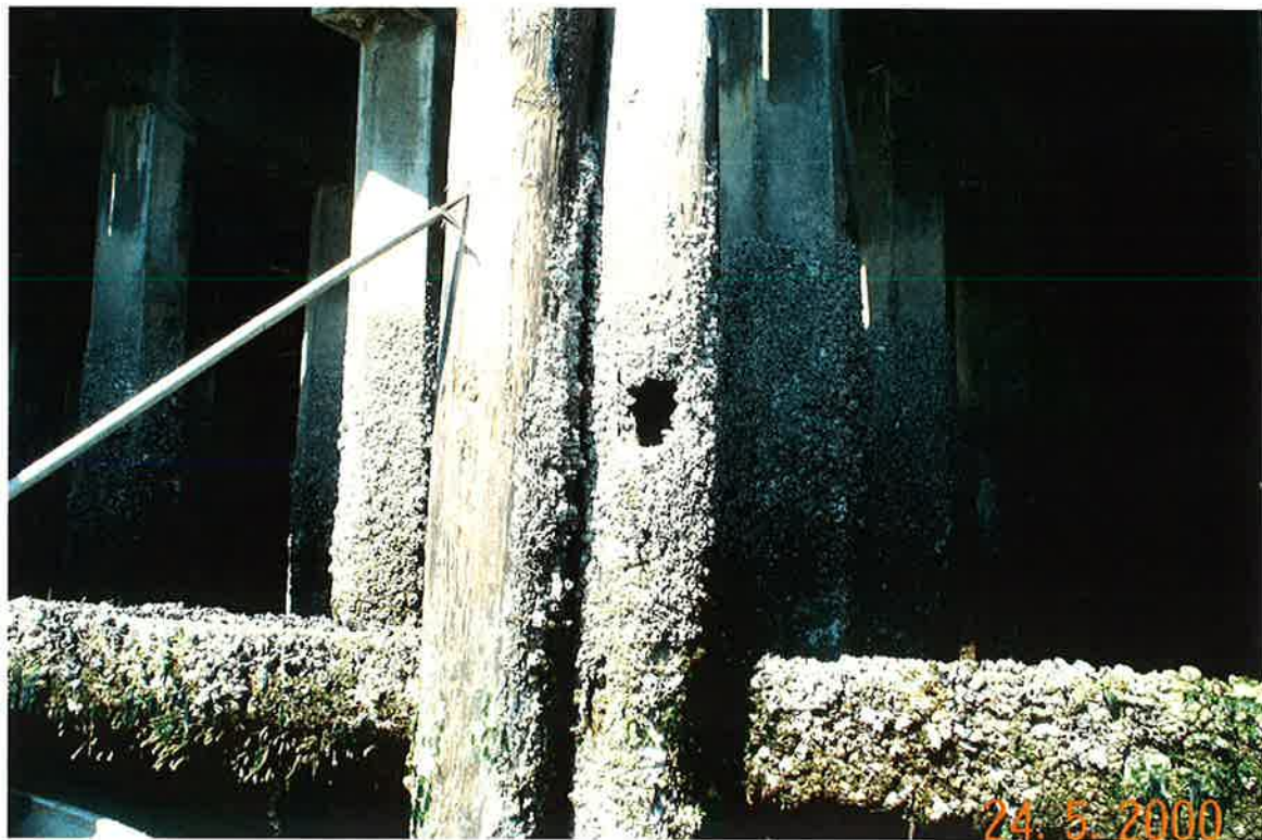
Photograph No. 12: Severe marine borer damage to Fender Pile No. 21A-2.
