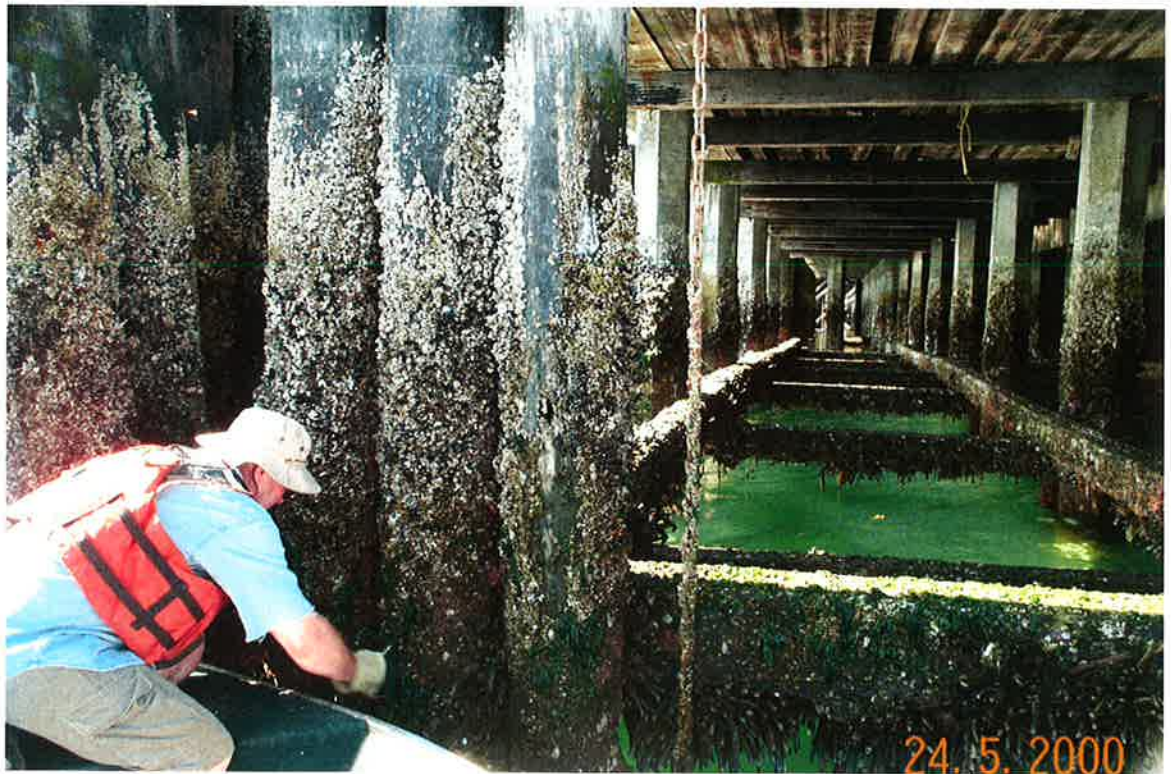
Photograph No. 14: Severe marine borer damage to Fender Pile No. 1-3.
