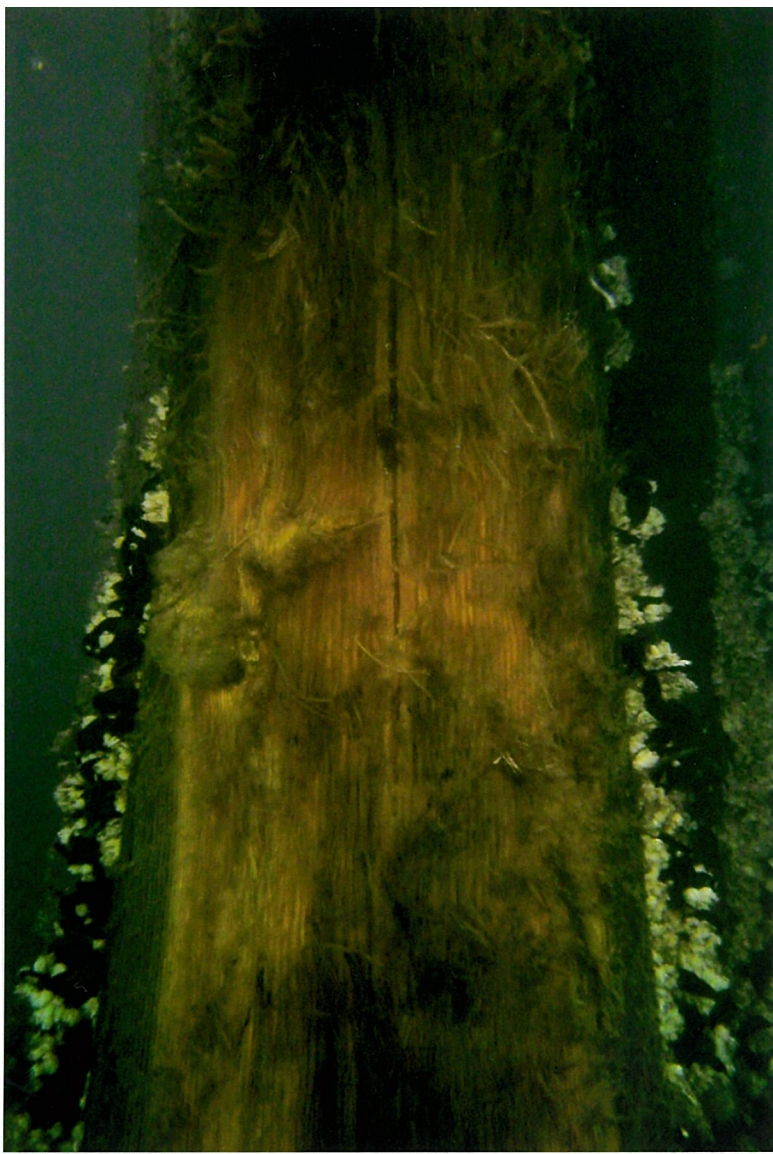
EXTENSIVE RUB WEAR OBSERVED ON THE OUTER TIMBER PILE FENDERS FOR THE JETTY
