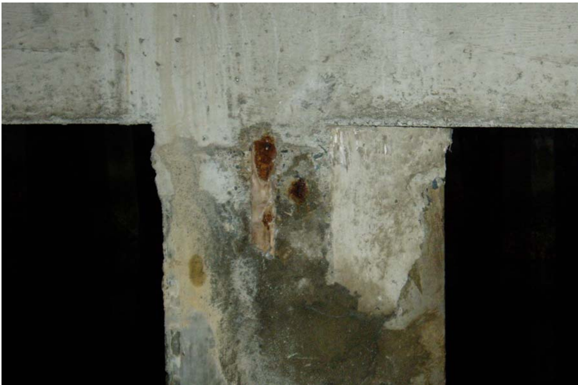
Photograph No. 9: Typical pile spall.
