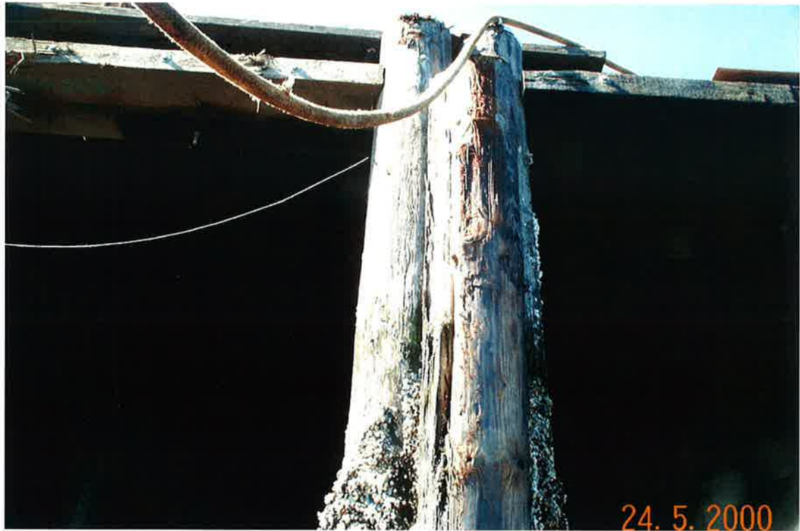
Photograph No. 9: Fungal decay and mechanical damage at the top of the rub pile.
