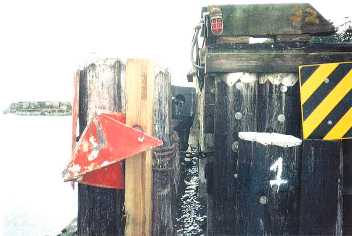
Photograph No. 3: Four Pile Cluster - Piles do not appear to be connected to the jetty.
