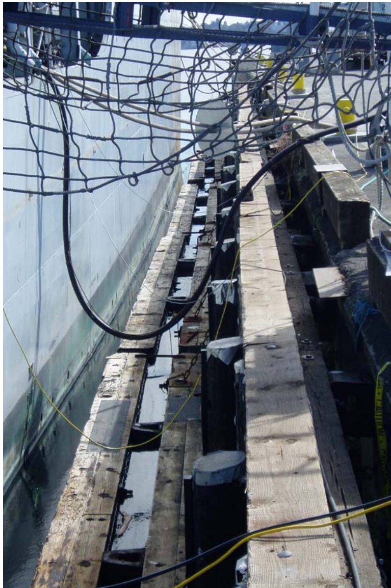
Photograph No. 4: Fendering on west berth face.
