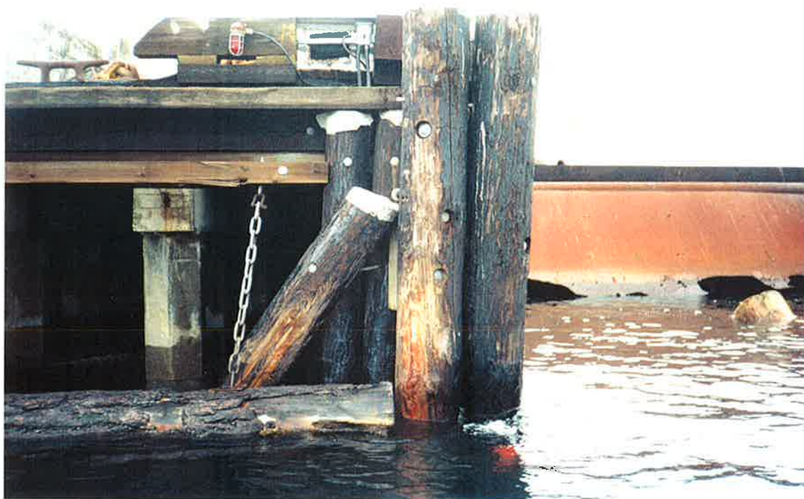
Photograph No. 1: Bent 19A, Rubbing Pole - Lower connection bolts are missing and Pile is loose.
