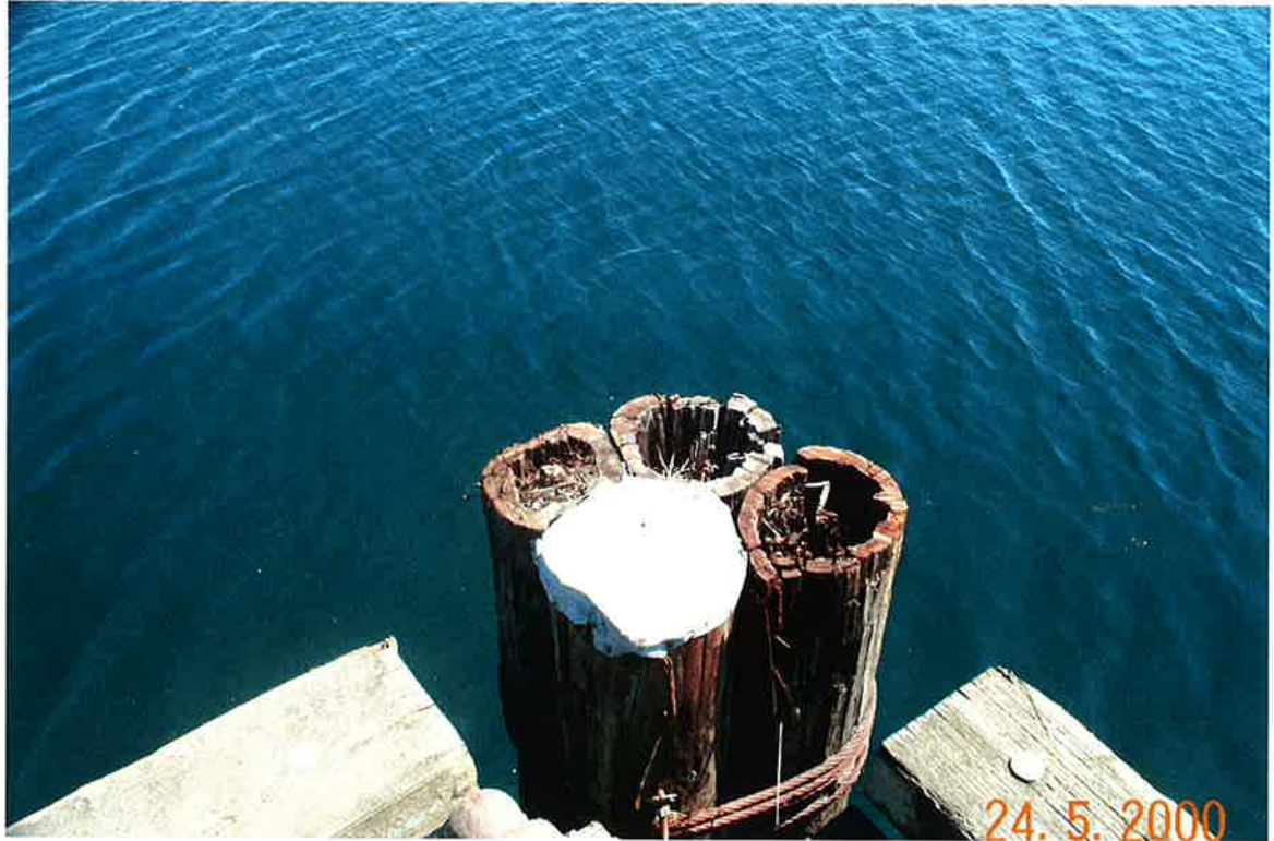
Photograph No. 13: Fungal decay in the tops of the 4-pile mooring dolphin at the northeast corner of the facility.
