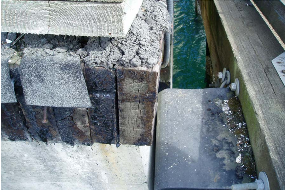
Photograph No. 6: Laminated deck damage in north-east corner.
