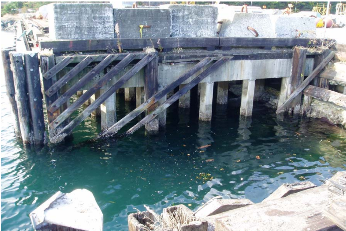
Photograph No. 11: Disused ramp area with missing debris guards.
