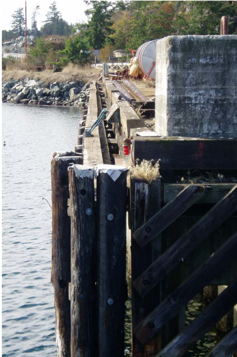
Photograph No. 5: Fender piles on north berth face.
