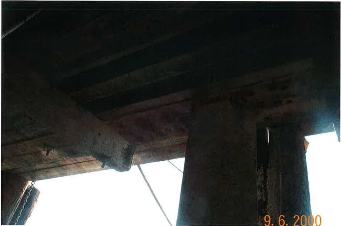
Photograph No. 3: Exposed, rusted reinforcing steel along Bent No. 1, between Piles A and B.
