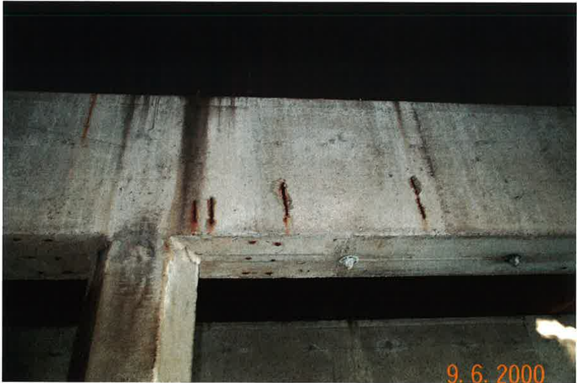
Photograph No. 5: Exposed, rusted reinforcement at Pile No. 24C.
