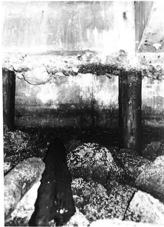
View facing service tunnel at bents 8/9 showing exposed piles and tunnel and crack in tunnel at construction joint.
