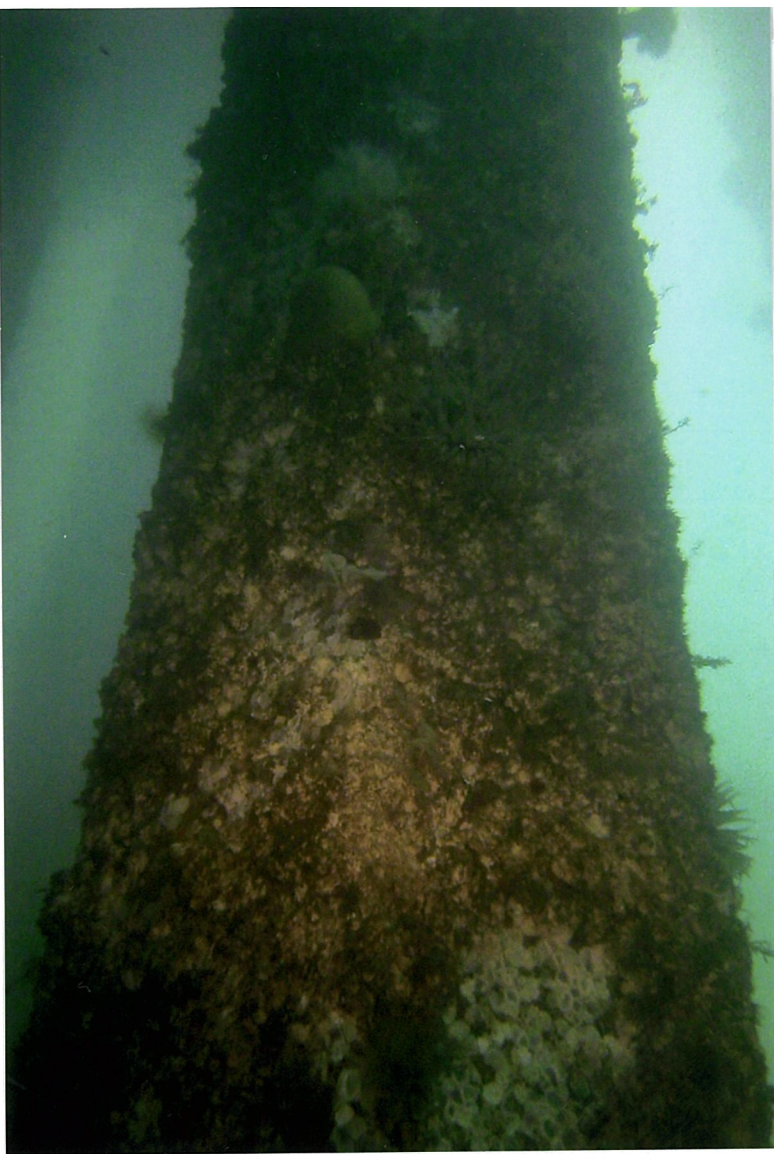
GENERAL EXTENT OF MARINE GROWTH AND CONDITION VIEW OF CONCRETE OCTAGONAL PILES
