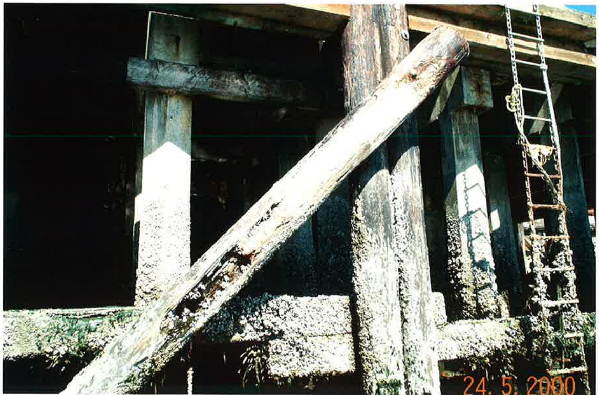
Photograph No. 8: Rub pile has severe marine borer infestation, and as a result the lower connection has failed.
