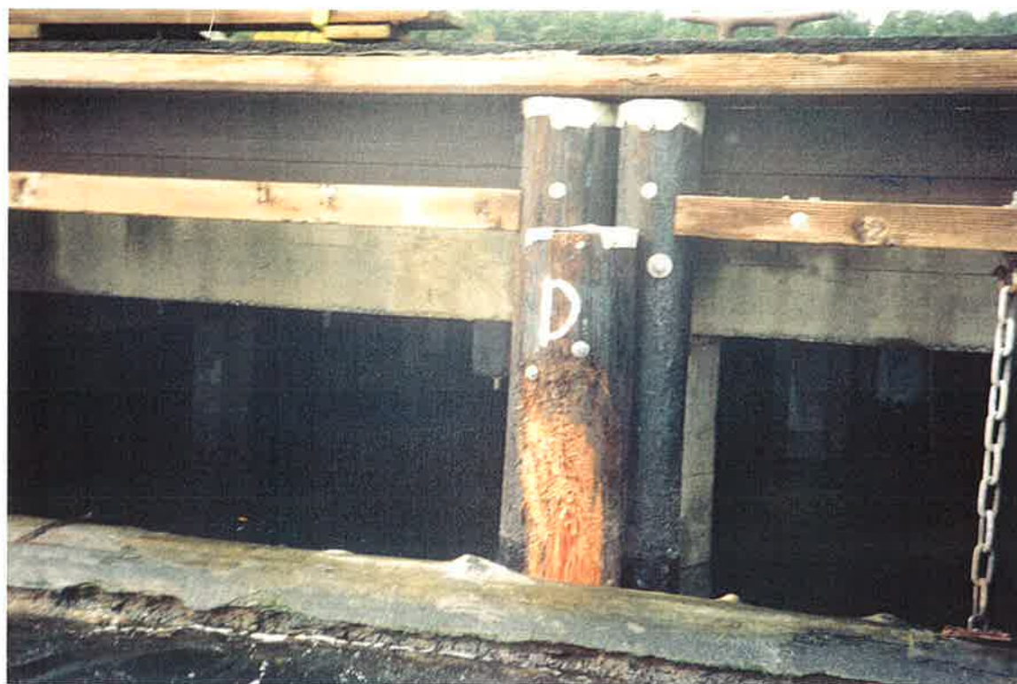
Photograph No. 2: Bent D, Rubbing Pole - 50% CSL in intertidal zone due to abrasion.
