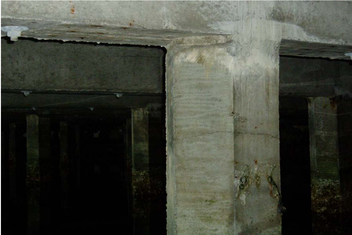
Photograph No. 10: Typical previous repairs to pile/pilecap interface.
