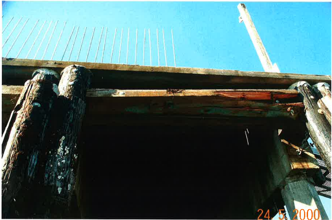
Photograph No. 15: Chock No. 37-38 is fractured.
