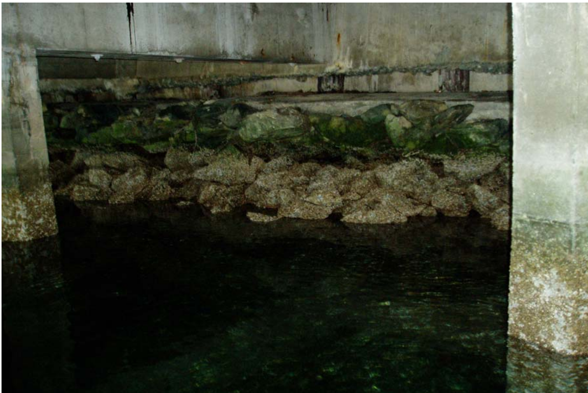
Photograph No. 7: Abutment undermining.
