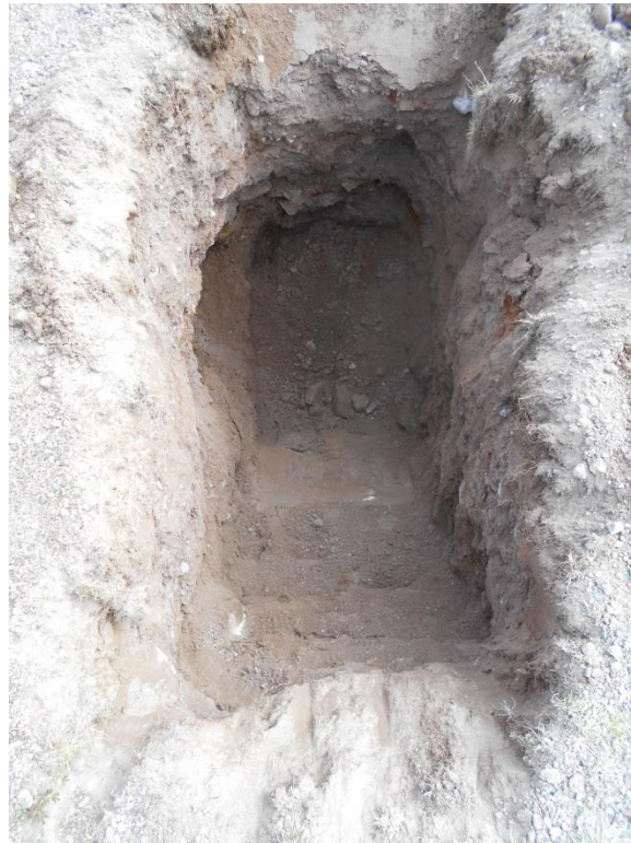
Test Pit TP-13
