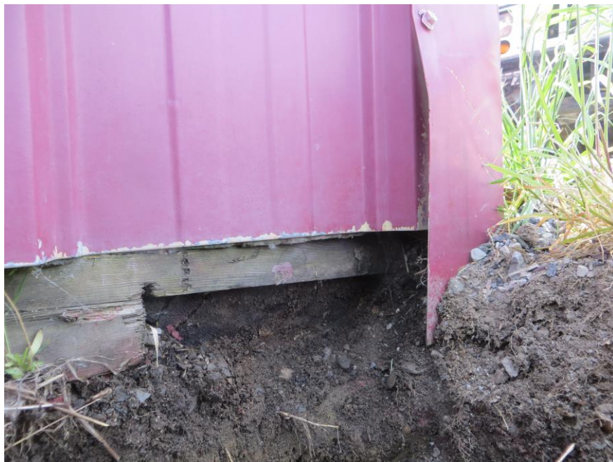
Photo 16: View of existing timber sill plate.
