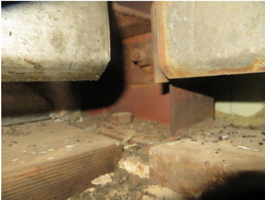
Photo 15: Typical baseplate at corner column.
