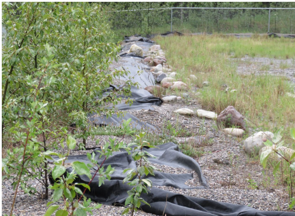
Photograph 6: View of typical berm construction at STF. Exposed liner on berm is woven material, and may extend below STF.
