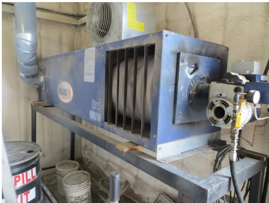
Photo 11: View of used oil unit heater.
