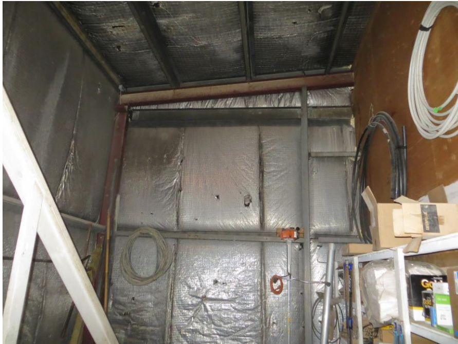
Photo 13: View of secondary framing on north wall (upper).
