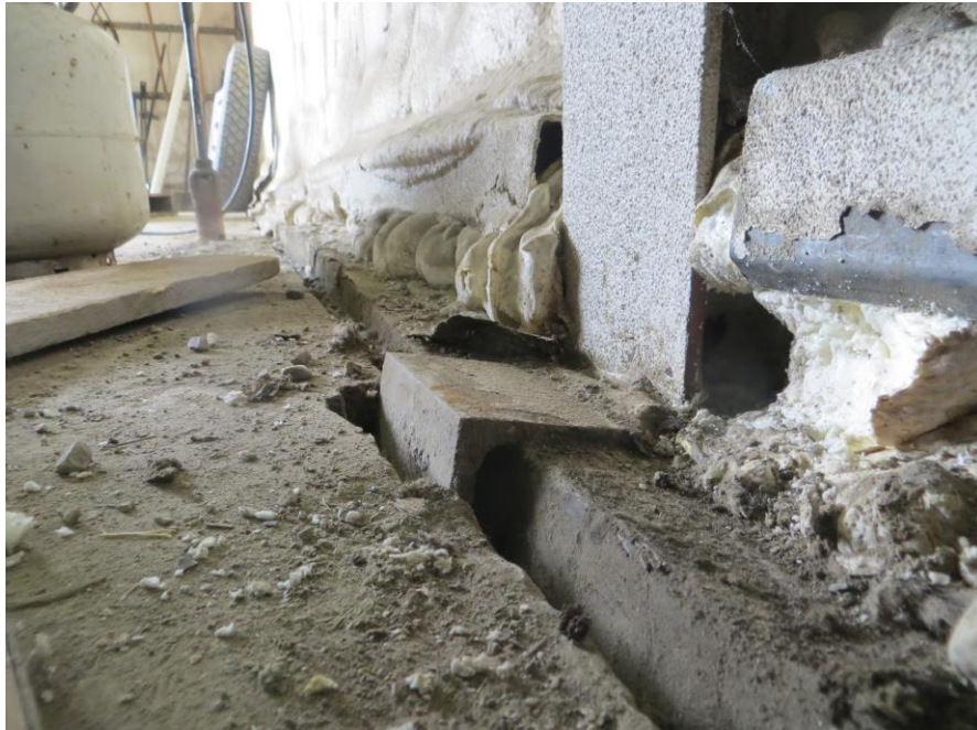
Photo 17: View of existing base plate of portal frame.
