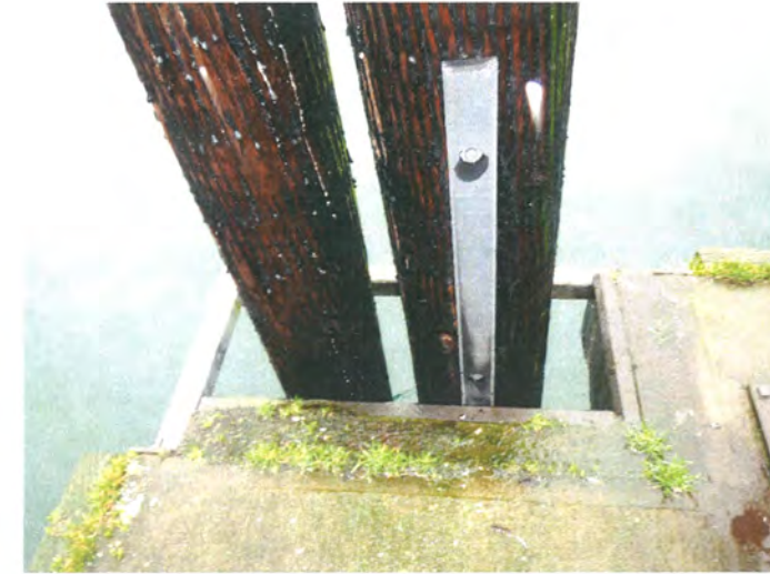
3. TIMBER LOCATOR PILES AND MOORING BRACKET
