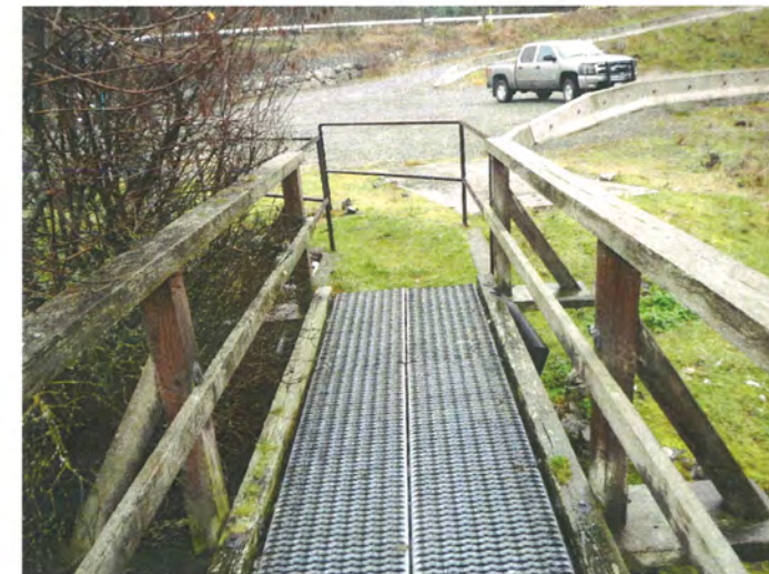
9. SHOREWARD END OF TIMBER APPROACH STRUCTURE
