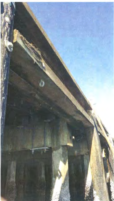
13. UNDERSIDE OF JETTY STRUCTURE AND TIMBER CHOCKS
