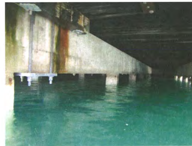
8. CONCRETE/TIMBER JETTY DECK STRUCTURE
