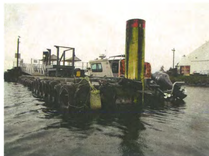
7. D JETTY FLOAT AT WEST END OF NORTH BERTH
