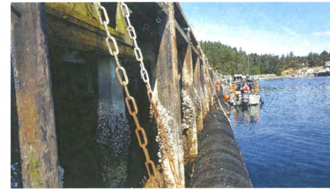
6. VIEW LOOKING WEST ALONG THE NORTH BERTH
