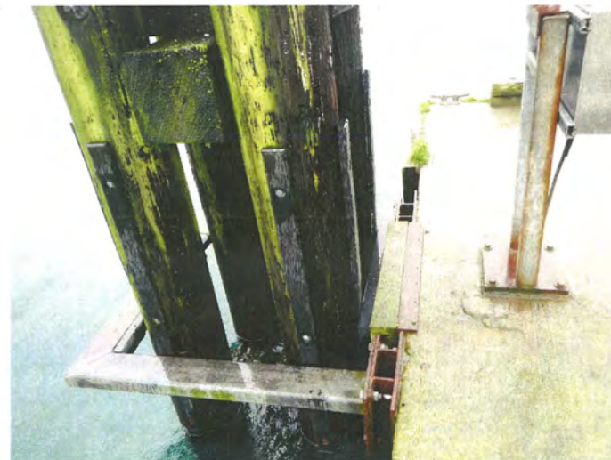
8. SEAWARD LOCATOR PILE GROUP AND MOORING BRACKET
