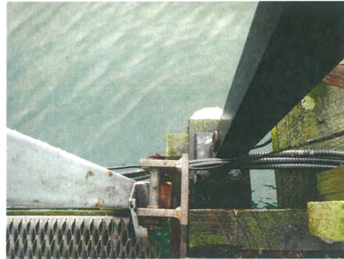
2. PINNED HINGE AT TIMBER PILED BENT
