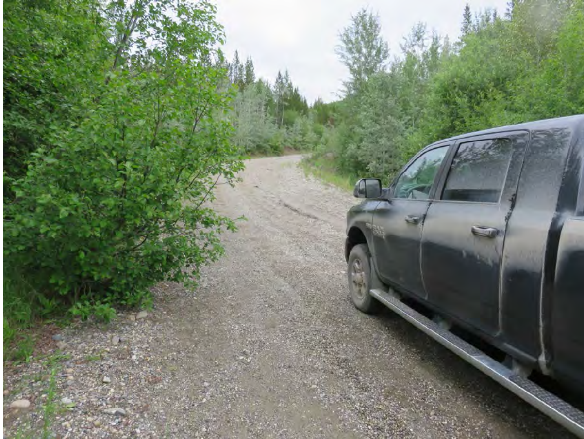
Photograph 1: View looking northeast at access road from near its junction with Highway 97. Note steep gradients ranging between approximately 10% to 15%.
