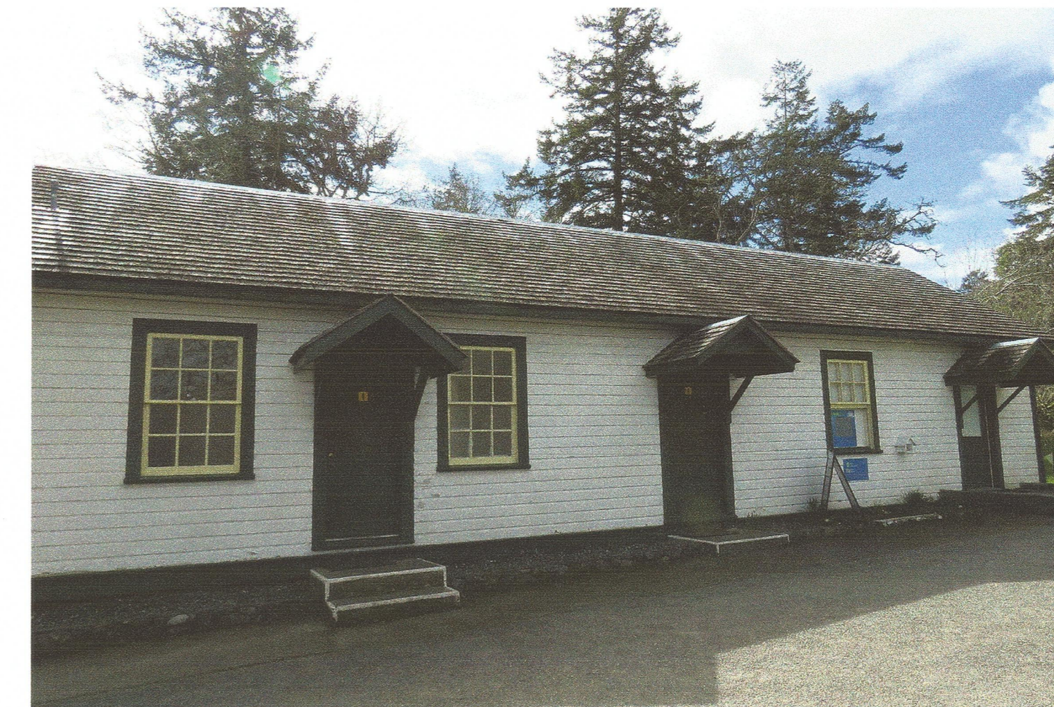
5. WW2 HUT (WASHROOM BUILDING)
