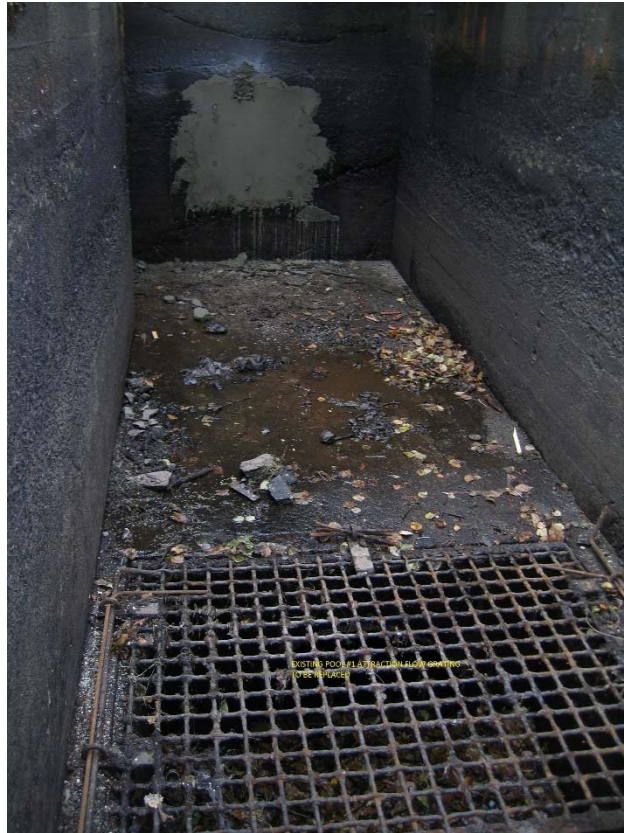
Attraction flow floor grating in Pool #1
