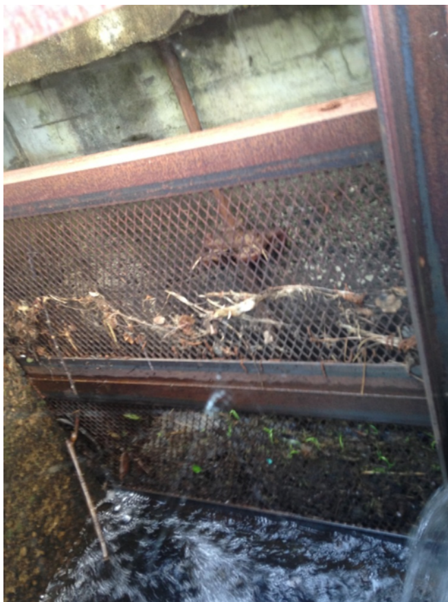
2015 – Debris on screen in Pool No. 6
