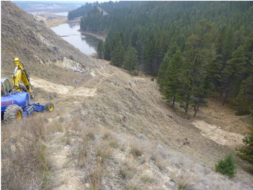
Photo 39: Re-contouring of disturbed test pit locations (TP8-11 and cavity assessment).
