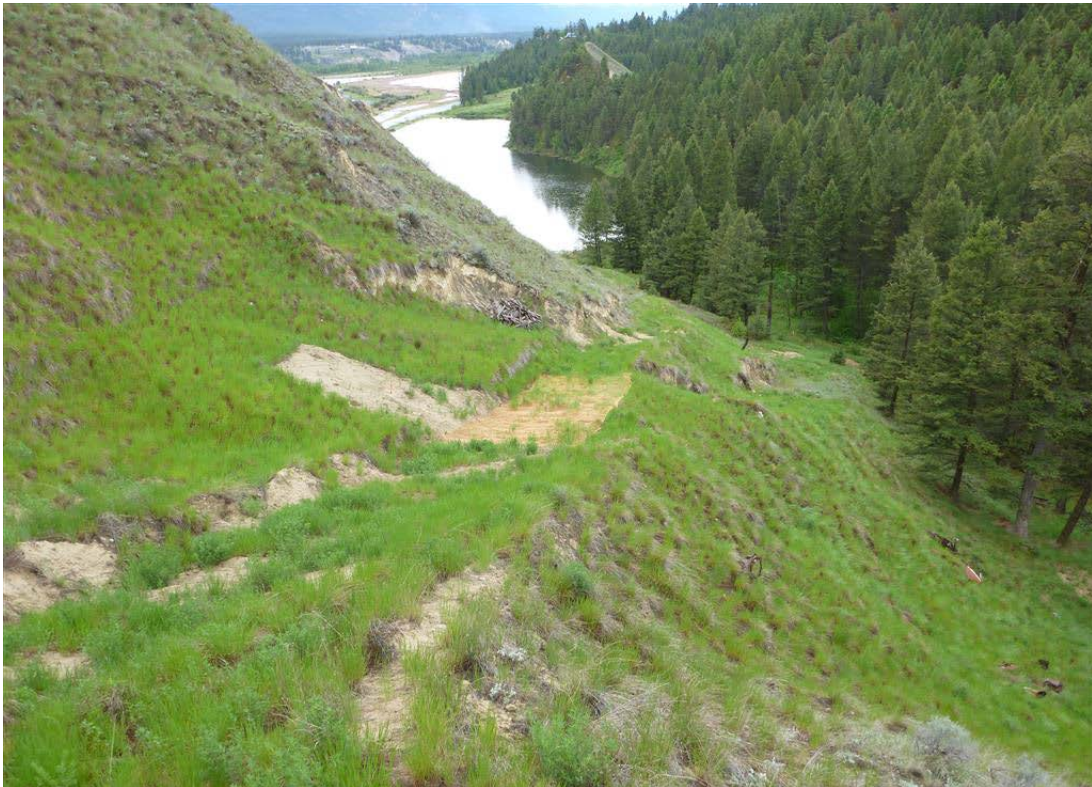
Photo 11: Area previously installed with coir material in April 2014 noted as stable.
