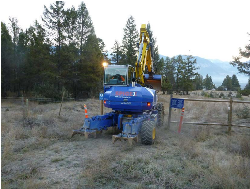
Photo 1: Fence opened to allow for access of SPIDEX excavator.
