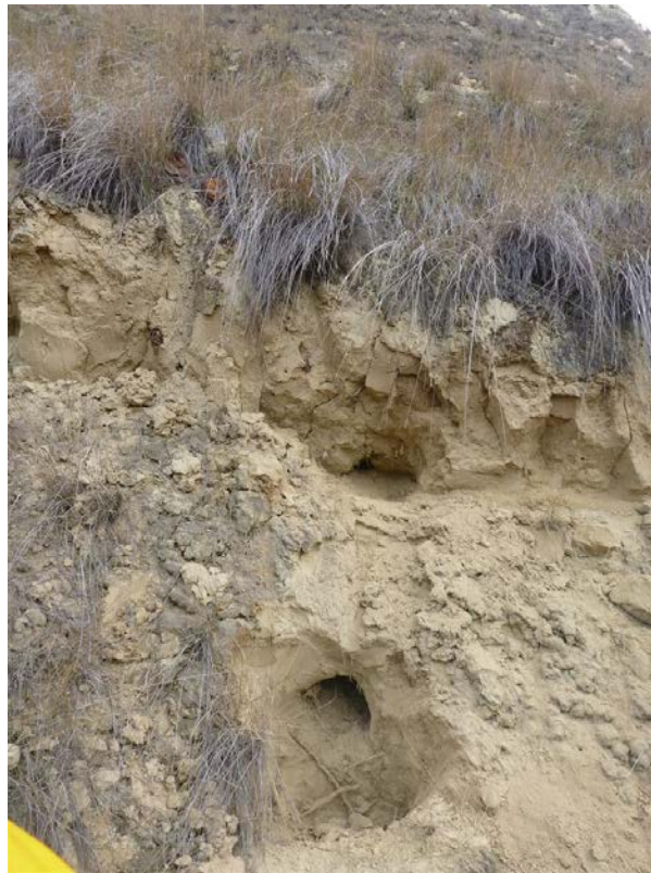
Photo 26: Located exit of cavity to south of trail flowing downslope .
