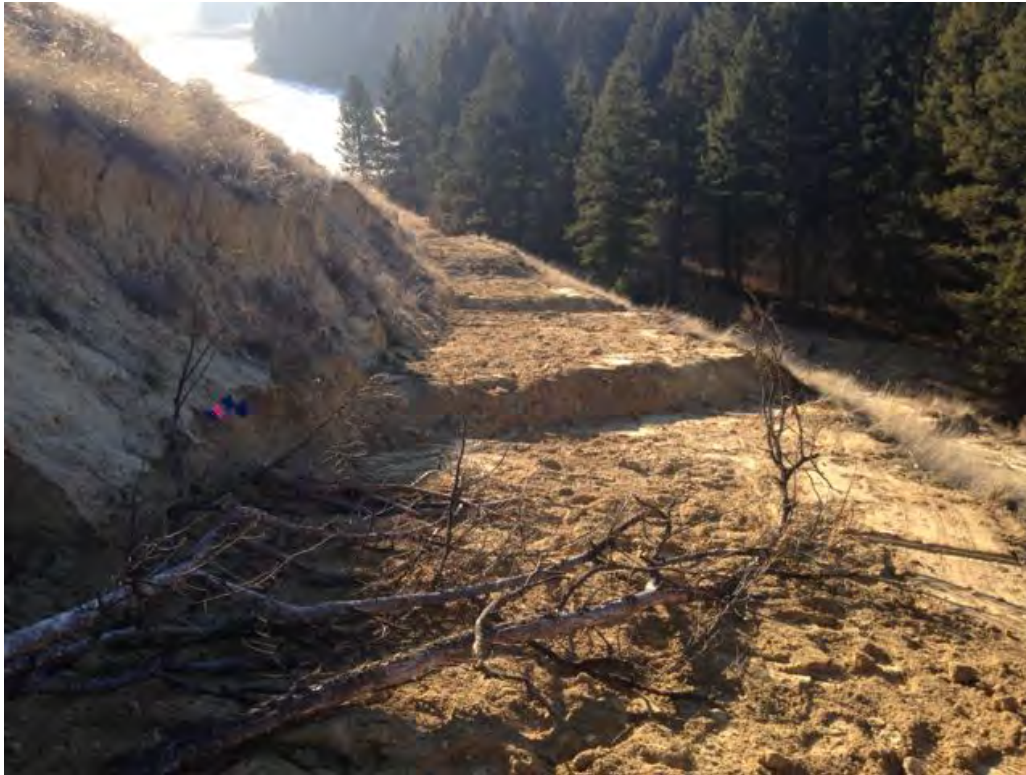
Photo 7: View of cross-ditches and regarding of lower trail (Feb. 24, 2015)
