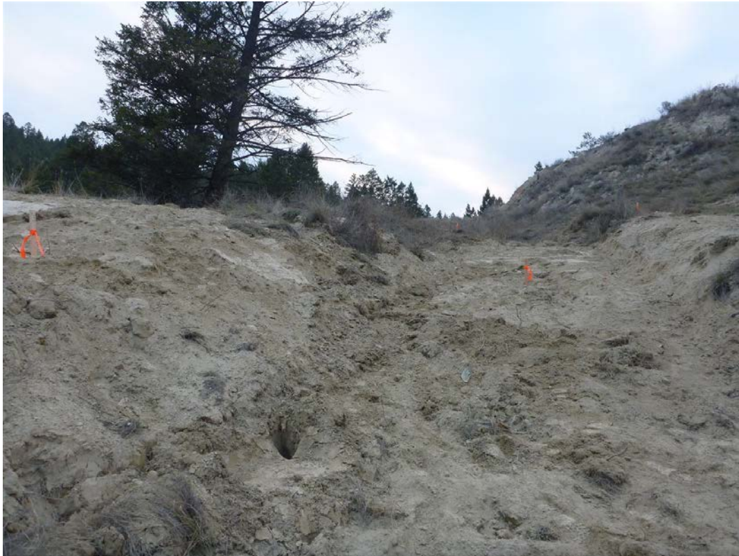
Photo 40: Following re-contouring, flagging of test pits was conducted.
