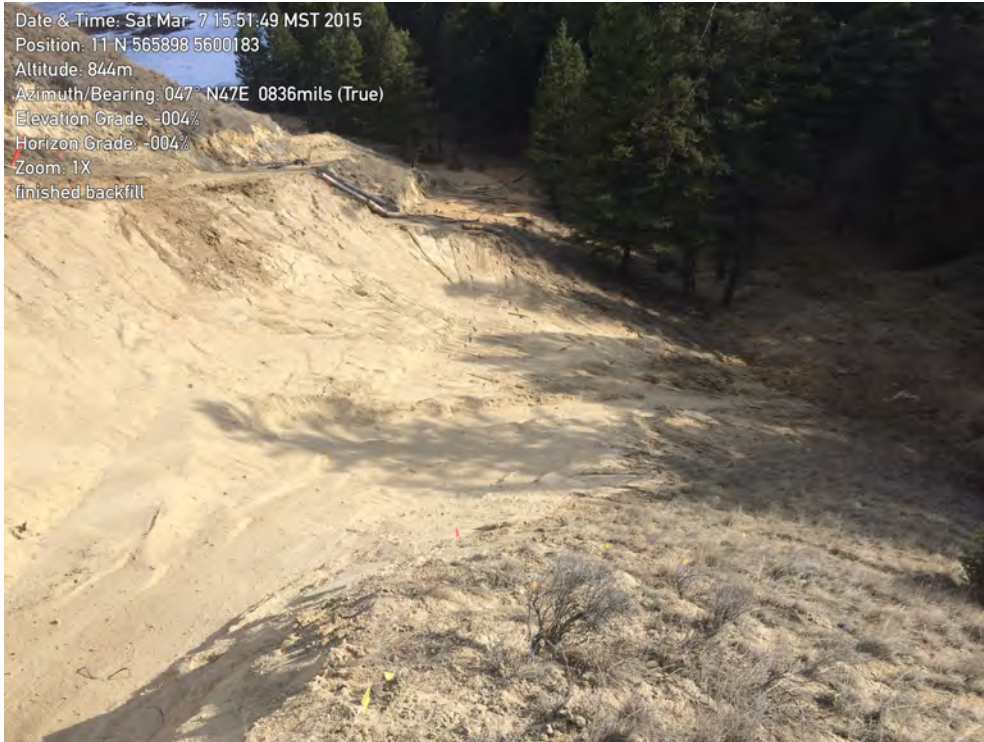
Photo 5: View of completed backfill within the MDZ (Mar. 7, 2015)
