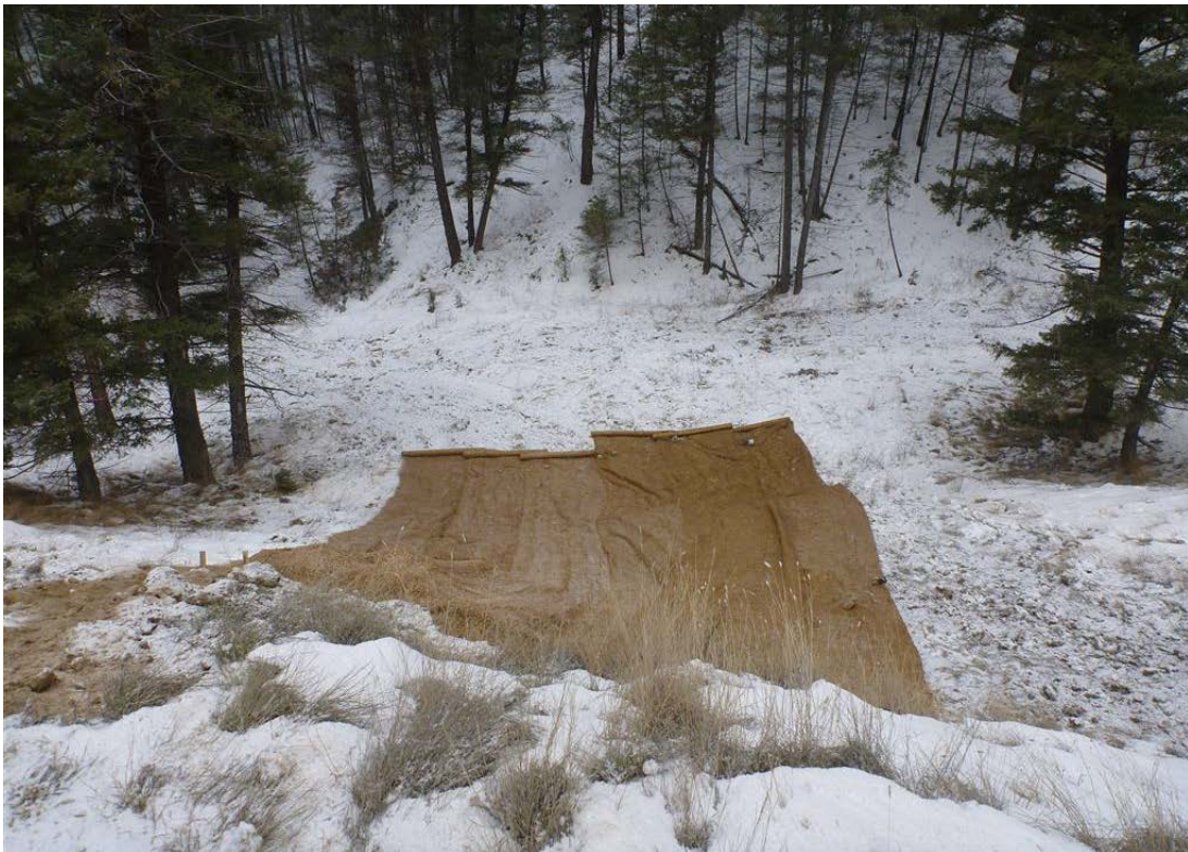
Photo 74: Temporary photodegradable blankets placed along south slope for erosion control.
