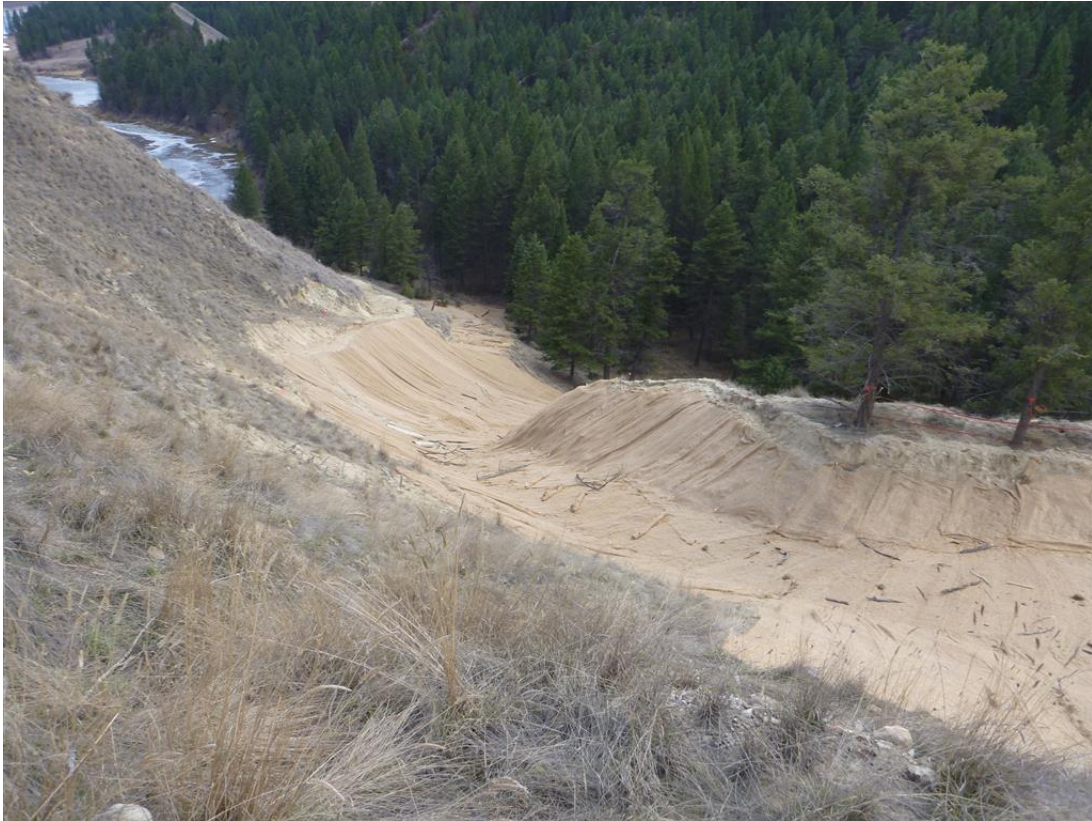
Photo 101: View of restored excavation area (looking east).
