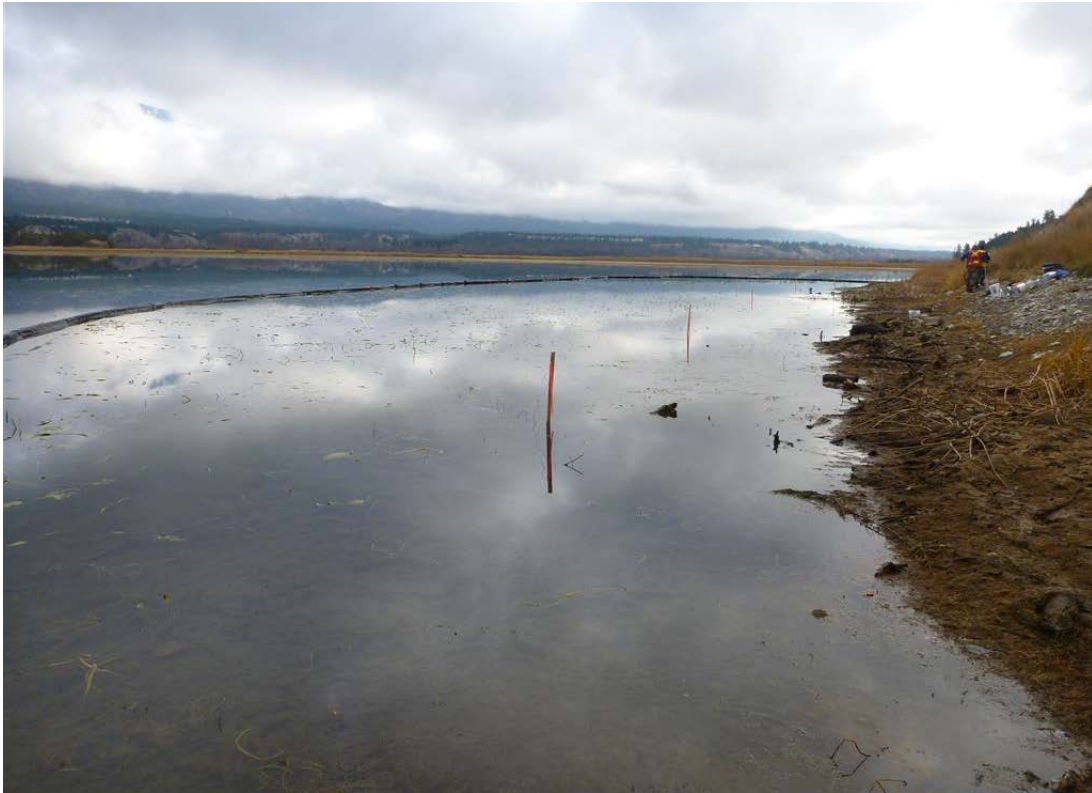
Photo 47: Minnow traps established and anchored with orange-flagged stakes along the inside of the isolation curtain and along the shoreline.
