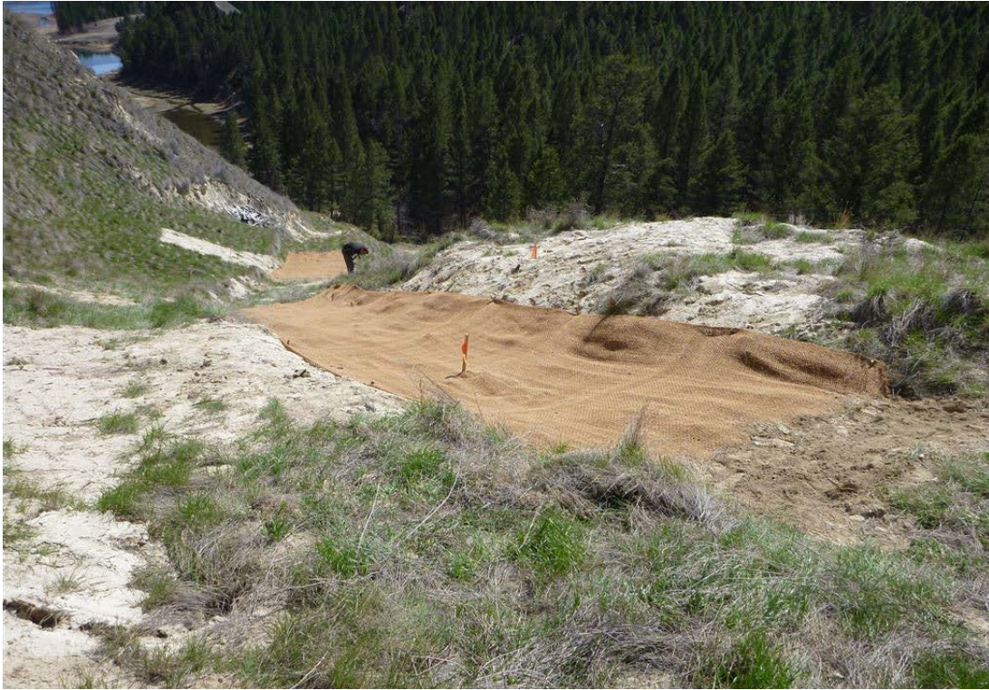
Photo 7: Looking east along trail at coir installation.
