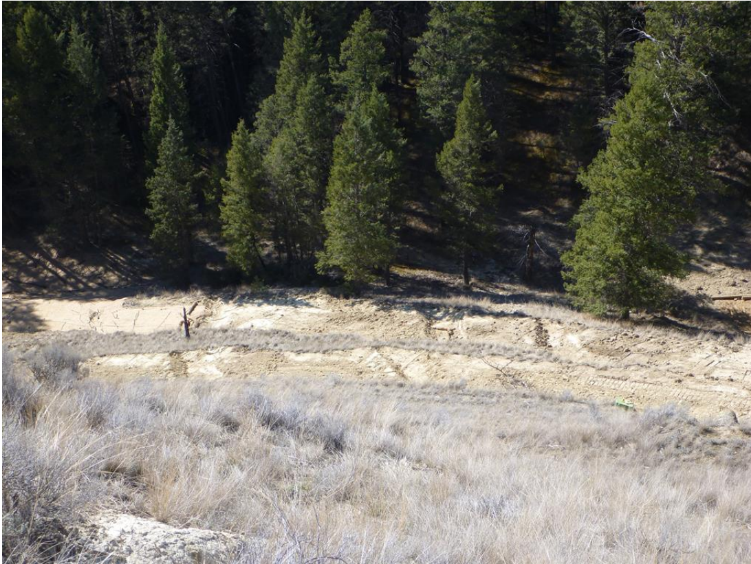
Photo 93: Cross ditches on upper and lower trails.
