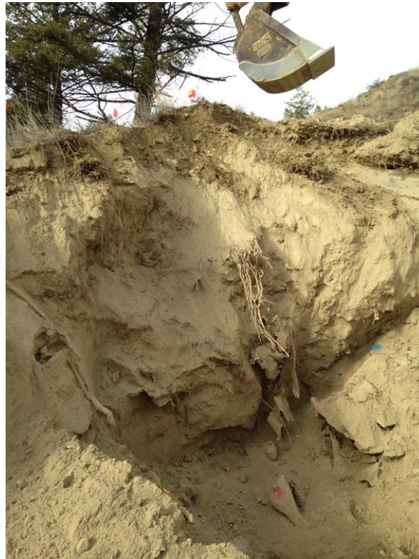
Photo 81: Excavation in MDZ at west end adjacent to existing trees.
