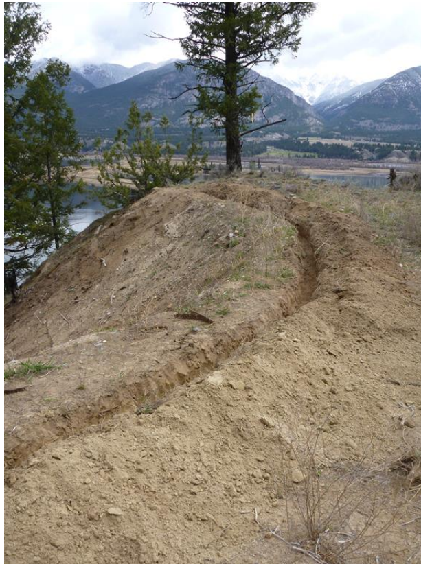
Photo 4: Trench cut at the top of the gully to key in coir.
