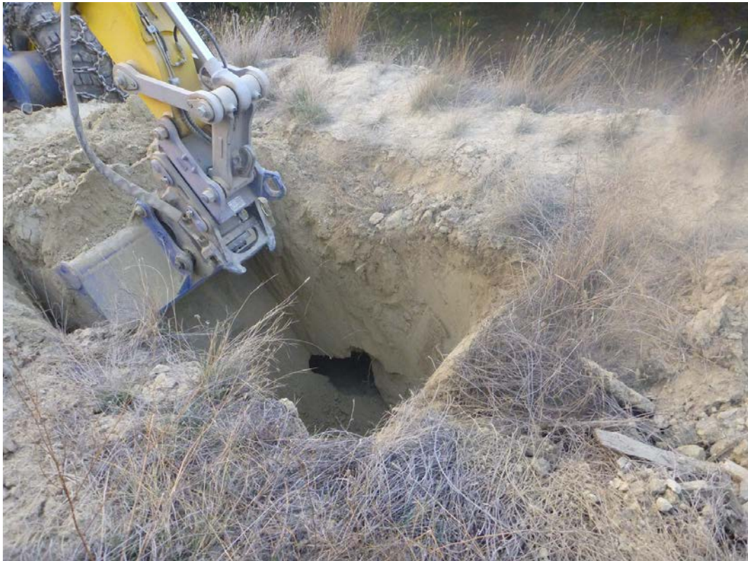
Photo 25: Excavation in area of cavity and water flow – found deep cavity in trail.
