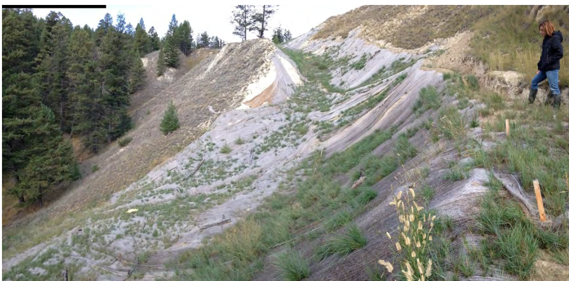
Photo 2: View of the Main Debris Zone to the west from the bottom of the slope. Note panels of fabric on the south side of the slope that have been wind blown (Sept. 21, 2015)
