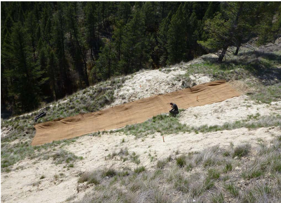
Photo 6: Installation of coir at test pits along trail.
