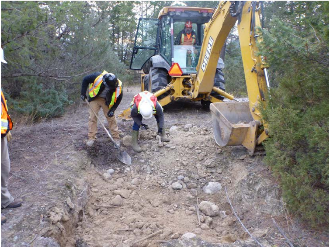
Photo 41: Site cleanup in 2011 - 0565811E 5600294N
