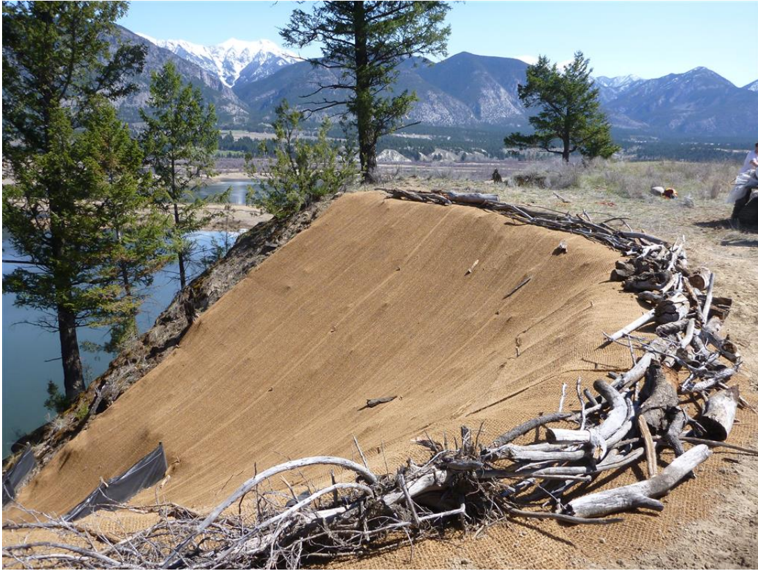
Photo 5: Coir installed at gully with woody debris around the top for stability.
