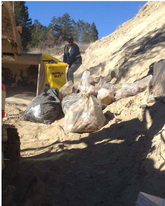
Photo 86: Fuel soaked absorbent pads collected in plastic bags and removed for disposal.
