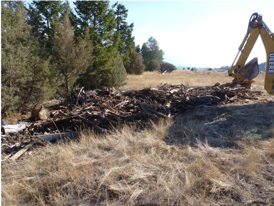
Photo 45: Site cleanup in 2011 - 0565018E 5601261N
