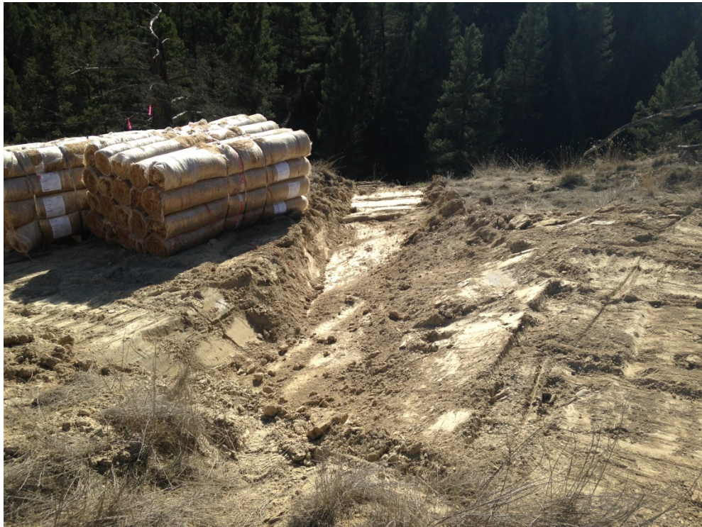
Photo 89: Permanent diversion ditches installed along trail.
