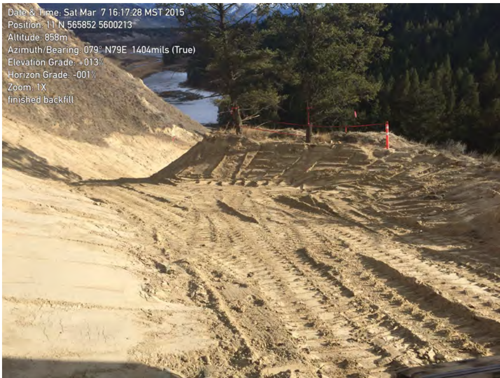
Photo 6: View of completed backfill in the area behind the trees (Mar. 7, 2015)
