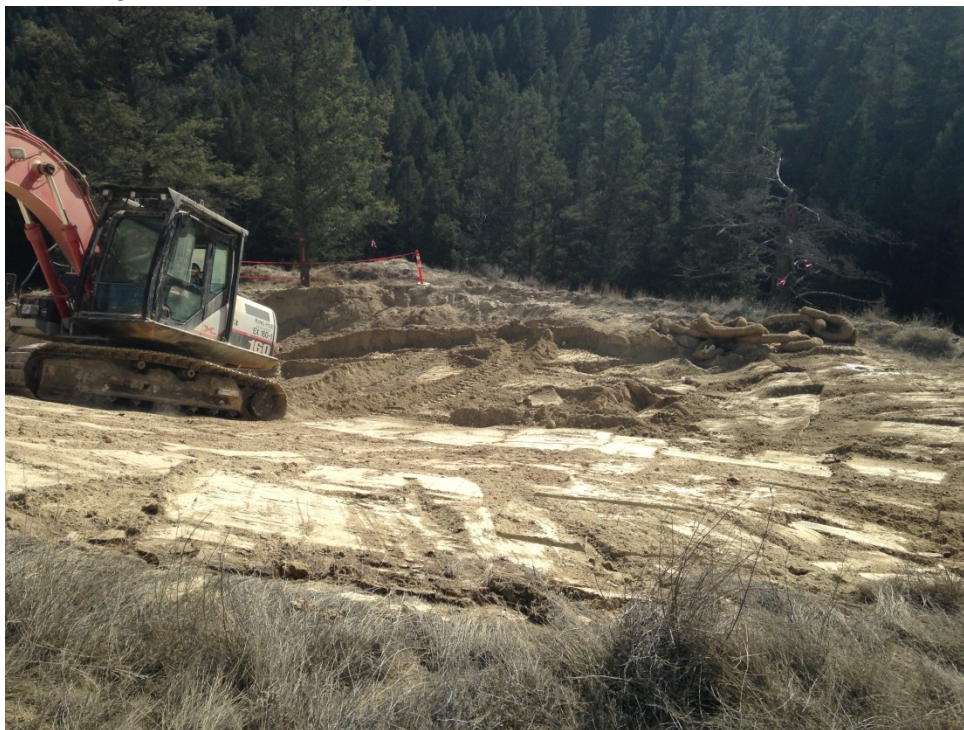
Photo 88: Excavation of fill material on north side of trees used for stabilization.
