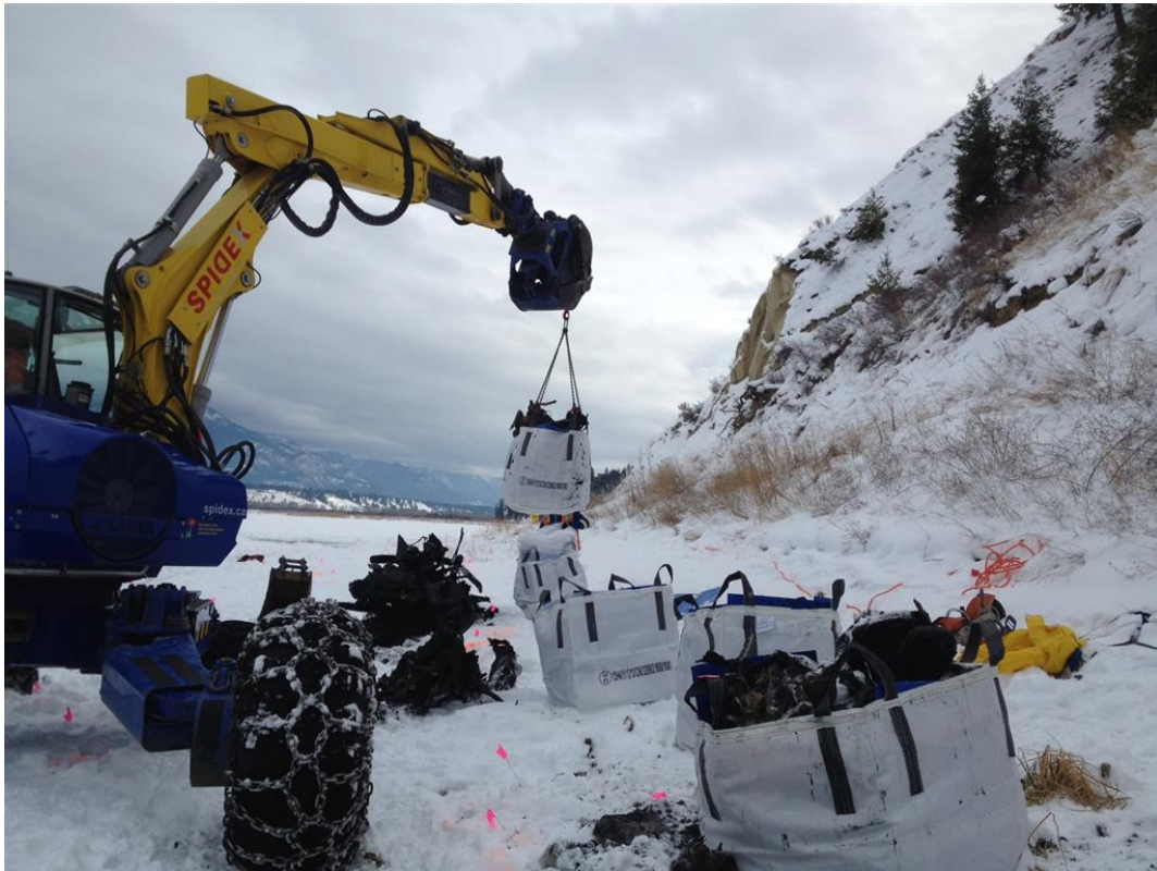
Photo 61: Material from shoreline and under ice collected in bags and bins.
