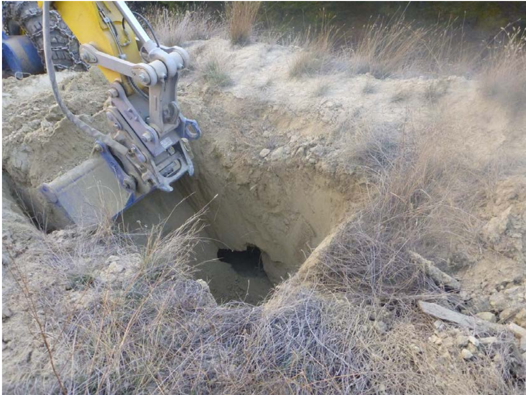
Photo 9: Excavation in area of cavity/void in lower portion of trail (Fall 2013).
