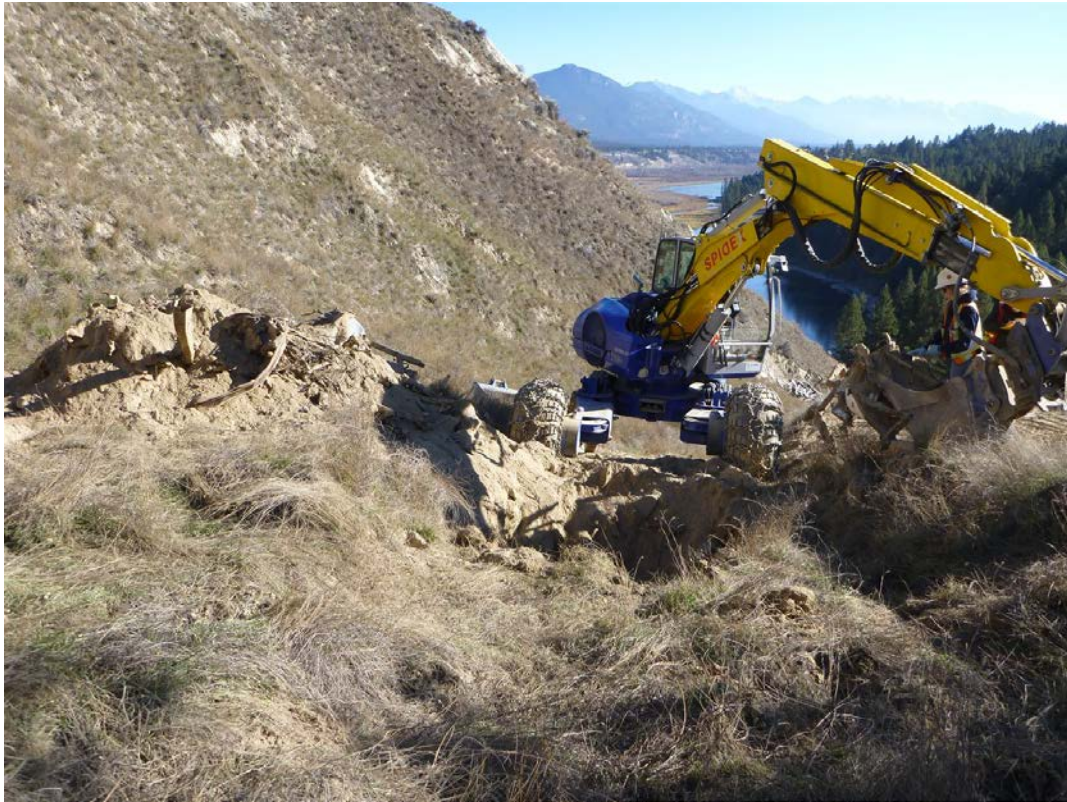
Photo 5: View of TP7 in Main Debris Zone (Fall 2013).
