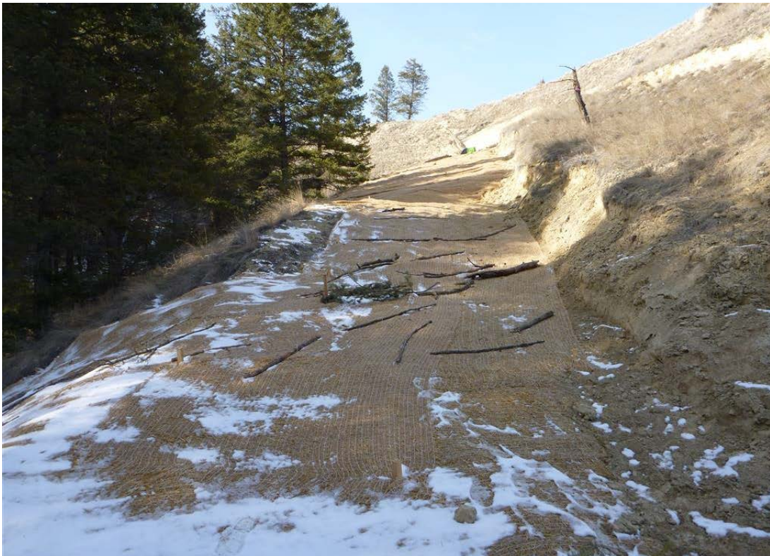
Photo 94: Lower trail erosion control blanket installation completed.
