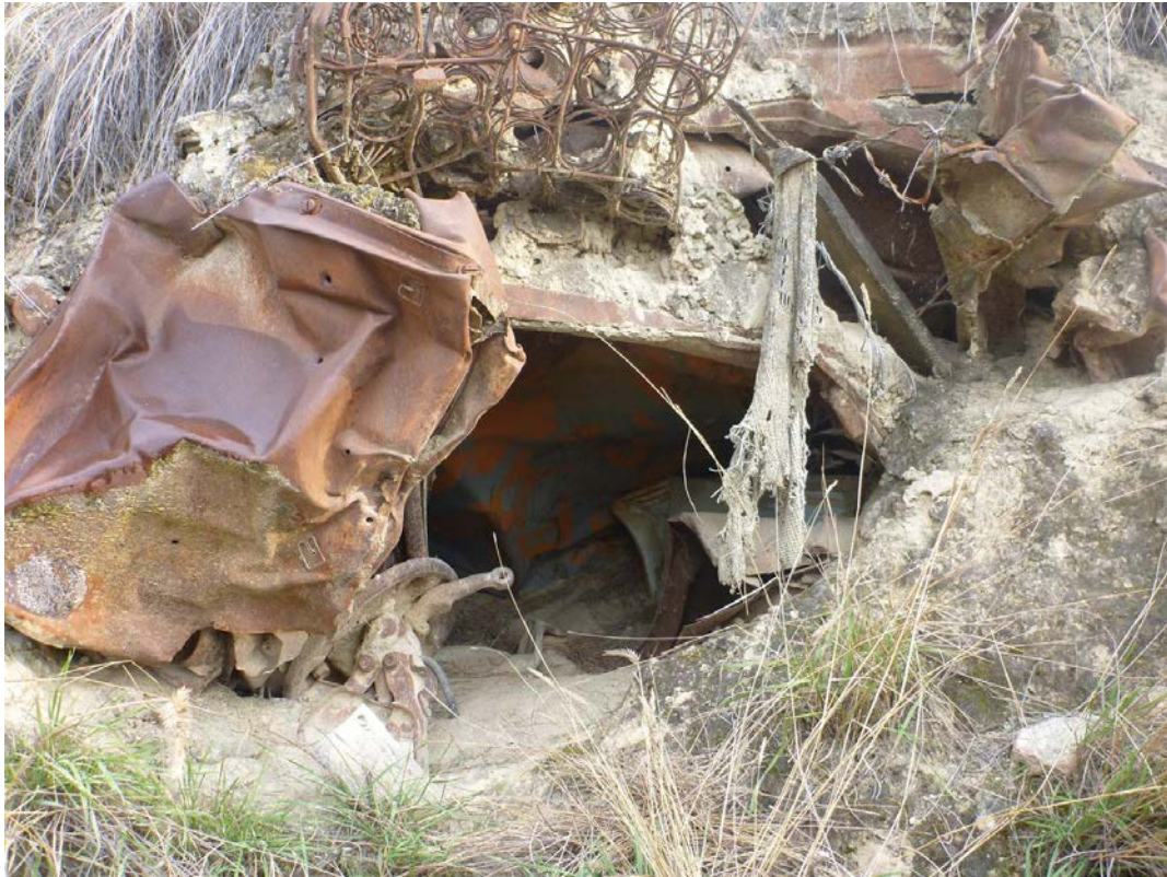
Photo 34: TP12 – Embedded metal debris in slope observed to have been used by wildlife in the past.
