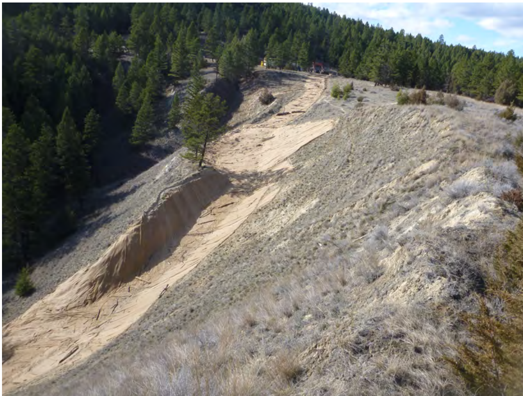
Photo 9: Final site completion showing ECB installation and CWD placement (Mar. 13, 2015)
