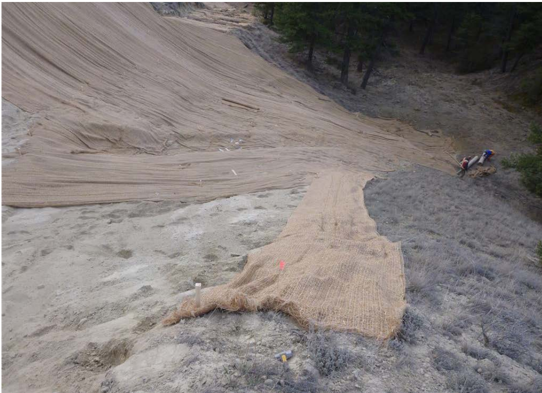
Photo 96: Installation of erosion control matting in the MDZ to lower slope.
