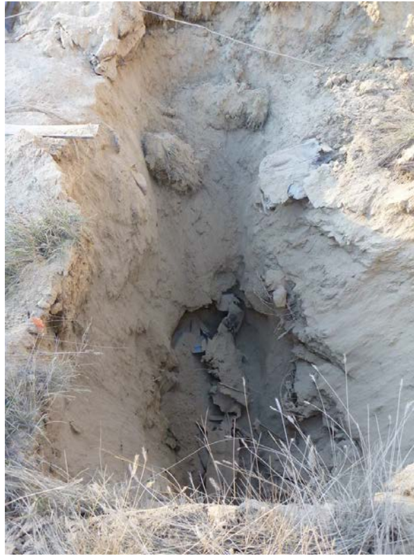
Photo 21: TP8 – Debris encountered to 4 m.
