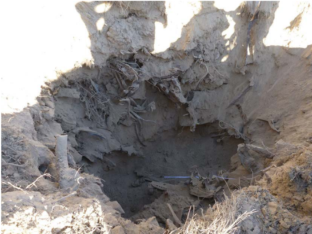
Photo 16: TP 7 - Metal debris still present in excavation at 4 m.
