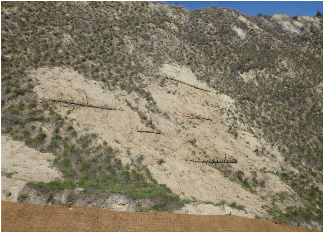
Photo 8: Test pits located on the north slope stabilized with woody debris.
