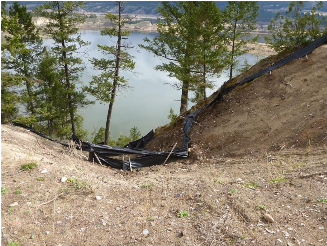
Photo 2: Silt fencing installed in 2012.
