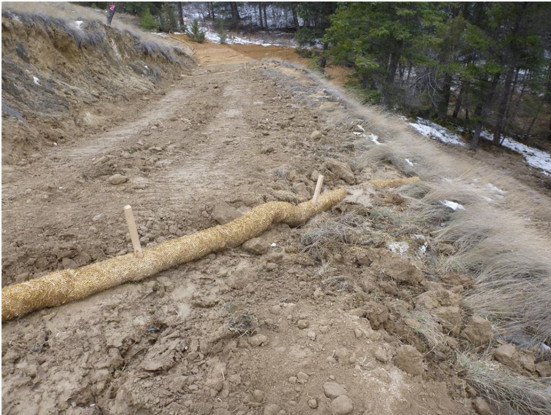
Photo 77: Temporary wattle installed at top of lower trail diverted rapid snowmelt water.
