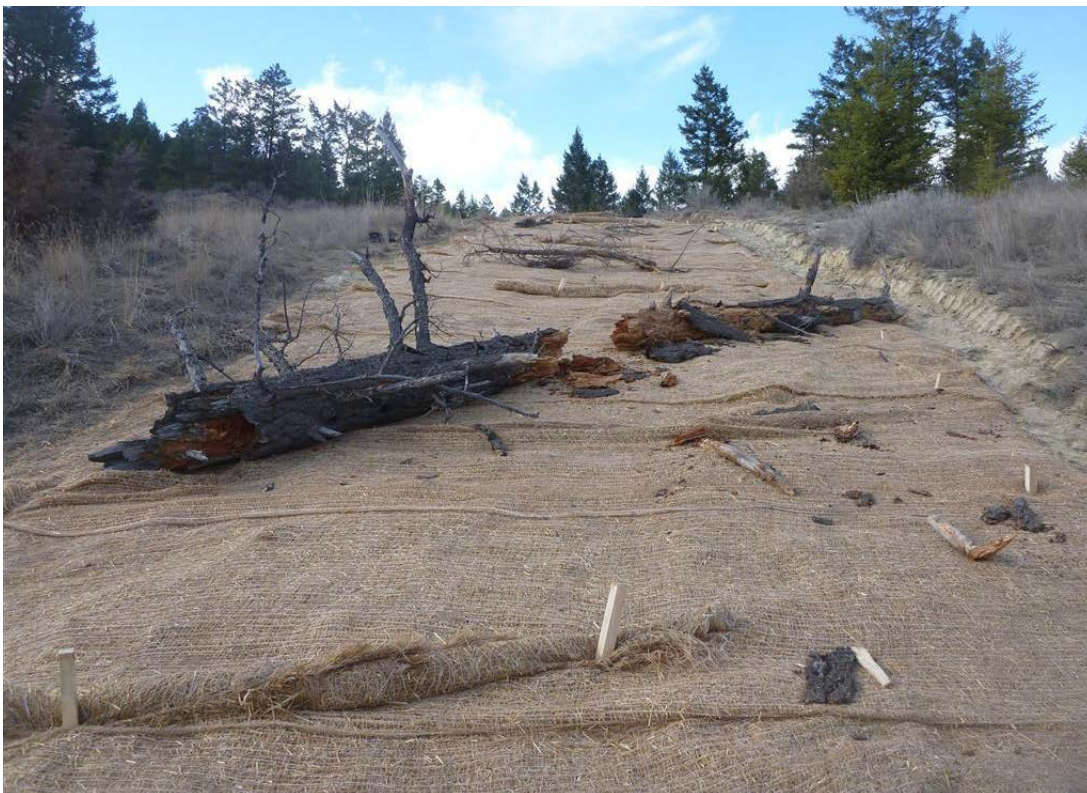
Photo 104: Woody debris and wattles installed along upper area of trail.
