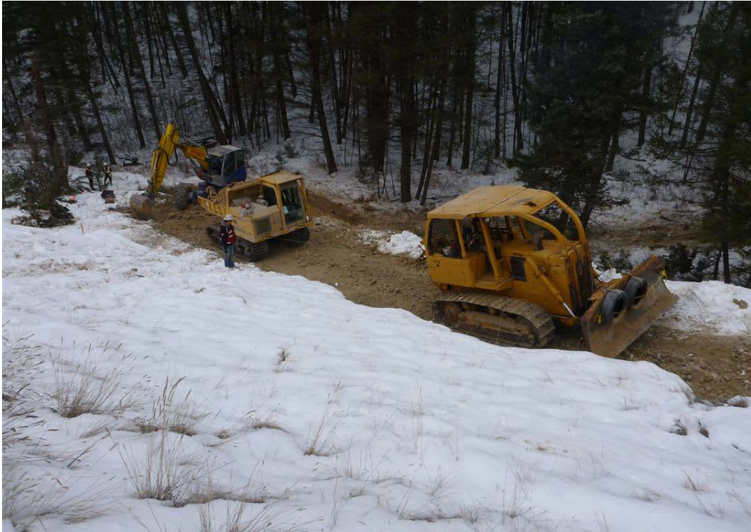
Photo 69: Winch system used to aid movement of morookas.
