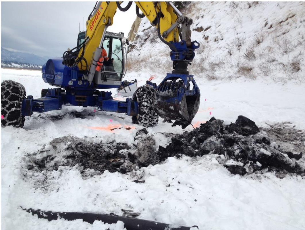
Photo 60: Shoreline debris removal using spider hoe.
