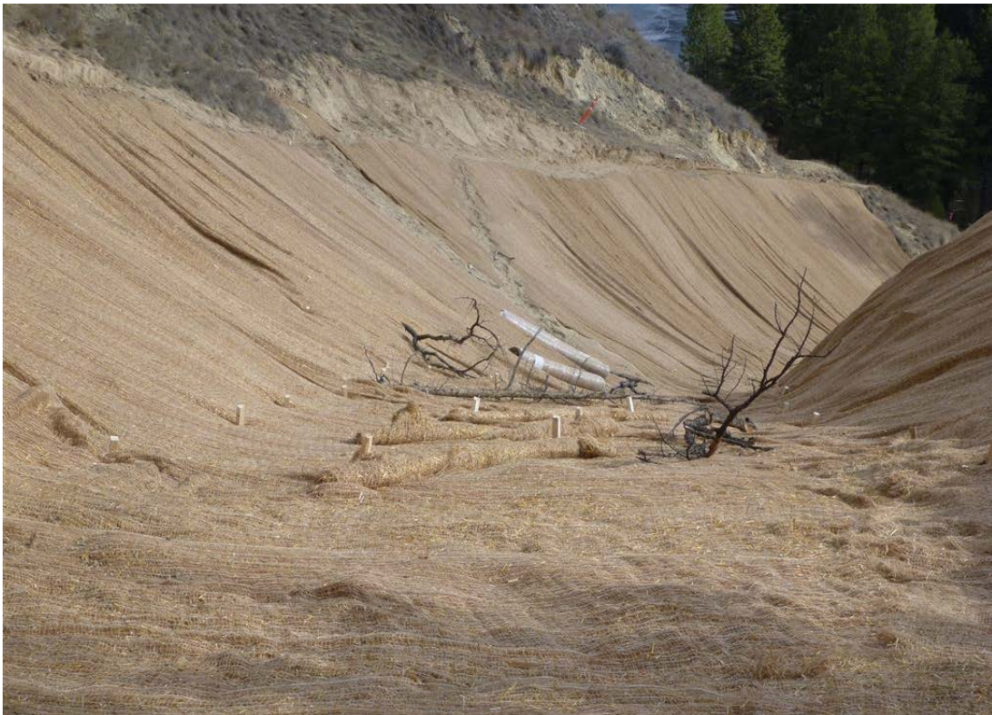
Photo 100: Wattles and woody debris installed along steeper portions of excavation area.
