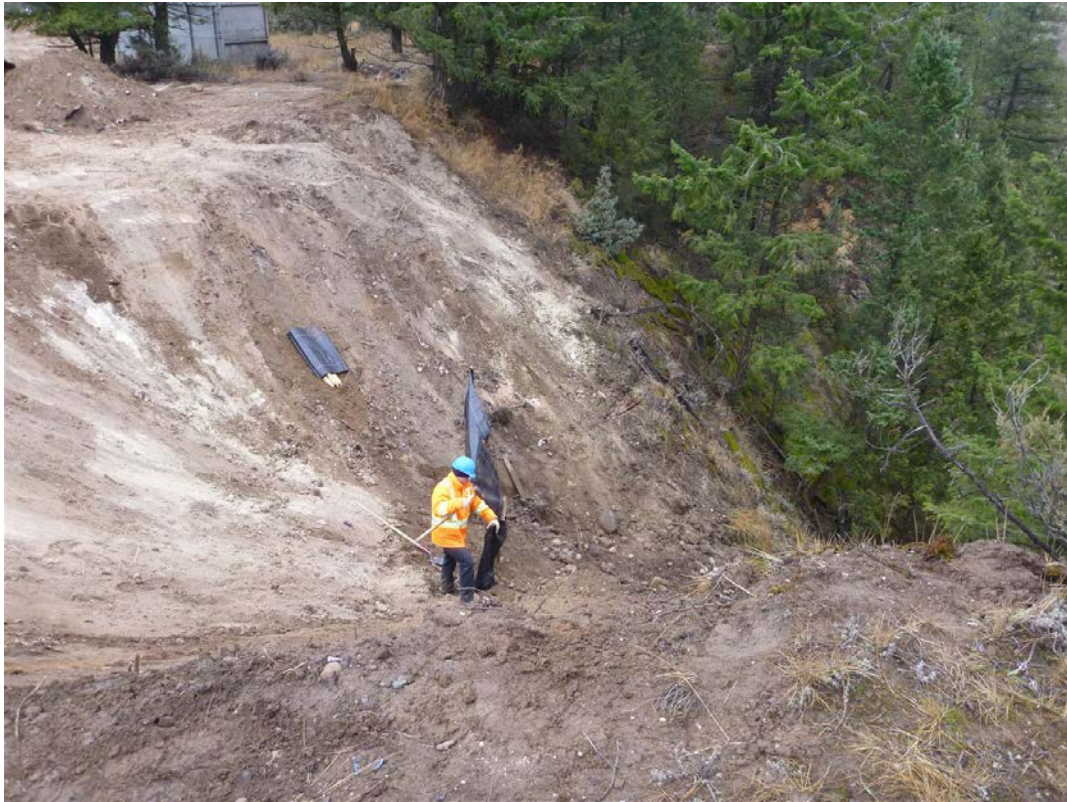
Photo 53: Large gully cleanup in 2012 - 0565971E 5600234N
