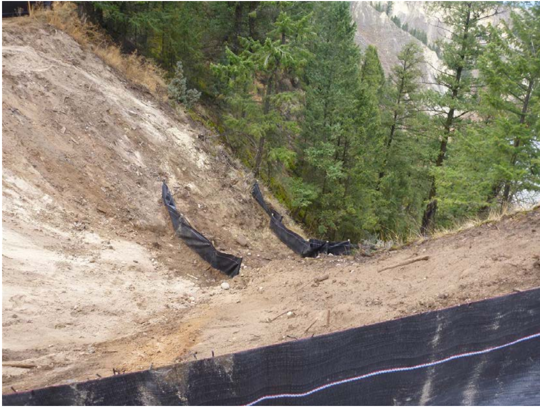
Photo 55: Large gully cleanup in 2012 - 0565971E 5600234N
