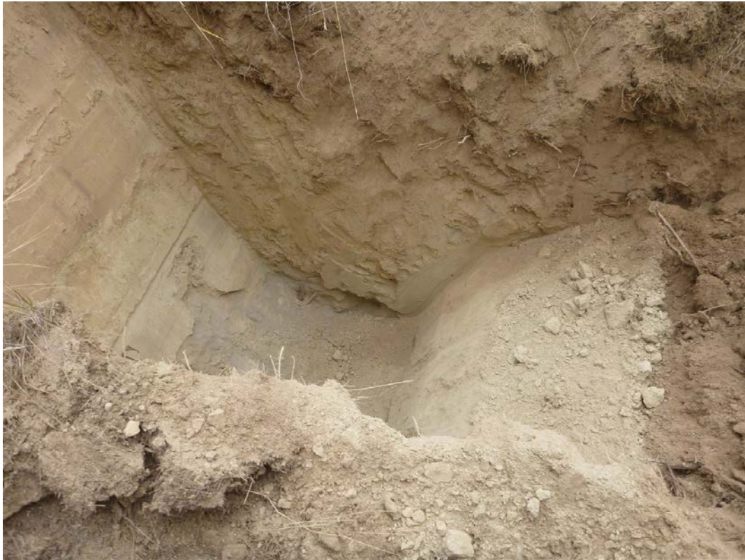
Photo 32: TP12 – Excavation revealed minimal debris.
