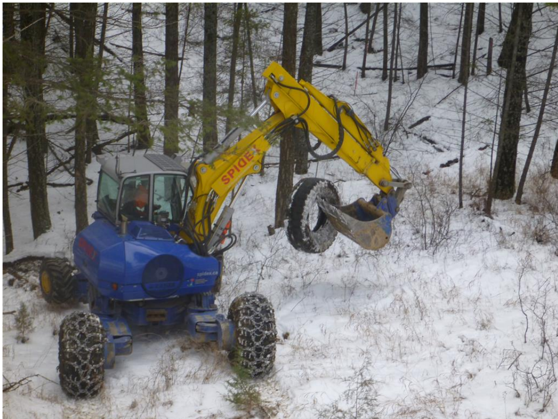
Photo 90: Debris removed from gully and other locations where possible.
