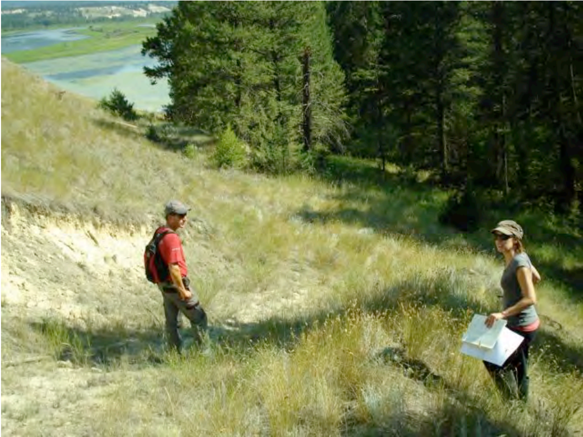
Photo 5: View downslope trail towards other area of test pitting. Note exposed soils along cutslope and erosion along surface of trail (in area of piping cavity).
