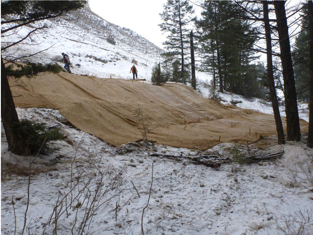
Photo 73: A13 temporarily matted with photodegradable erosion control blankets.
