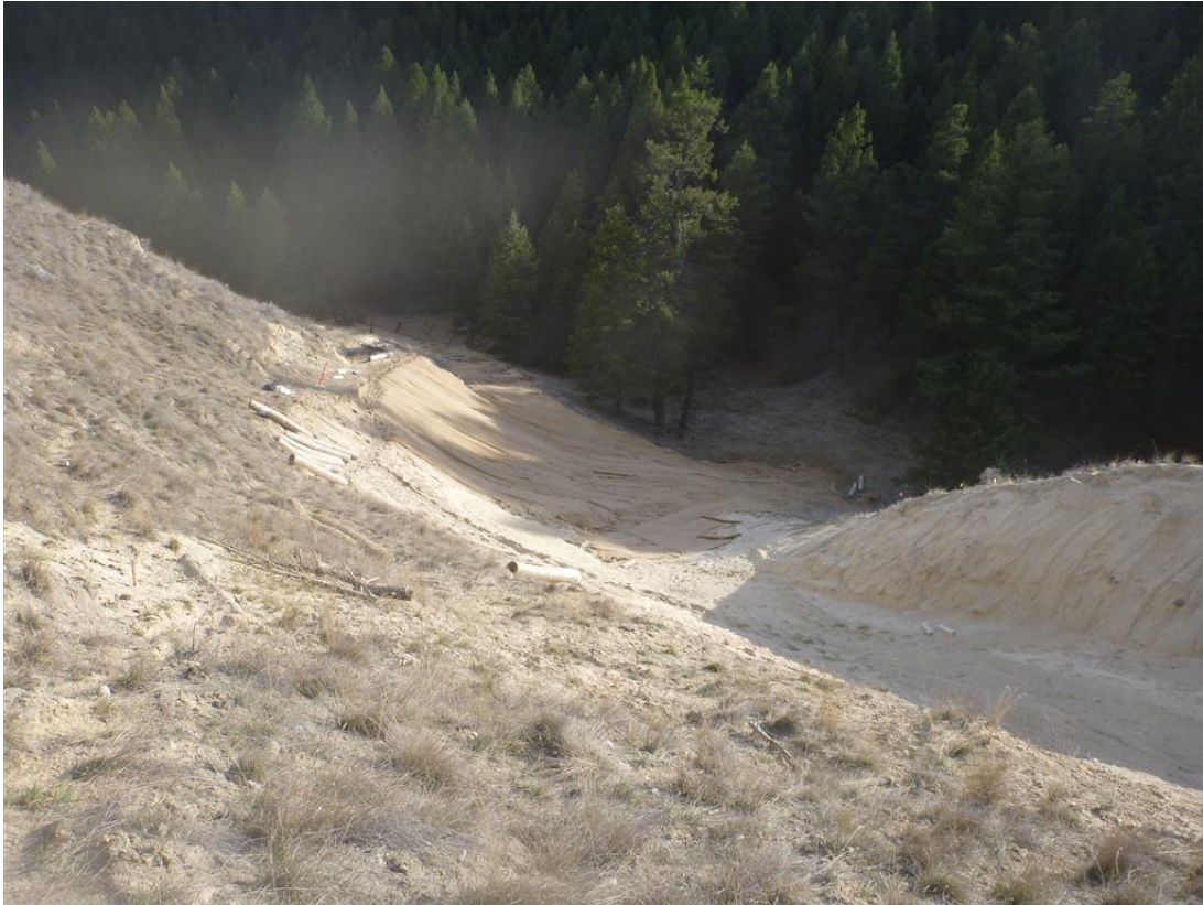
Photo 95: Commencement of erosion control blankets in MDZ.
