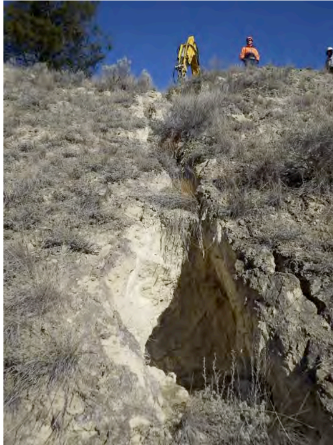
Photo 3: Gully (0.75 m deep) extending downslope from slope crest
