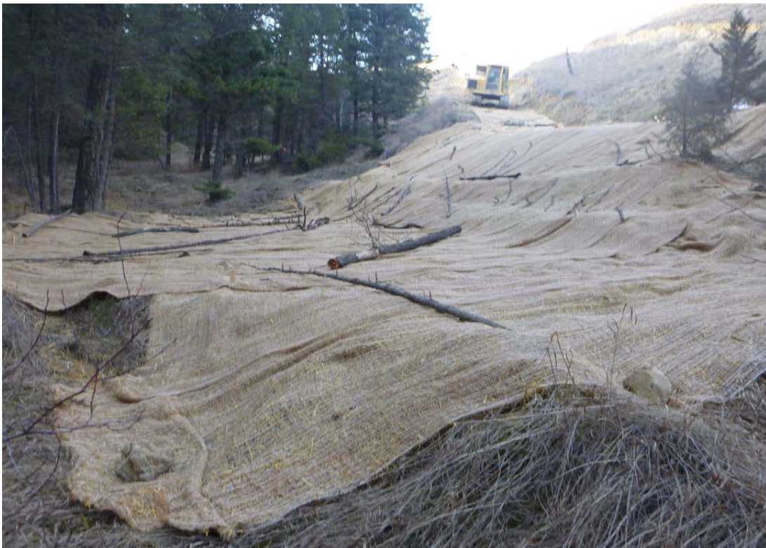
Photo 92: Biodegradable erosion control blanket and woody debris installation and woody debris – AI3.
