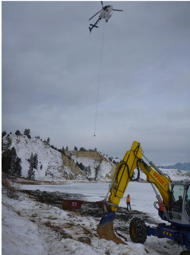
Photo 63: Debris bins and bags flown to stockpile management area by helicopter.
