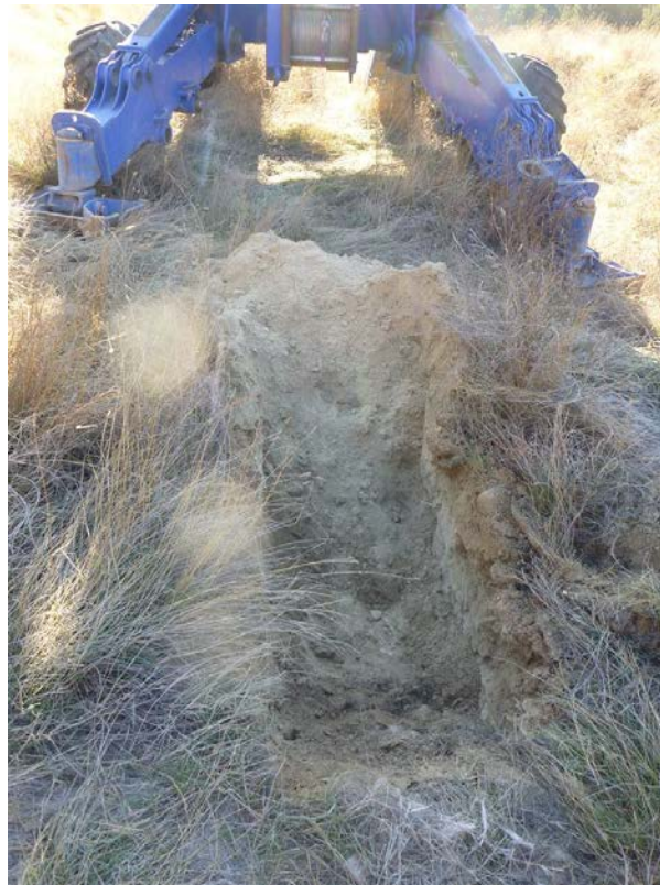
Photo 3: TP1 – First scrape of surface material. Some minor debris observed.
