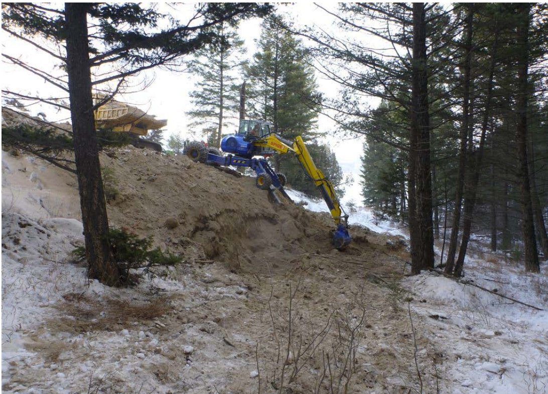
Photo 68: Excavation of A13 by spider hoe.
