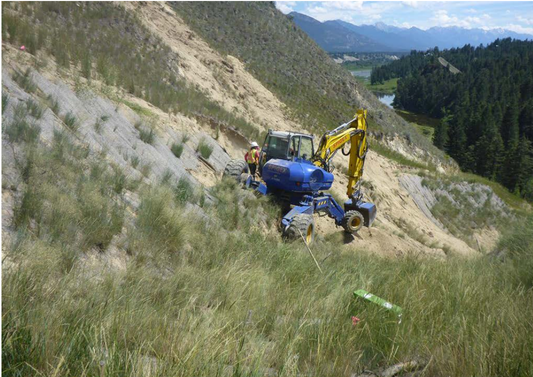
Photo 5: Test pitting with all-terrain excavator (spider hoe) in June 2016.
