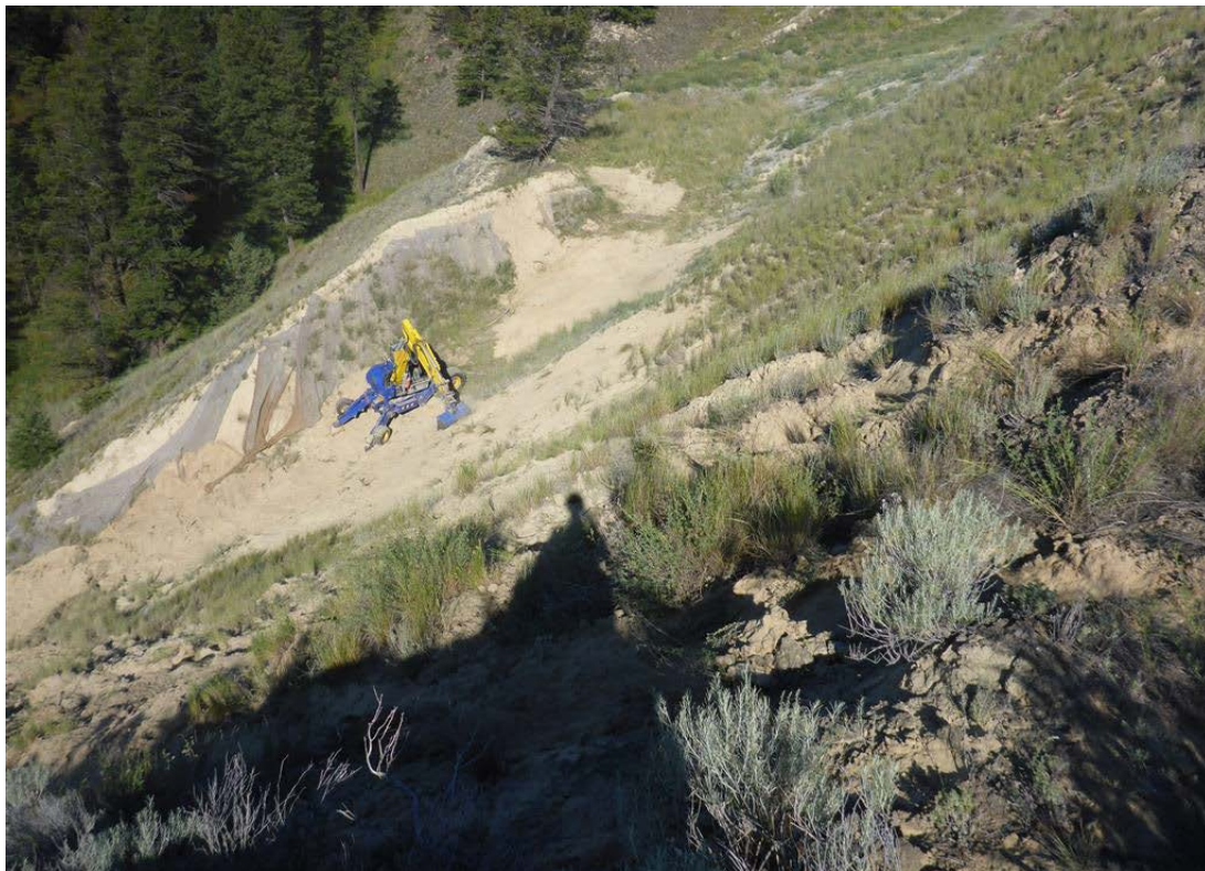
Photo 4: Test pitting in MDZ in June 2016.
