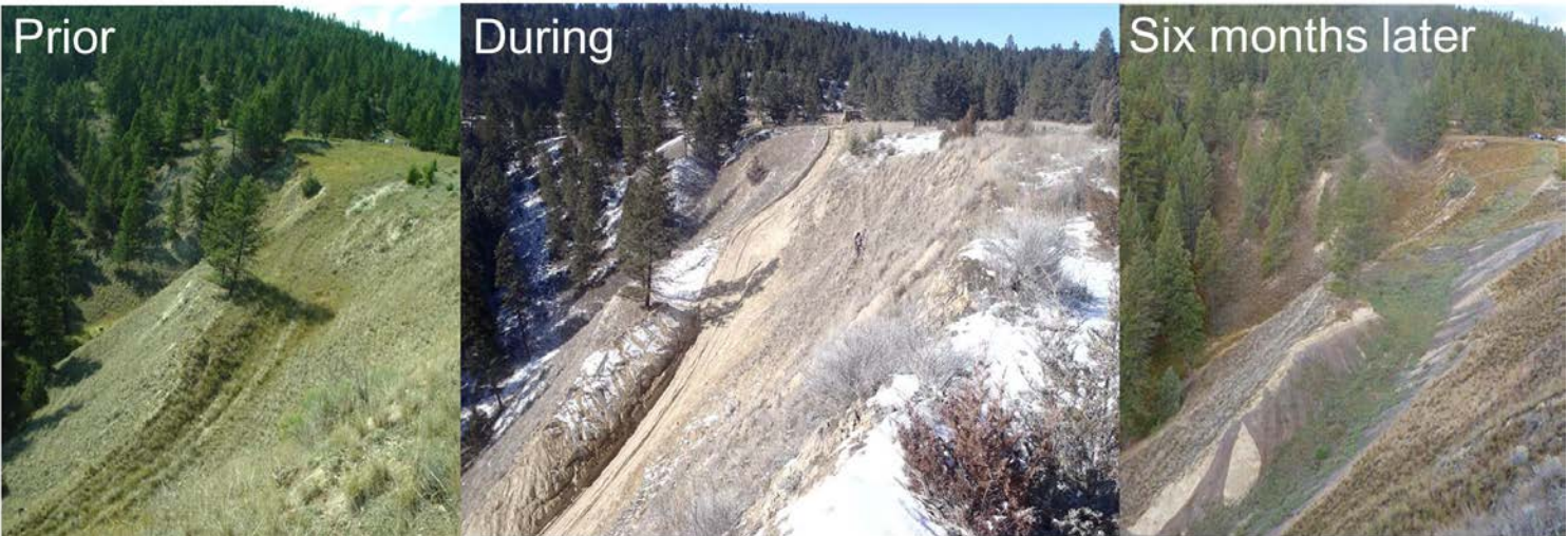
Photo 2: View of MDZ prior to, during and six months following remediation in 2014-2015.
