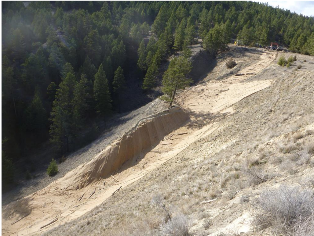
Photo 3: View of extensive erosion control blanket installation in March 2015.
