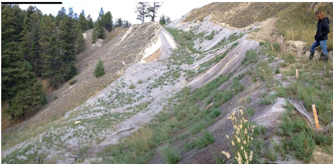
Photo 2: View of the Main Debris Zone to the west from the bottom of the slope. Note panels of fabric on the south side of the slope that have been wind blown (Sept. 21, 2015)
