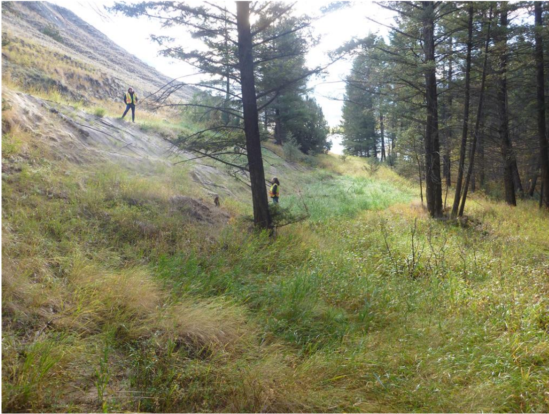
Photo 5: View of gully below remediation work area looking toward marsh.
