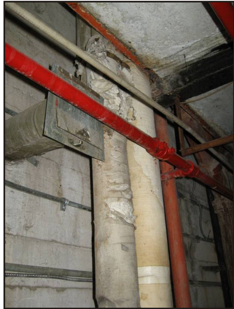
PHOTO 8: AIRCELL PIPE INSULATION (70% CHRYSOTILE) IN POOR CONDITION ROOM 108 (img_2416.jpg)
