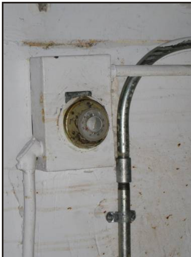
PHOTO 6: MERCURY THERMOSTAT IN ROOM 107 (img_2403.jpg)
