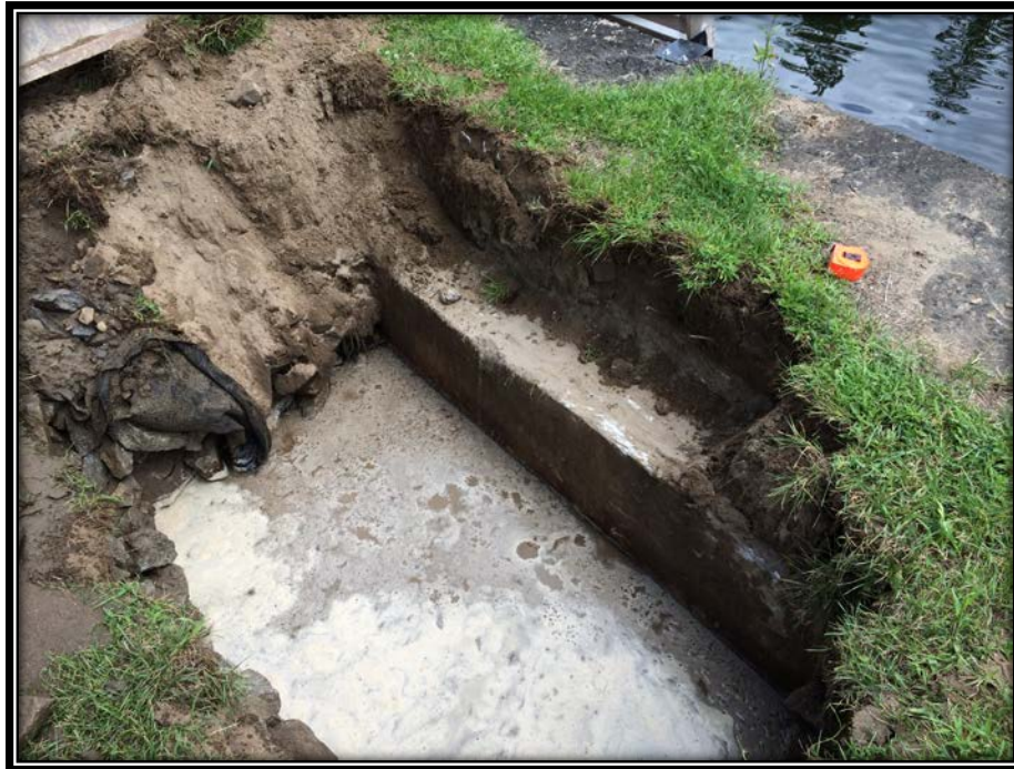
Figure 13 –TP7-N, concrete retaining wall
