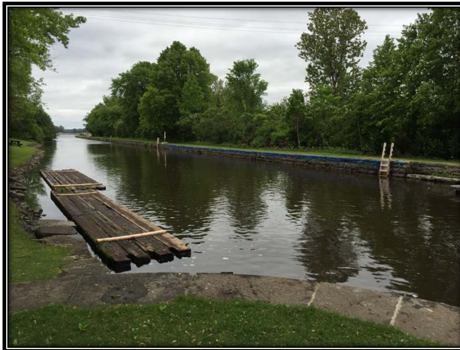
Figure 1 - Nicholson's Earth Dam - upstream side, looking west at canal wall (June 01-2015)
