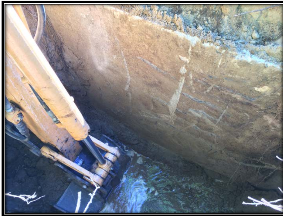
Figure 3 –TP2-N, concrete retaining wall
