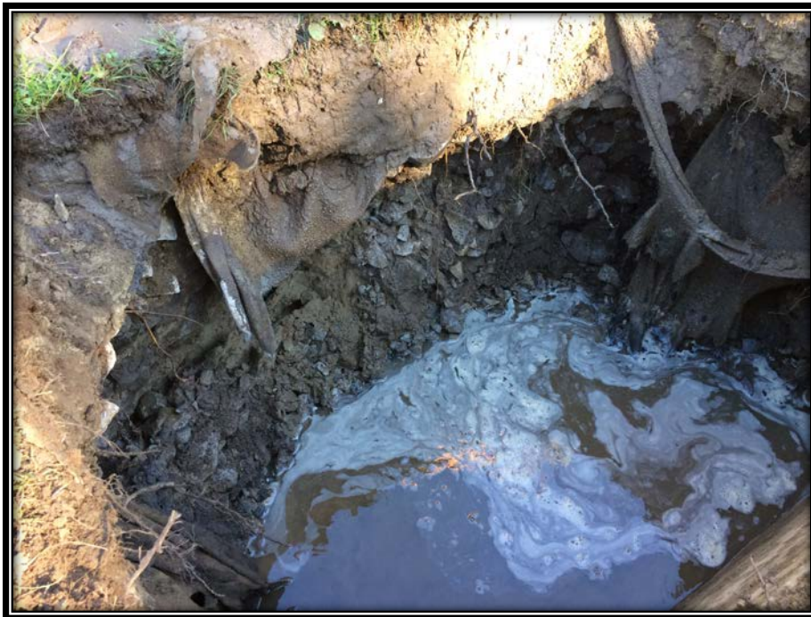
Figure 2 –TP1-N, overburden material – note geotextile fabric on edges of test pit
