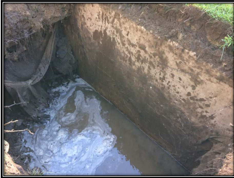
Figure 1 –TP1-N, concrete retaining wall
