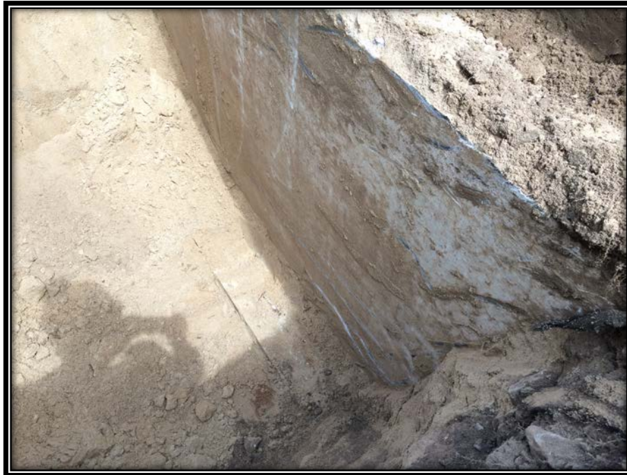
Figure 15 – TP8-N, concrete retaining wall
