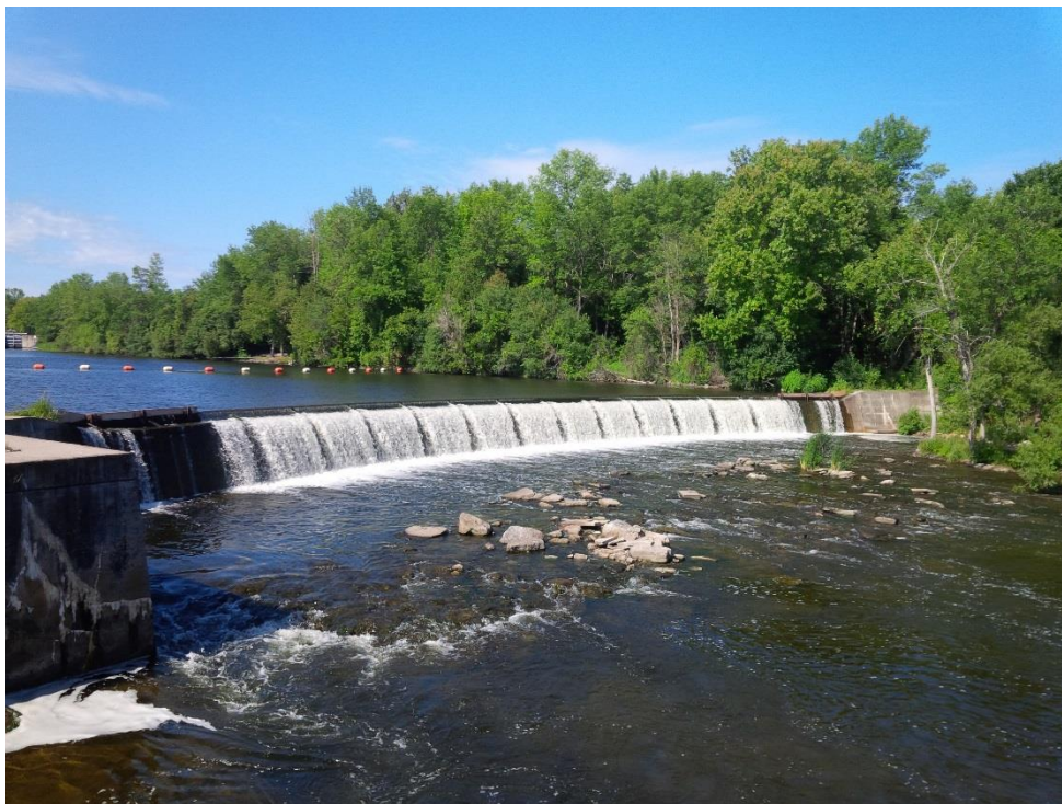
Photo 3. View of spillway dam and western embankment (July 2016).
