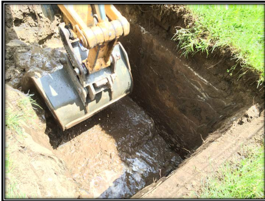
Figure 11 –TP6-N, concrete retaining wall
