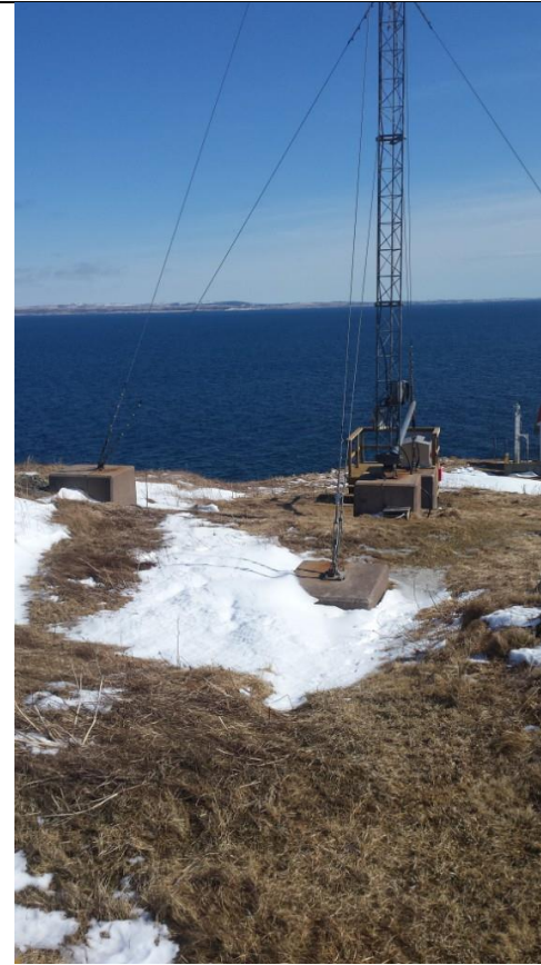
Photo 2: Proposed Location of Turbine 14-01 after decommissioning of existing turbine.
