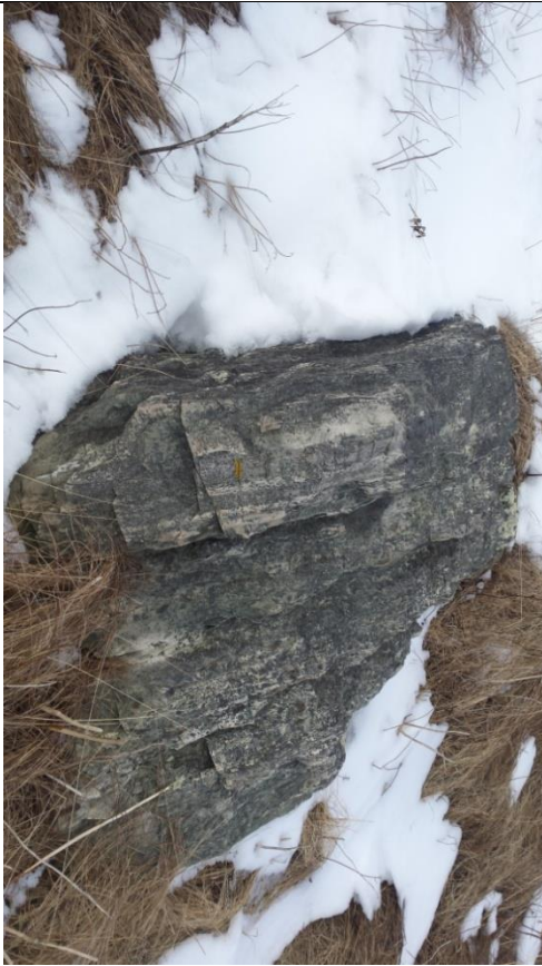
Photo 21: Outcrop G located ~ 30 m NE of approximate location of Turbine 14-04. One dominant joint set striking E-W with near vertical dip.
