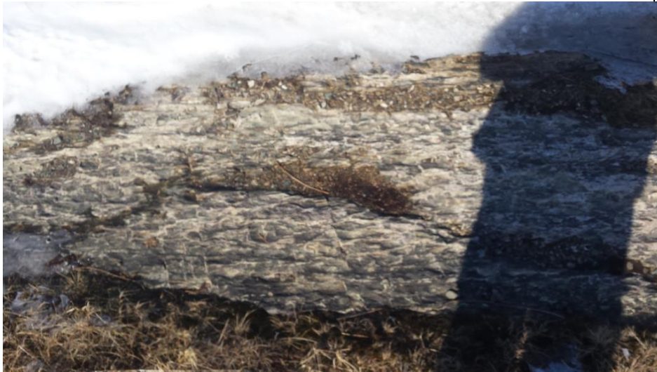
Photo 11: Outcrop D – near approximate location of Turbine 14-02. Note close spacing of joints / cleavage planes with some surface fracturing.
