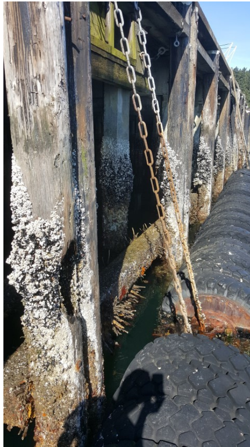
Photo 1: Rubbing pile missing, major section loss of fender pile
