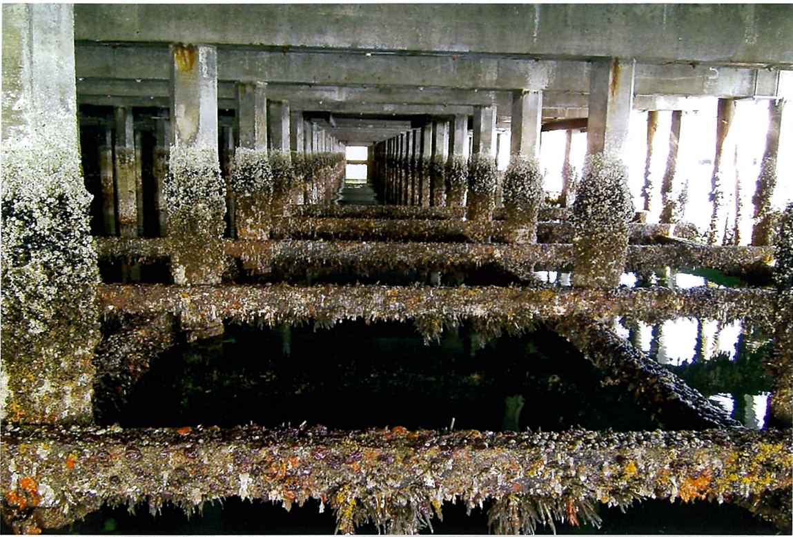
VIEW OF EXPOSED CROSS BRACING LOOKING EAST ON NORTH BERTH
