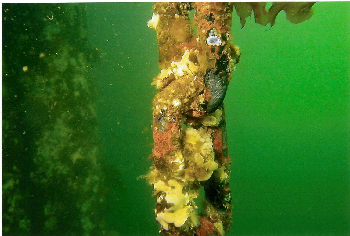
GENERAL CONDITION OF MOORING CHAINS AND COUNTER WEIGHT FOR CAMEL FENDERS
