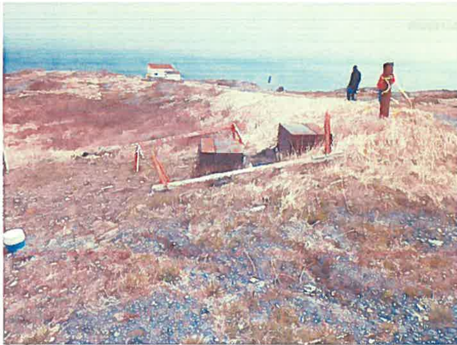
Figure 1 Transformers to be Decommissioned and Replaced
