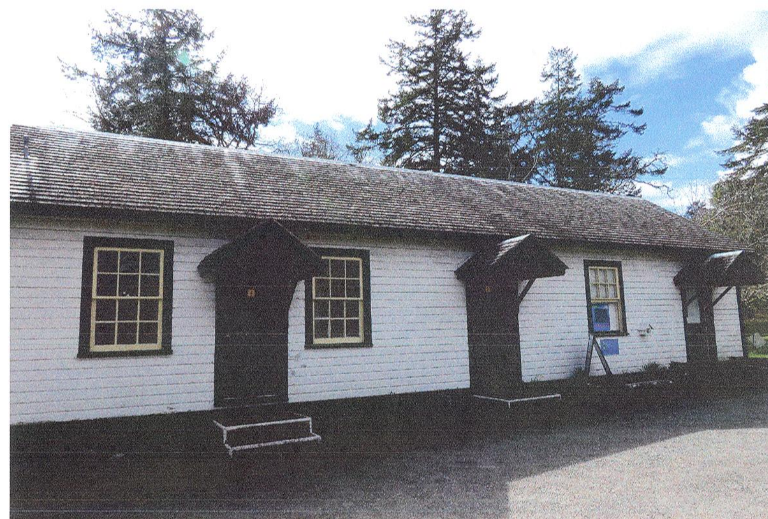
BUILDING 5: WW2 HUT (WASHROOM BUILDING) VIEW FROM NORTH
