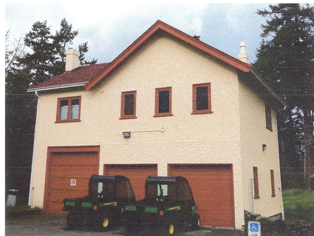
BUILDING 2: CARRIAGE HOUSE VIEW FROM SOUTH
