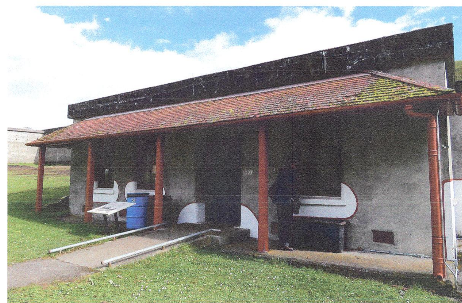
BUILDING 6: CANTEEN VERANDA VIEW FROM NORTH
