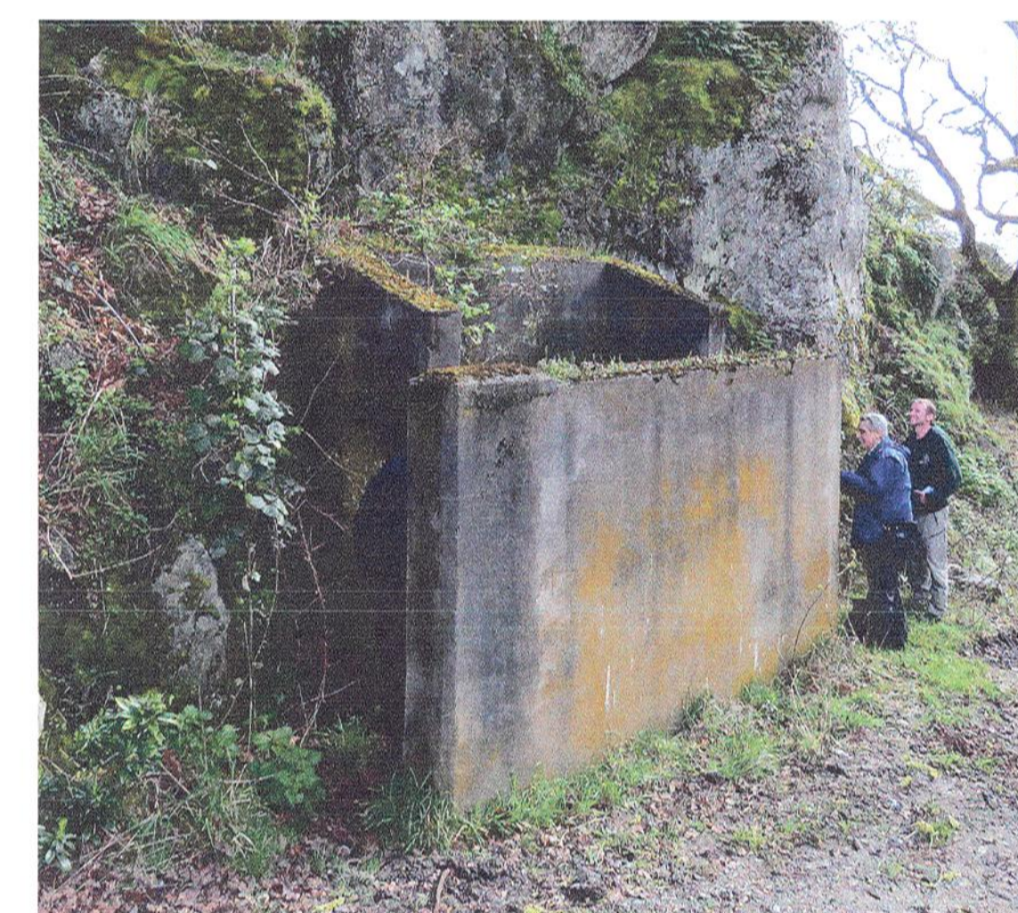
BUILDING 9: LATRINE BUILDING VIEW FROM NORTH
