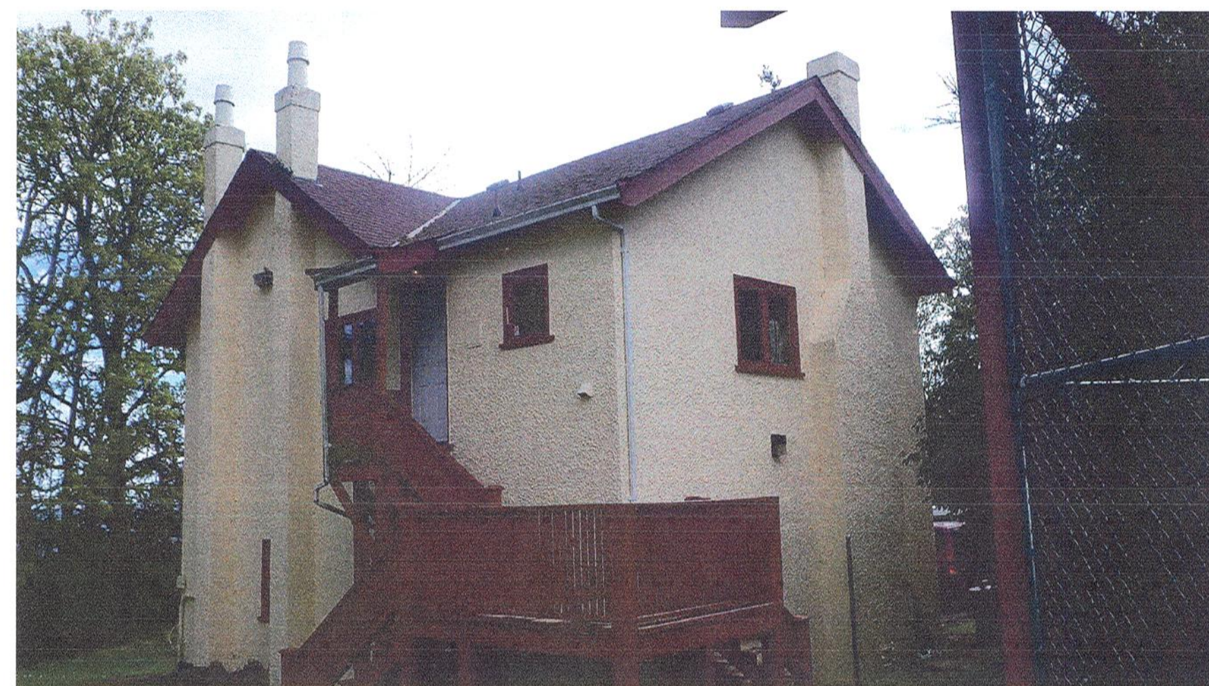
BUILDING 2: CARRIAGE HOUSE VIEW FROM NORTH
