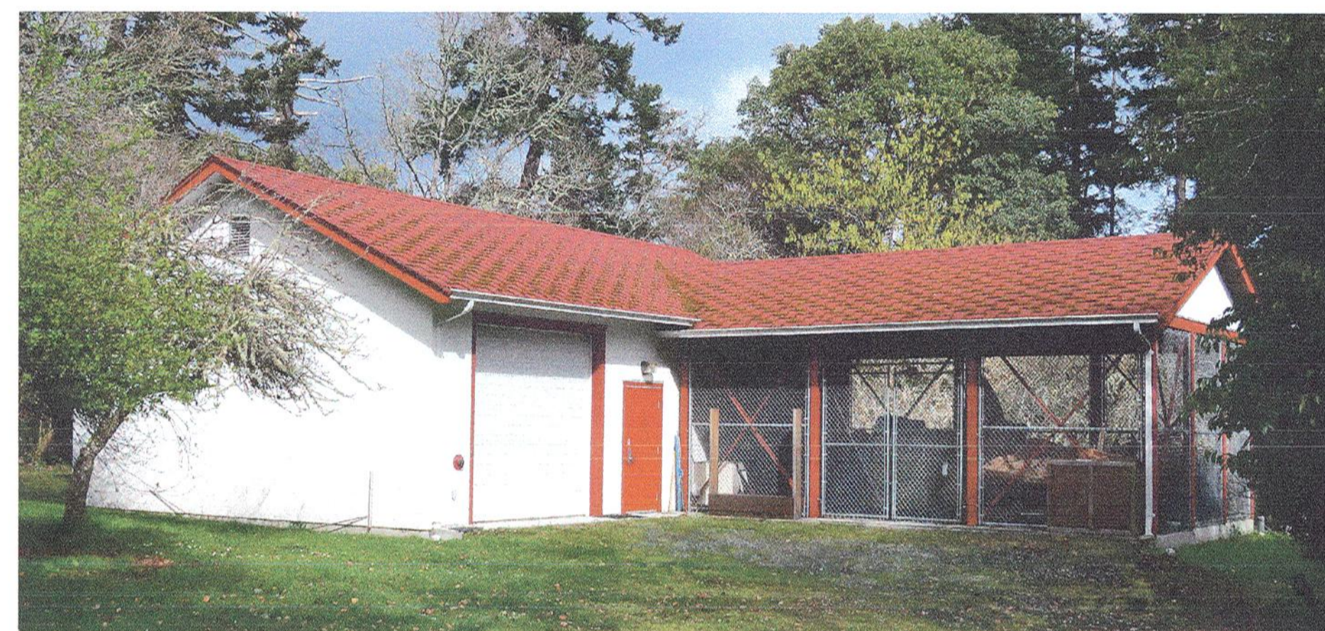
BUILDING 3: COLLECTIONS BUILDING VIEW FROM SOUTH
