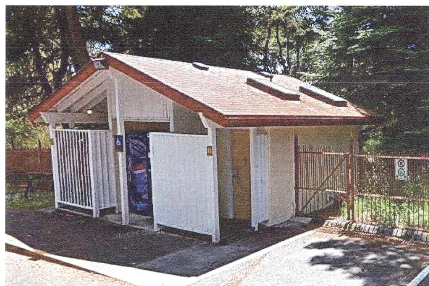
BUILDING 10: WASHROOM BUILDING VIEW FROM NORTH
