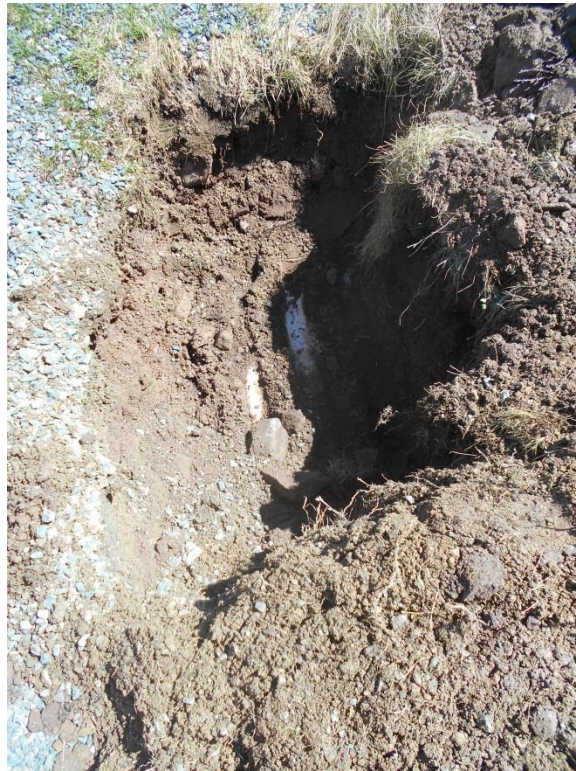
Test Pit TP-05
