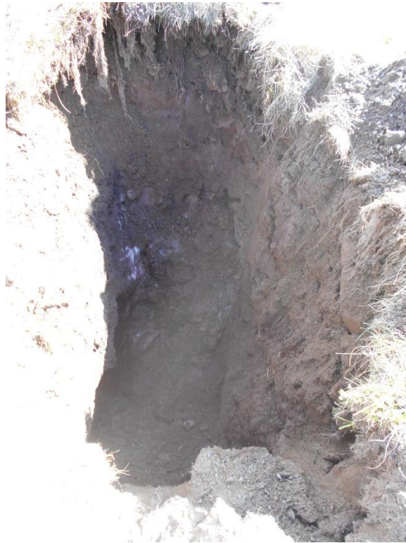
Test Pit TP-01
