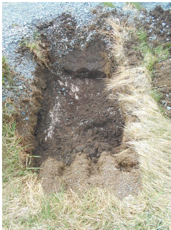
Test Pit TP-08
