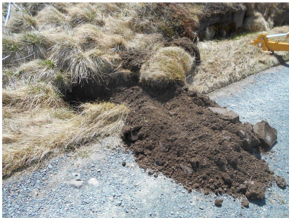
Test Pit TP-10 Spoil Pile
