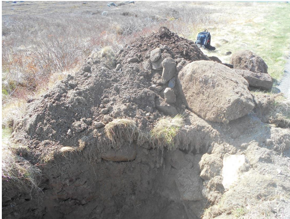
Test Pit TP-01 Spoil Pile
