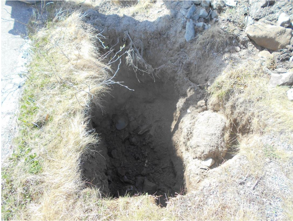
Test Pit TP-03
