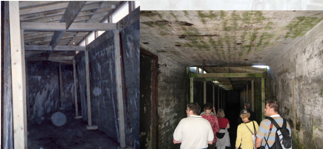
Figure 12. WWII bunker. Corridors that lead to the ammunition storage rooms.
