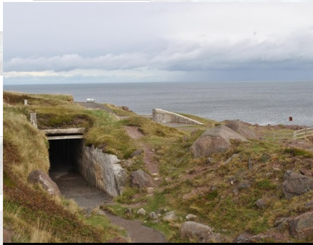
Figure 6. Cape Spear WWII bunker.
