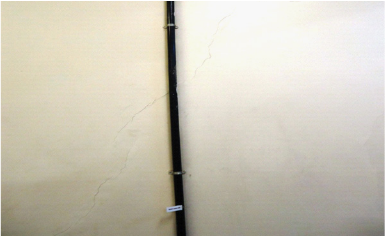
S-5: Vertical Crack on Slab soffit in sub-basement Electrical Room
