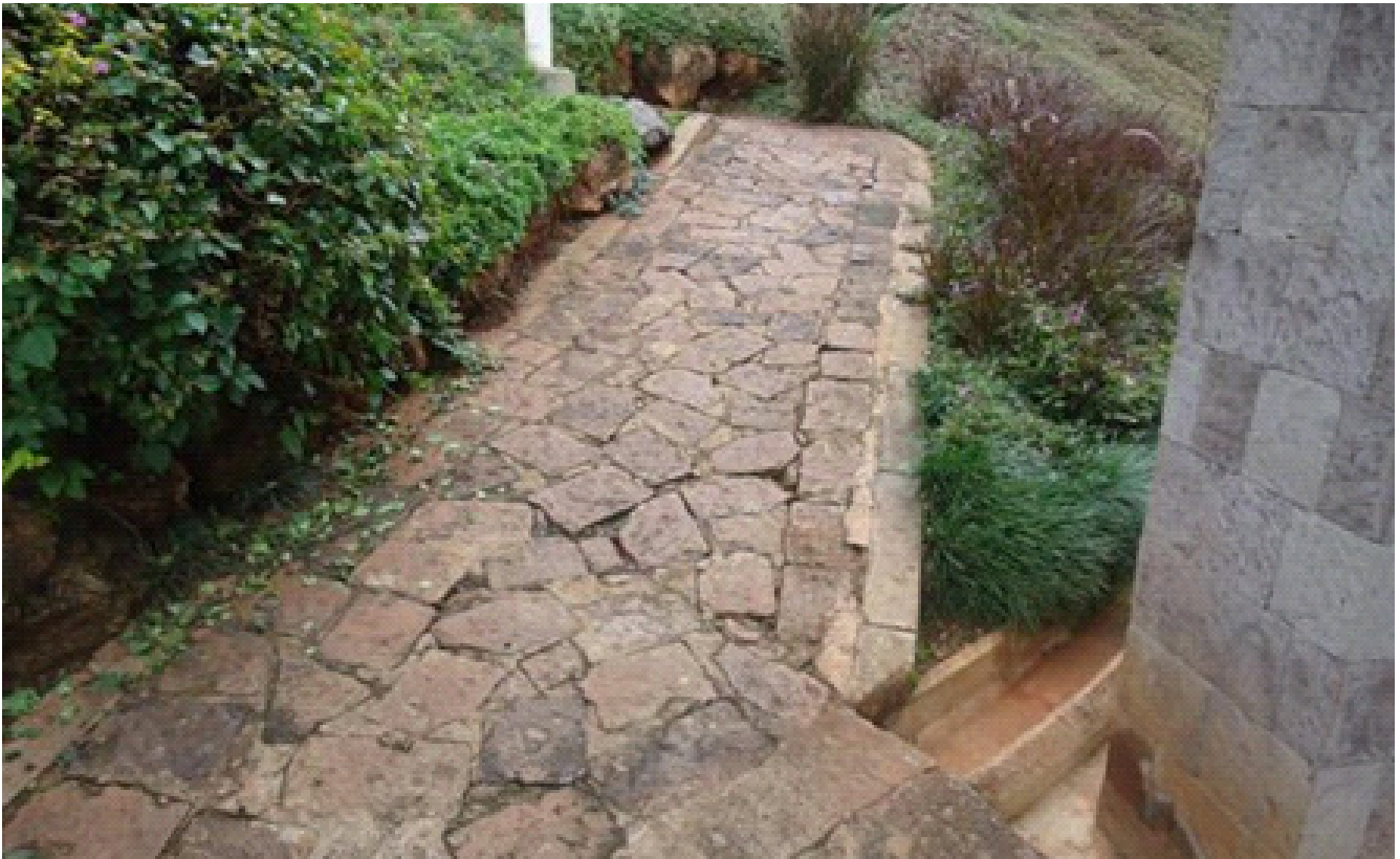
BG-1: Access to the public area
