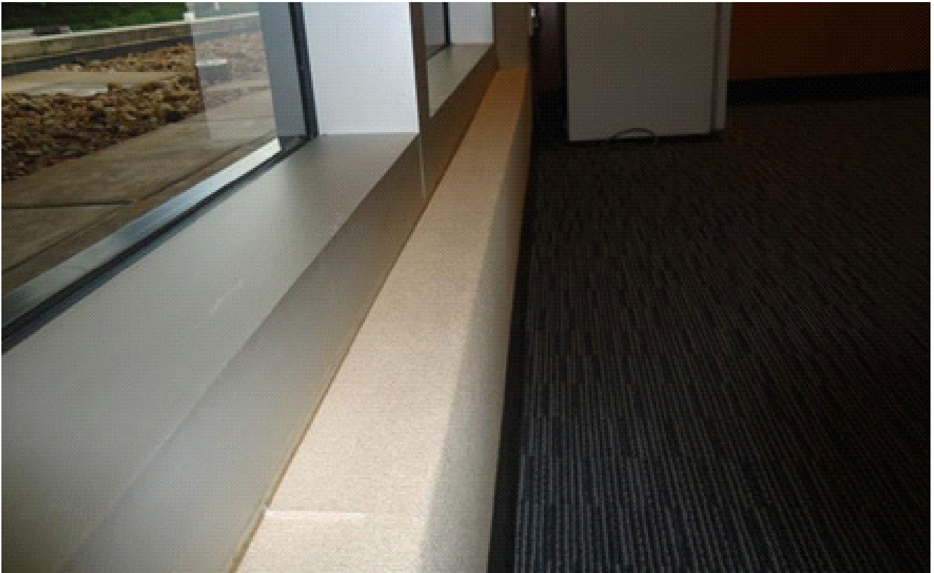
BE-7: Window Frame
