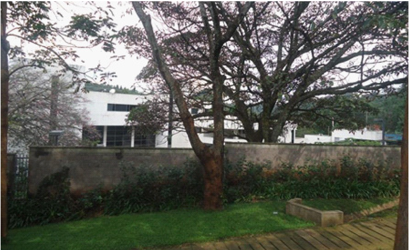
BG-2: Aluminum Glass Curtain Wall from Limuru Road
