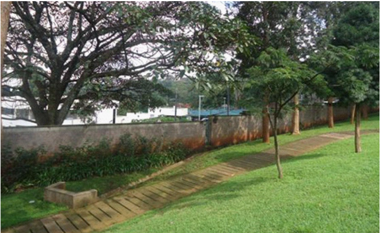
BG-4: Boundary wall along Limuru road
