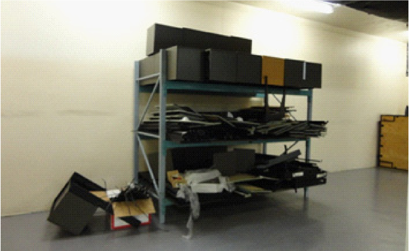
MS-5: Storage in AHU Room
