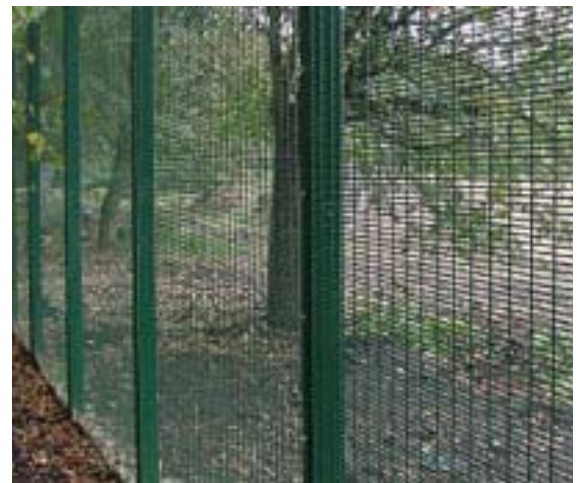
Figure 4.2.20: Weld mesh fence
