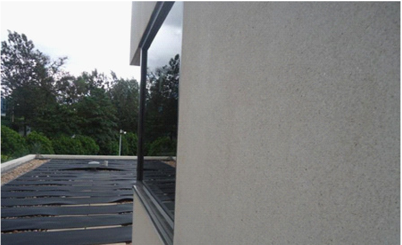
BE-8: Window glazing from outside
