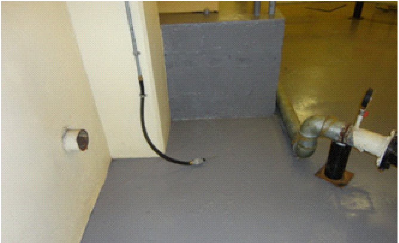
MS-14: Tamper switch at old valve position
