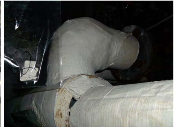
Photo 63: View of pipe elbow parging sample AS-62.
