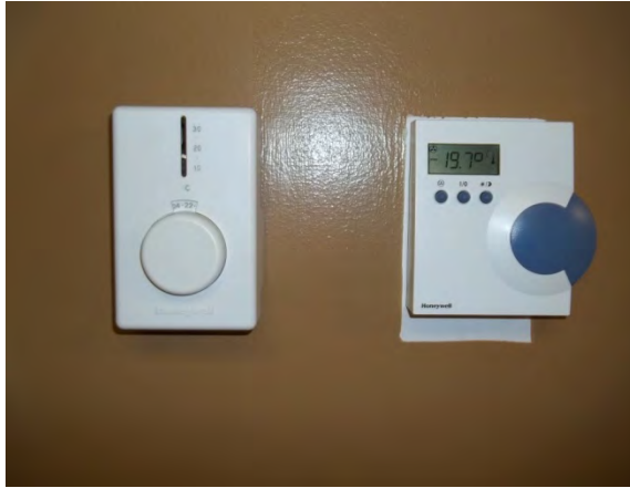
Photo 122: View of white Honeywell rectangular (left) and electric square (right) thermostats.
