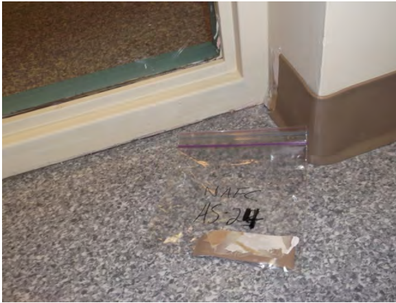
Photo 25: View of baseboard and mastic sample AS-24.
