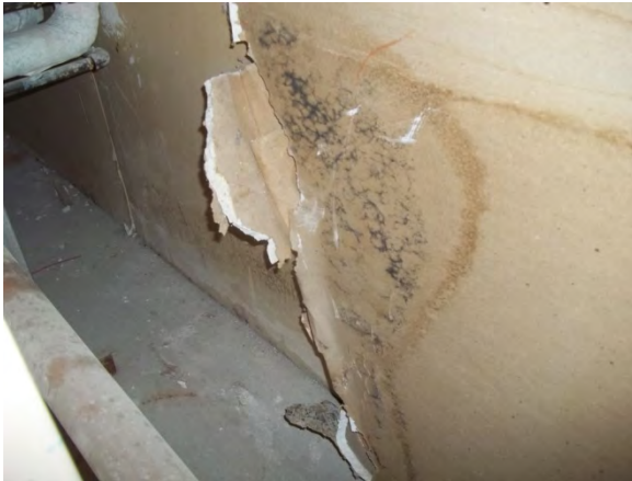
Photo 91: View of water staining and suspected visible mould growth on drywall in N20-125.
