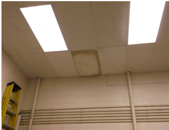
Photo 89: View of acoustic ceiling tile water stain in M19-101.
