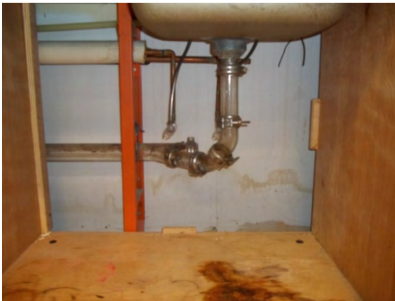
Photo 88: View of water staining on drywall under a sink in N20-118.
