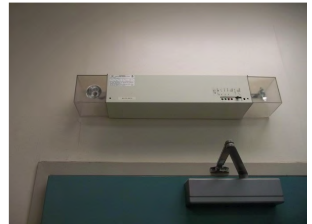
Photo 132: View of emergency light fixture.
