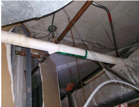
Photo 92: View of water staining and suspected visible mould growth above ceiling tiles in N20-101.
