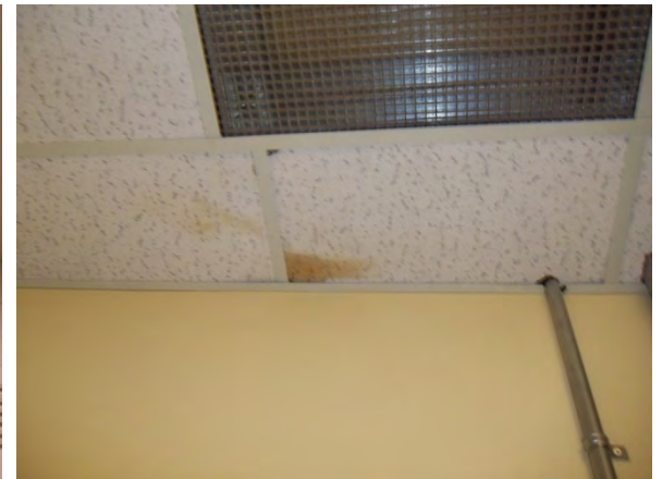
Photo 90: View of acoustic ceiling tile water stain in N20-108A.
