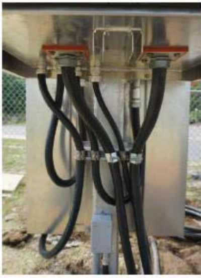
View of Cable entry to instrument box
