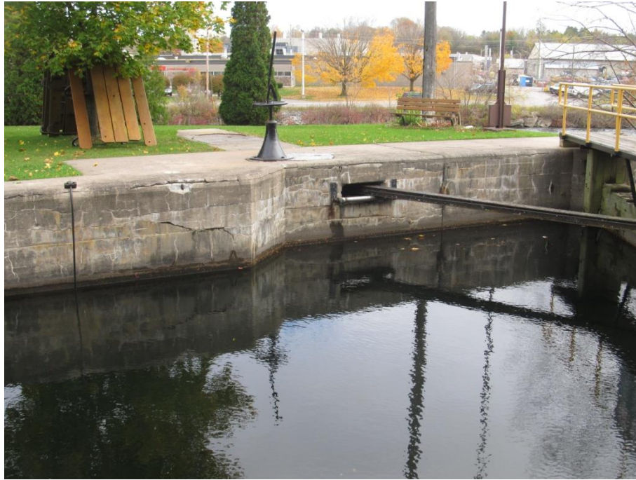
(P7) Lock 26 - SE Lock Gate Control Mechanism and Roller Bar
