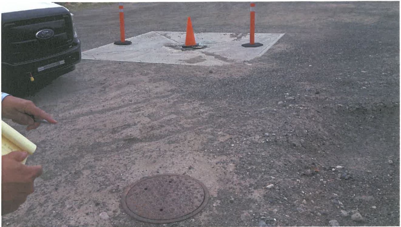
Photo 5: View of the manhole to the sanitary utility line within the south section of the planned 2016 excavation footprint.
