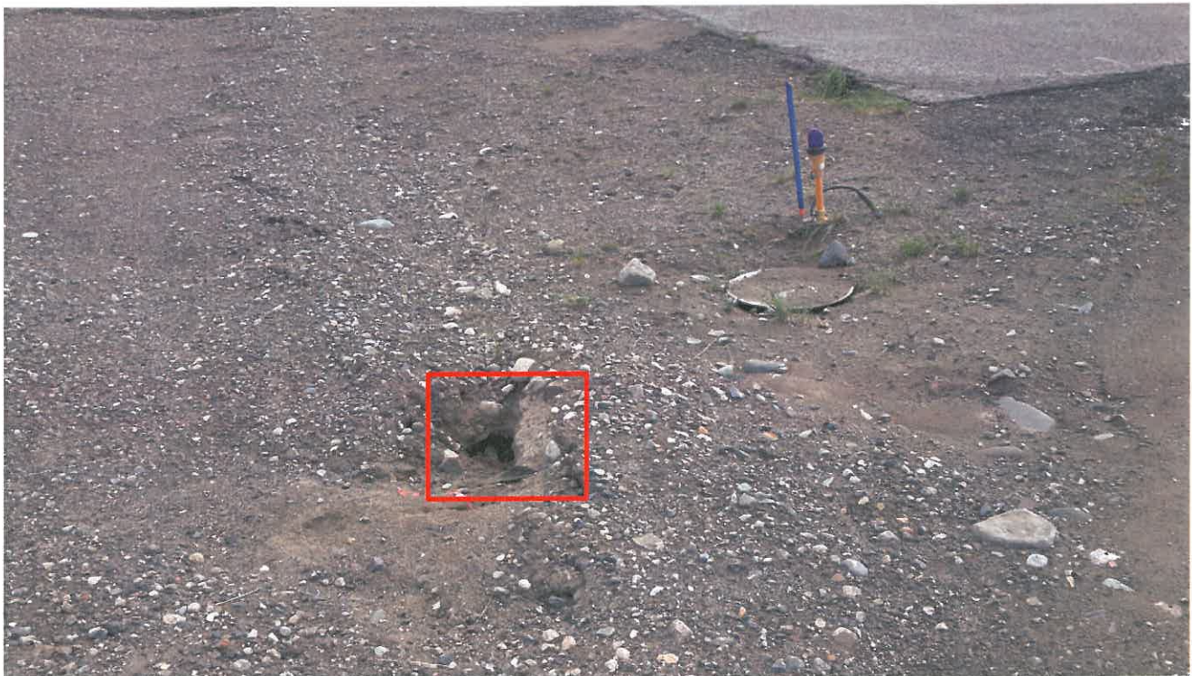
Photo 4: View of another of the subsidence areas within the 2015 remedial excavation footprint, which requires reparation during Phase I of the work program. Of note is the piping shown in the red box.
