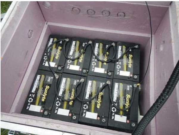
DC Kit Battery Box interior
