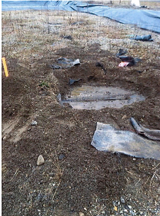
Photograph 13: Detailed view of LTF cell liner perforation.
